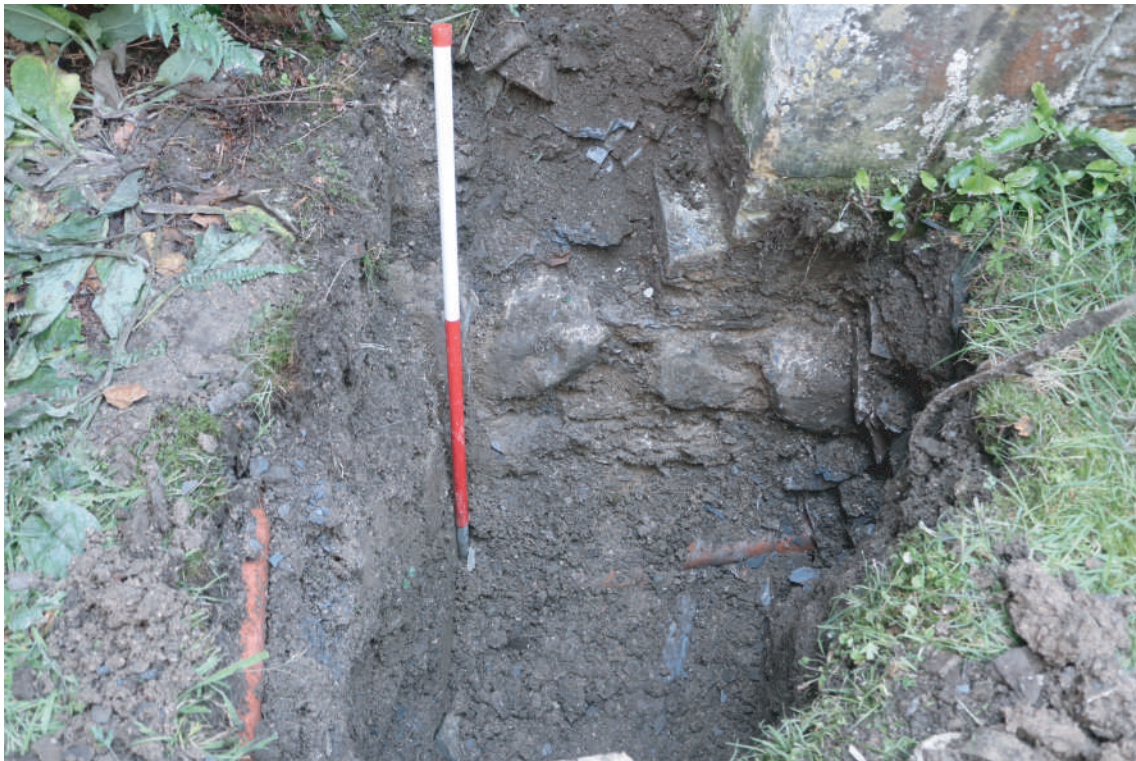
Plate 33. St. David's Church, Blaenporth - Completed Trench for Lightning Conductor Plate 3 on west side of Vestry. Note foundation for earlier church becoming exposed and 19th Century clay drainage pipe at base of trench.. Looking S.
