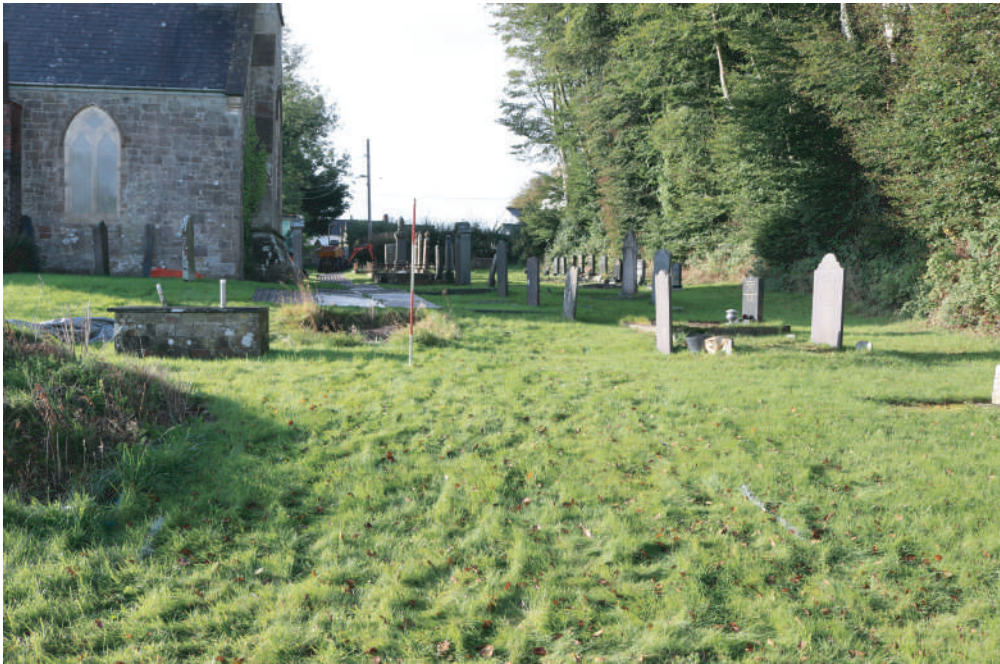
Plate 01. St. David's Church, Blaenporth - View of area of proposed septic tank. Looking south.
