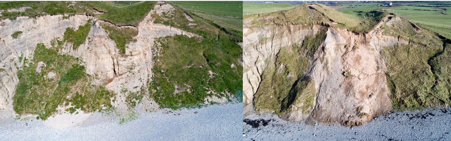
These UAV images of Dinas Dinlle hillfort in Gwynedd show the cliff-face before (June 2018) and after (February 2019) collapse revealing the sand filled inner ditch of the fort. After periods of prolonged rain the ground becomes saturated, which causes water to emerge from the cliff-face at the interface between the underlying soft and hard sediments. The emerging water exacerbates gravitational slumping and the degradation of the softer sediments.
