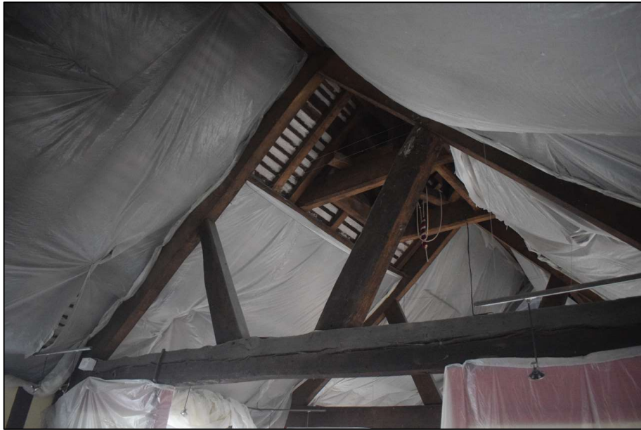
Fig. 13 View north of Roof Truss 2 Photo CPAT 5096-027
