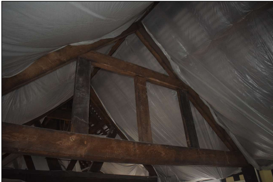
Fig. 14 View south of Roof Truss 1 Photo CPAT 5096-026
