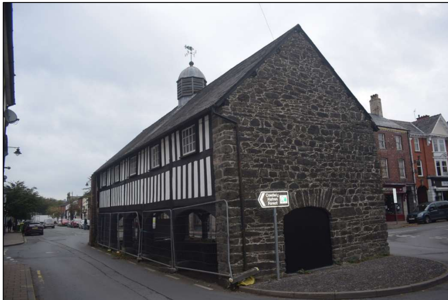
Fig. 2 South and west elevation of the hall looking north along Long Bridge Street. Photo CPAT 5096-002
