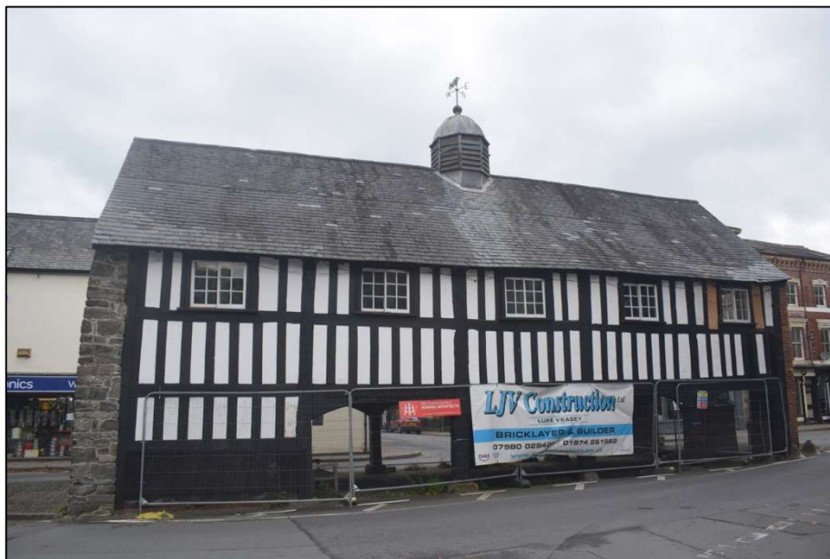
Fig. 6 Hall viewed from the east Photo CPAT 5096-004
