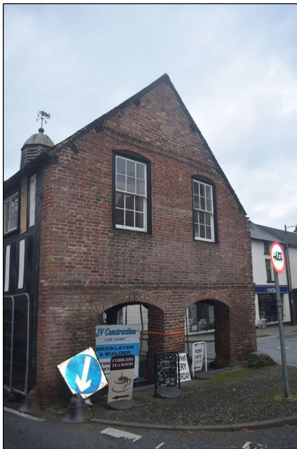
Fig. 4 North elevation of the hall viewed from the north Photo CPAT 5096-006
