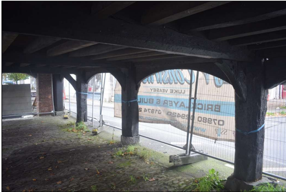
Fig. 7 View north-east across the covered market. Photo CPAT 5096-014
