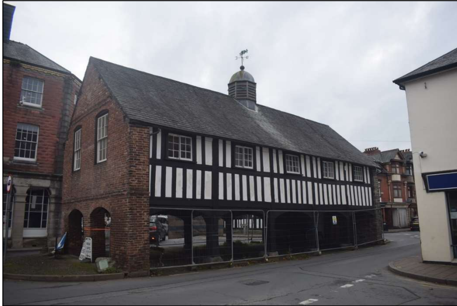
Fig. 3 North and west elevations of the hall viewed from the west. Photo CPAT 5096-001
