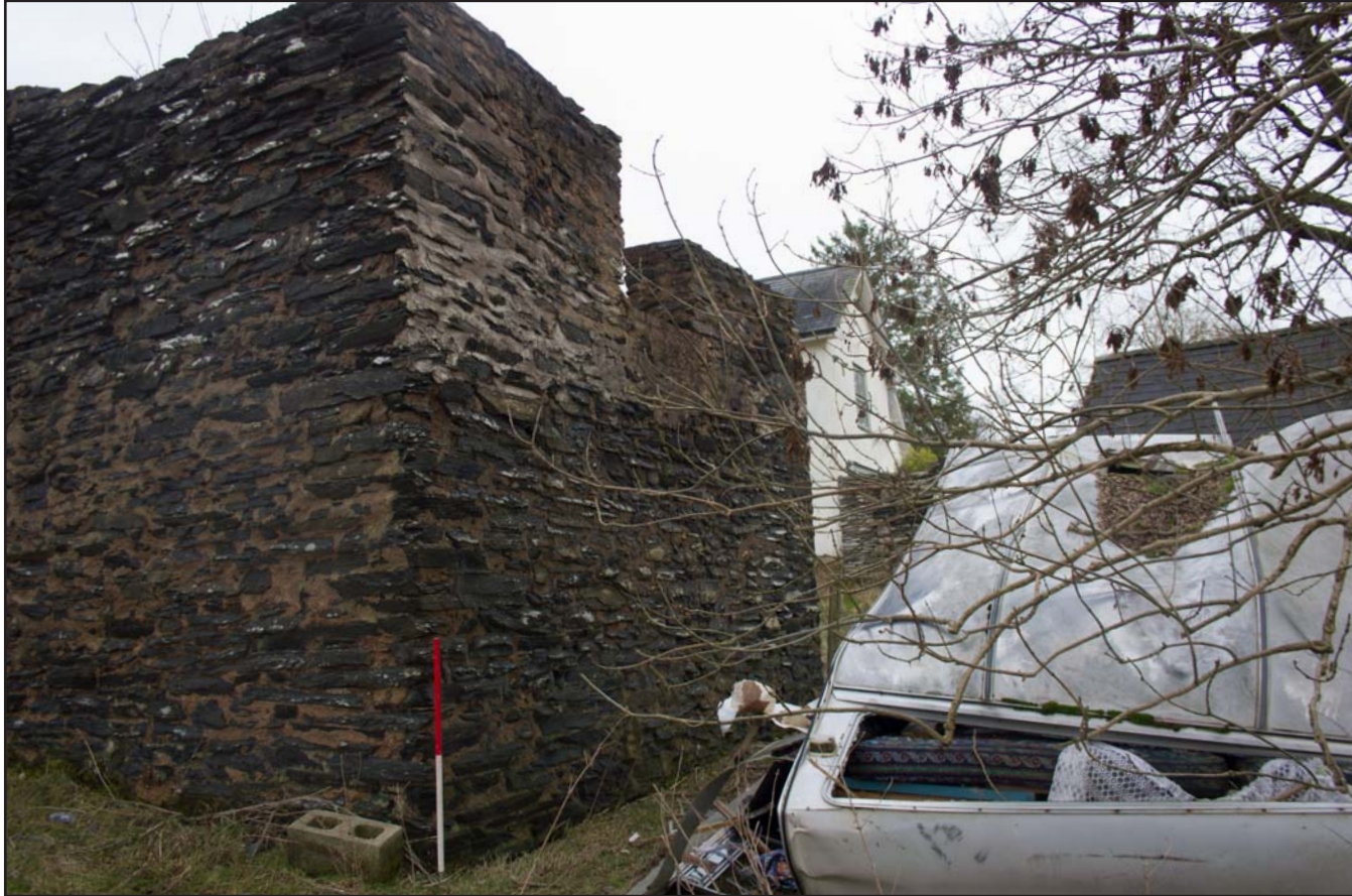
Plate 08: South facing external elevation, from the southwest. Scale 1.0m.
