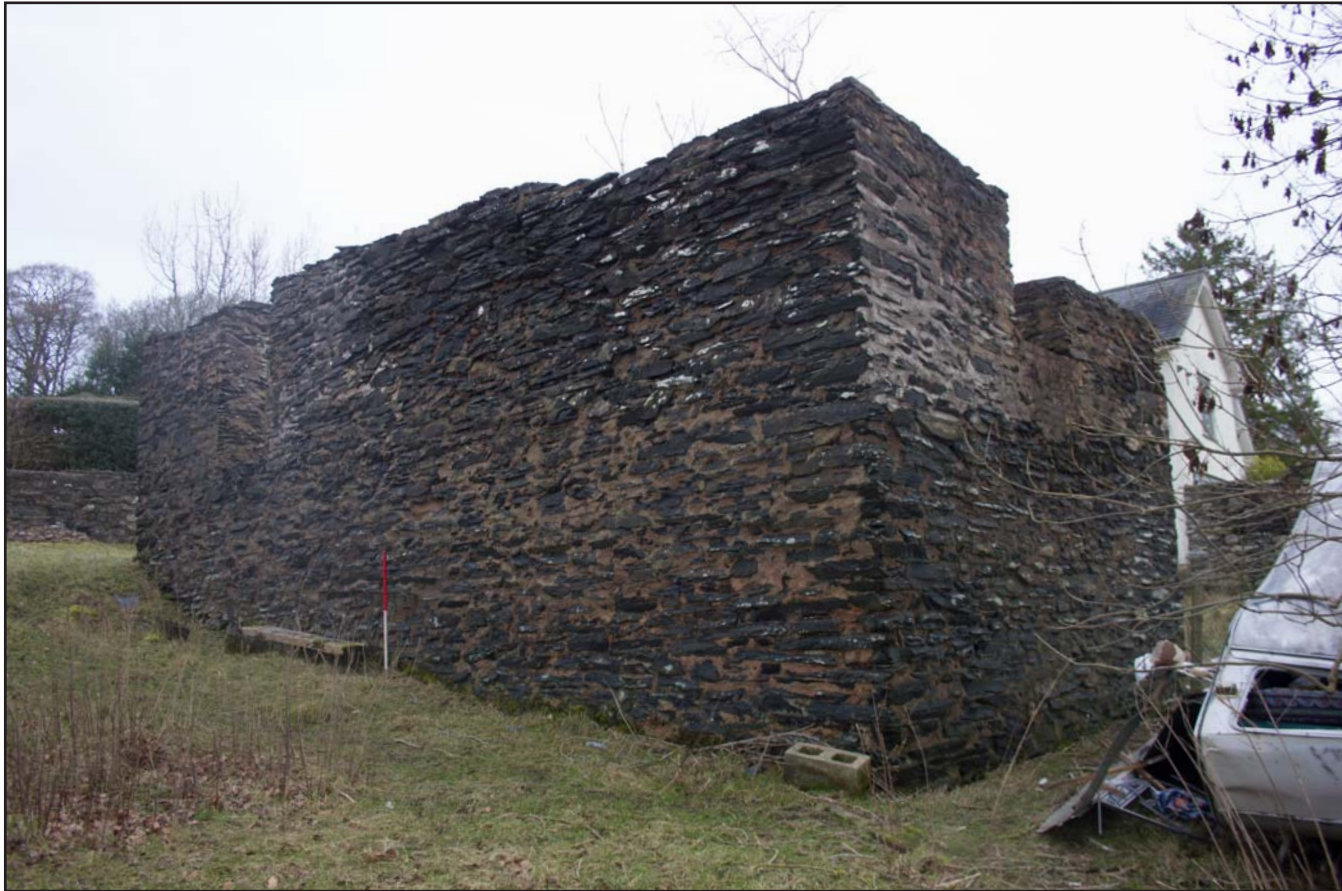
Plate 07: West and south facing external elevations, from the southwest. Scale 1.0m.
