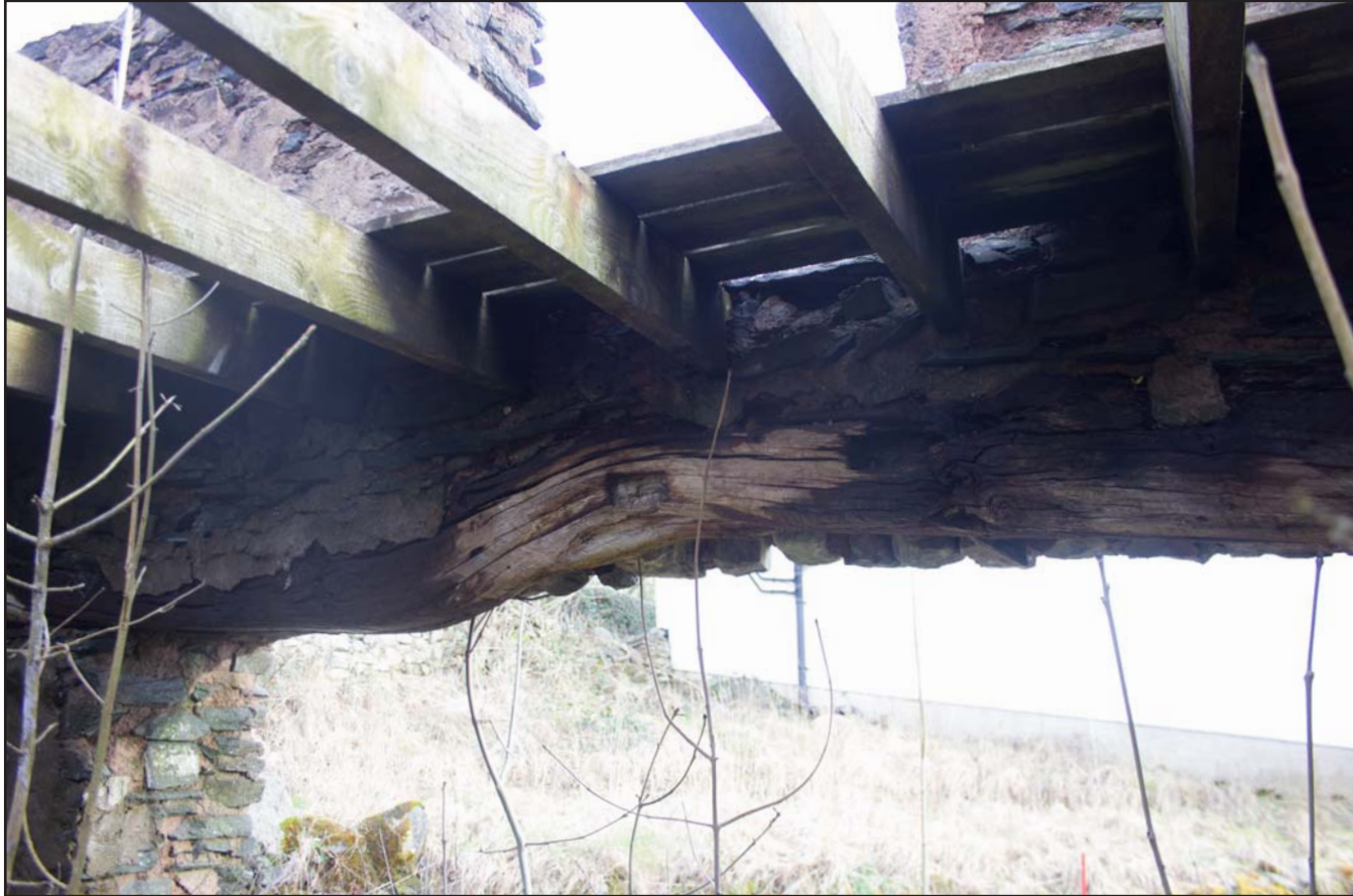
Plate 19: Room 2 showing hand hewn wooden lintel, from the southwest.
