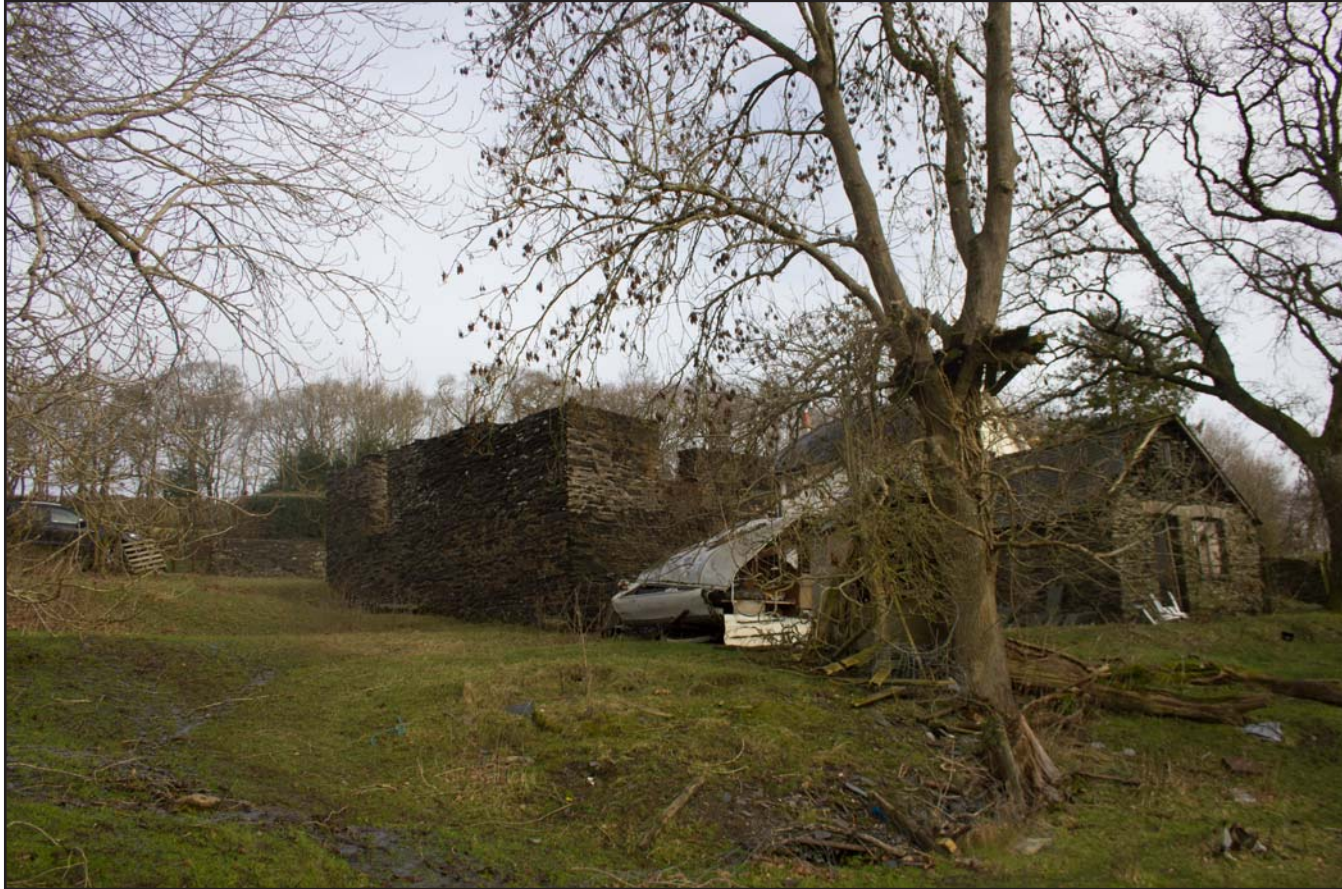
Plate 02: Context shot of outbuilding, from the southwest.
