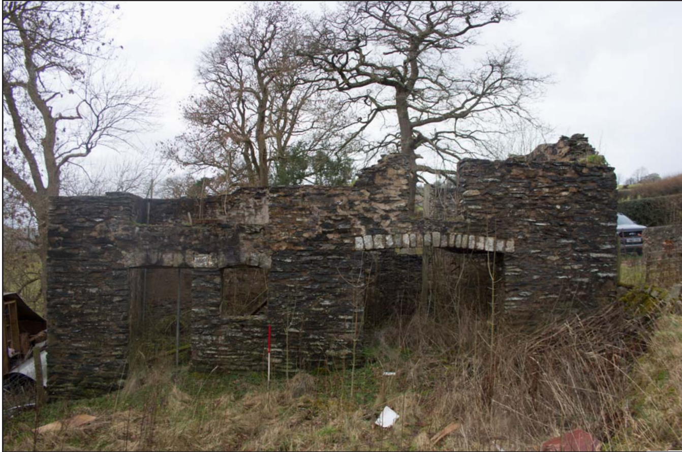
Plate 10: East facing external elevation, from the east. Scale 1.0m.
