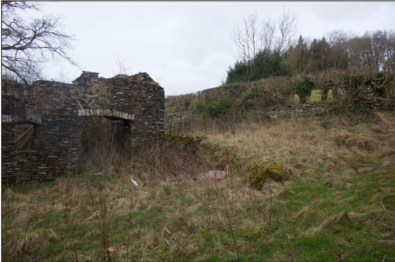
Plate 14: Former access trackway to eastern elevation, from the southeast. Scale 1.0m.
