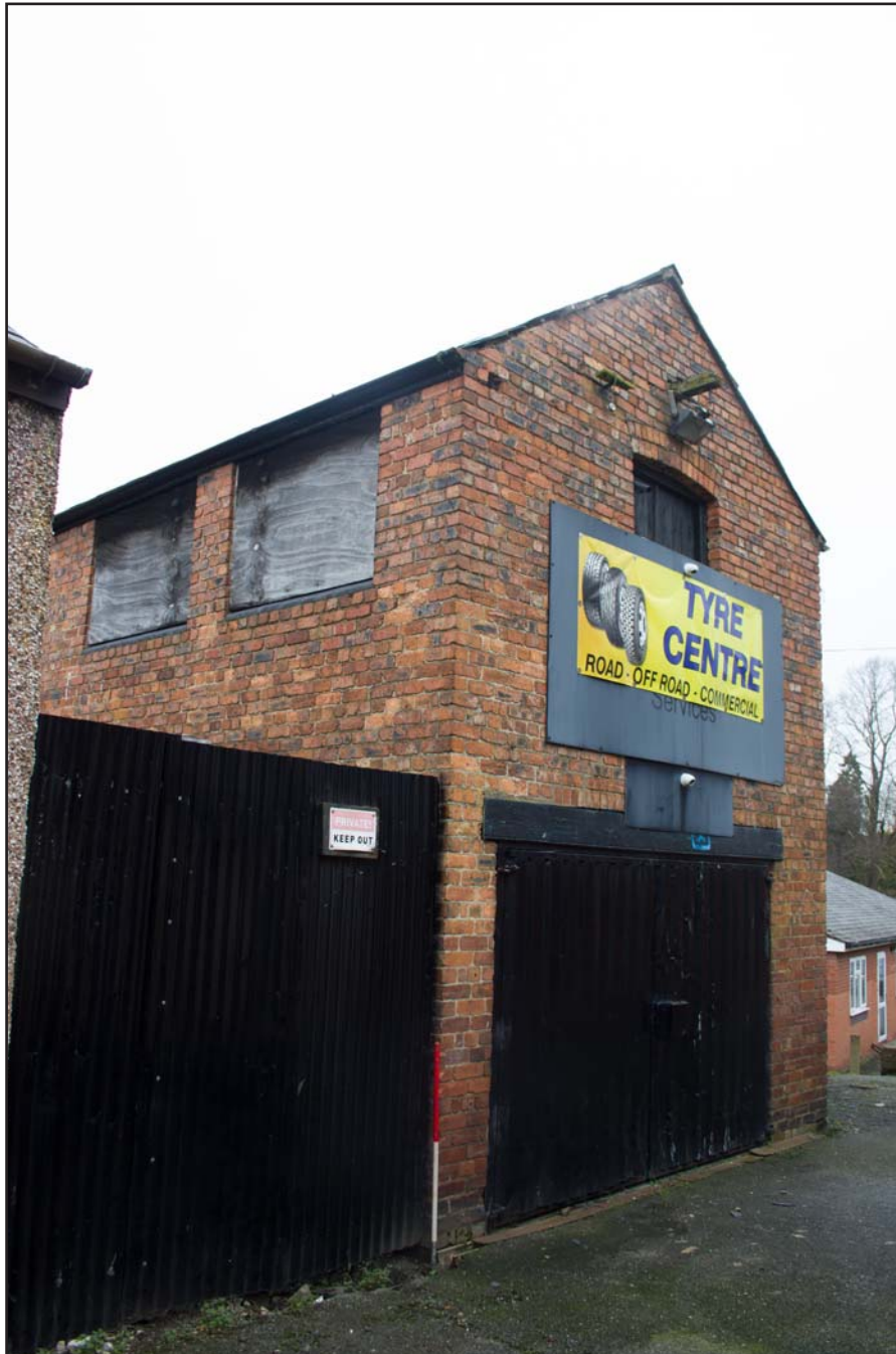
Plate 08: Southwest and southeast facing external elevations, from the south. Scale 1.0m.
