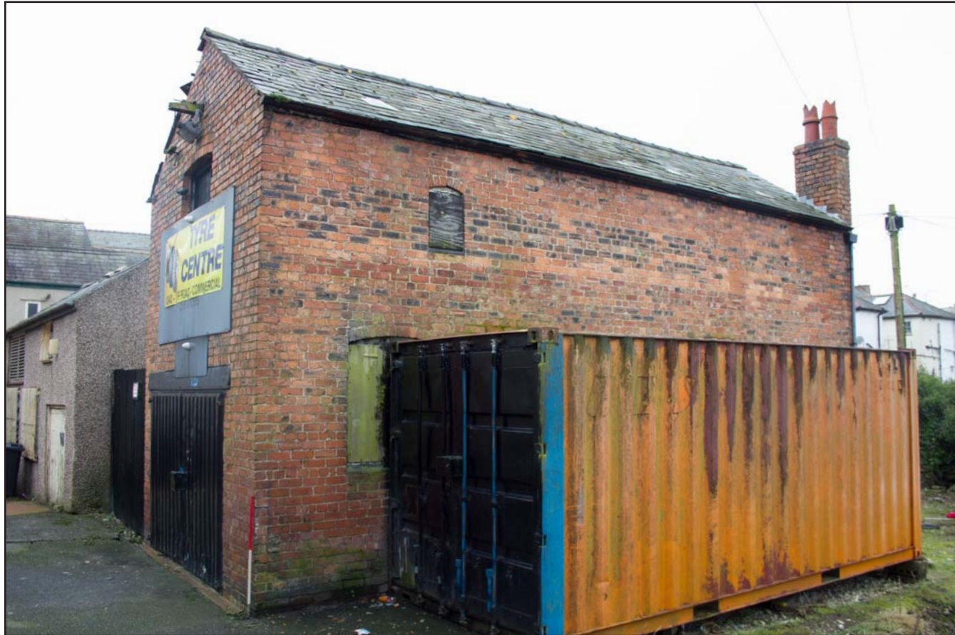
Plate 03: Southeast and northeast external elevations, from the east. Scale 1.0m.
