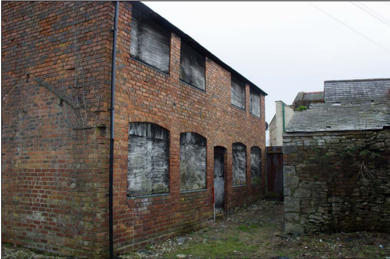
Plate 07: Southwest external elevation, from the west. Scale 1.0m.
