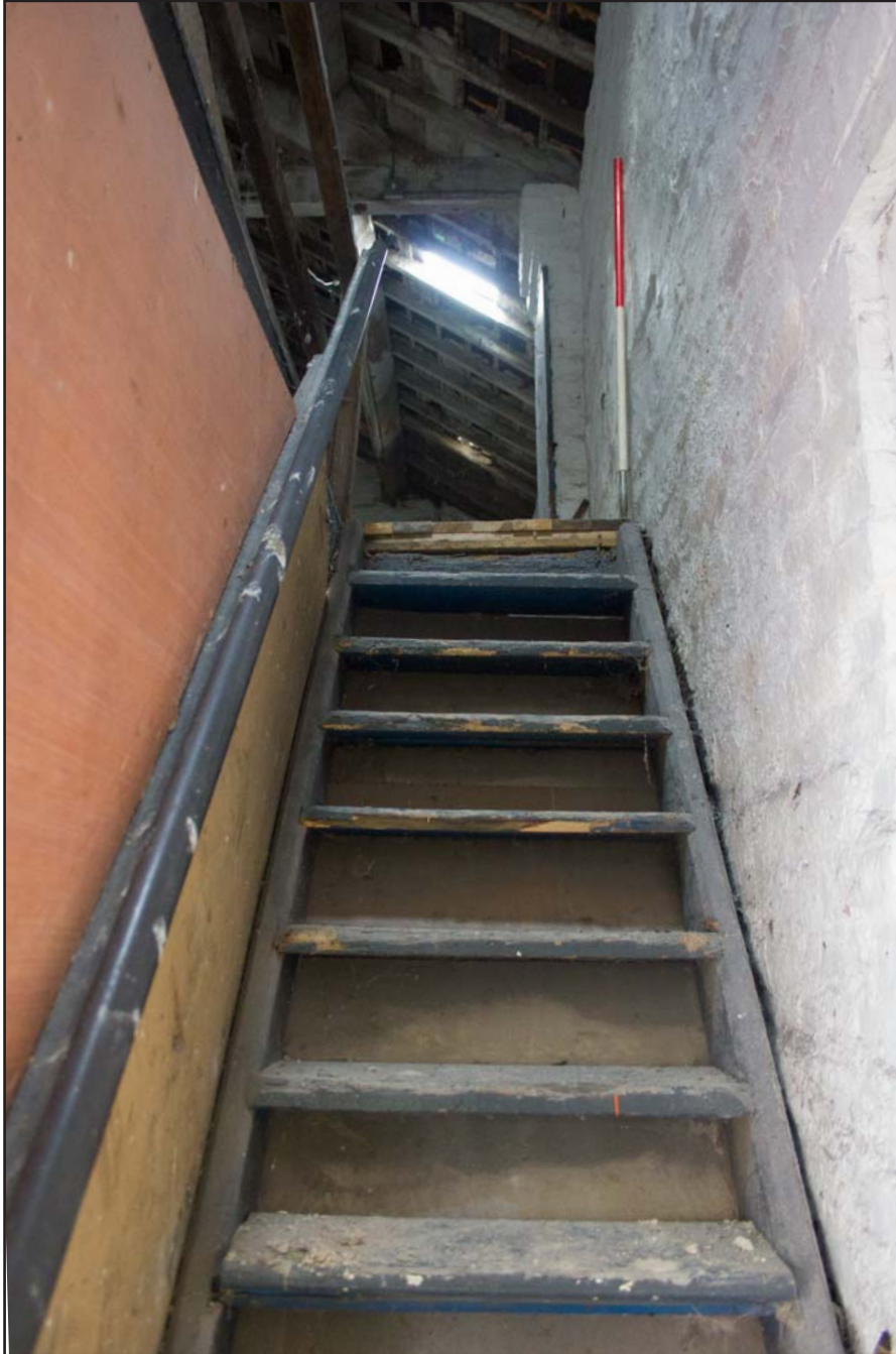
Plate 11: Stairwell, from the southeast. Scale 1.0m.
