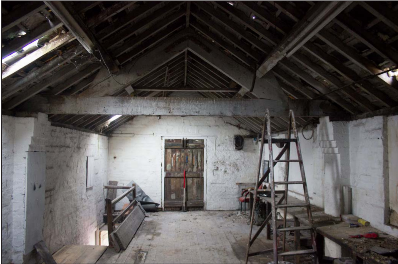
Plate 12: First floor Store, from the northwest. Scale 1.0m.
