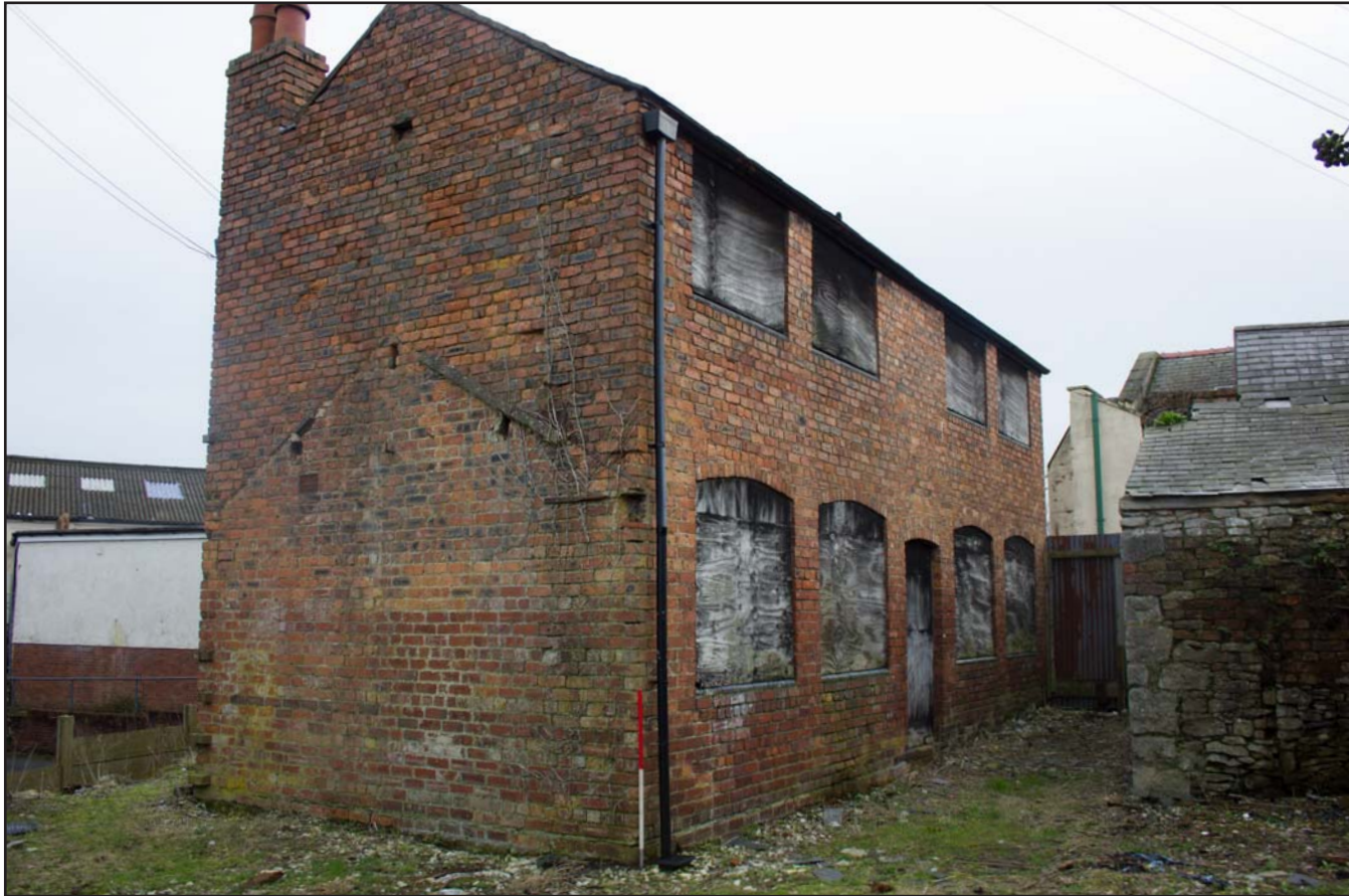
Plate 06: Northwest and southwest external elevations, from the west. Scale 1.0m.
