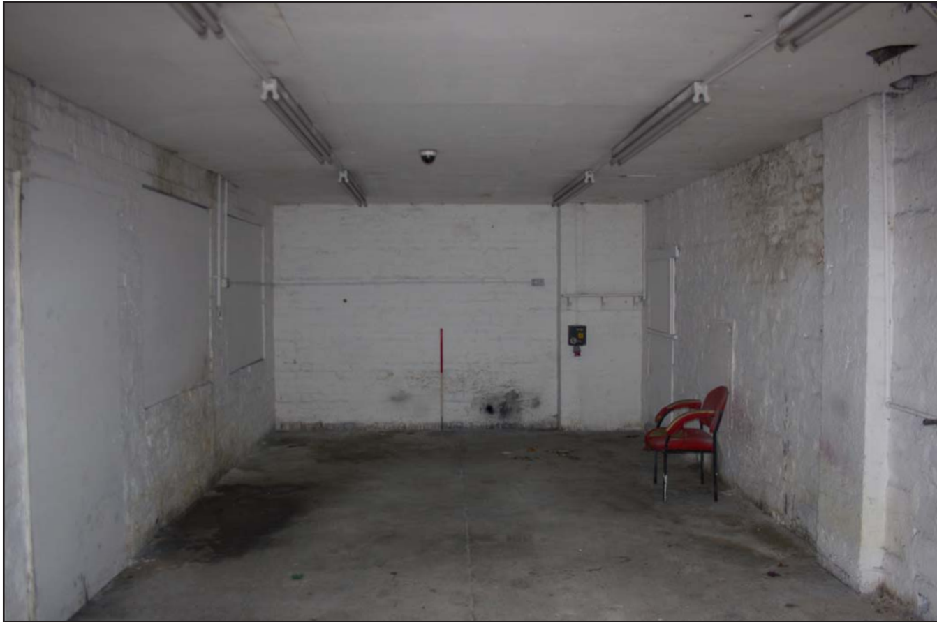
Plate 09: Ground floor workshop, from the southeast. Scale 1.0m.
