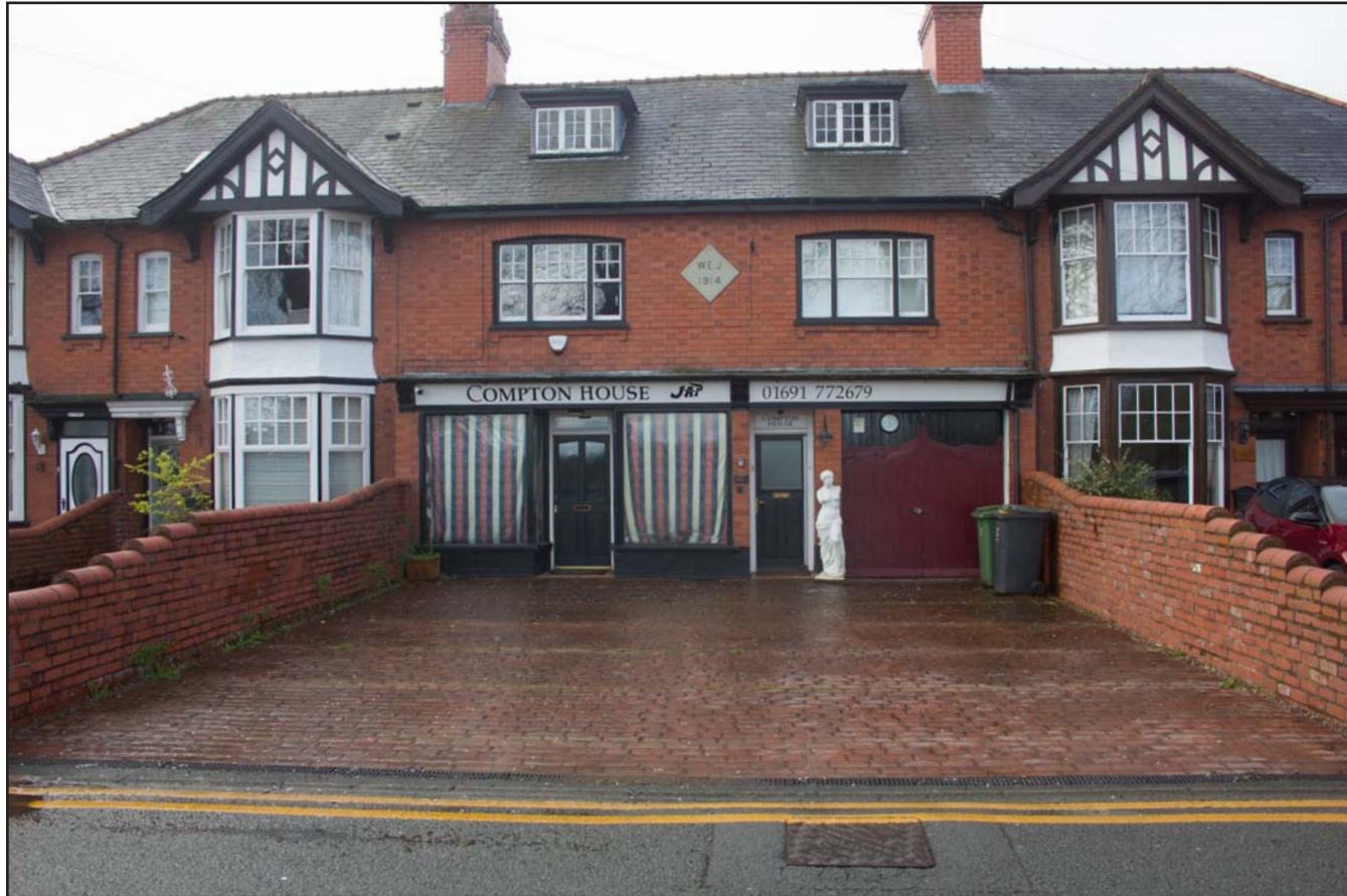
Plate 04: Shot of Compton House, 10 Station Avenue, Chirk, Wrexham - from the north - no scale
