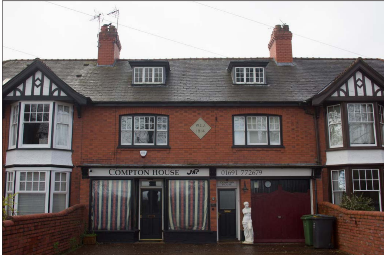
Plate 06: Focus shot of frontage of Compton House, 10 Station Avenue, Chirk, Wrexham - from the north - no scale
