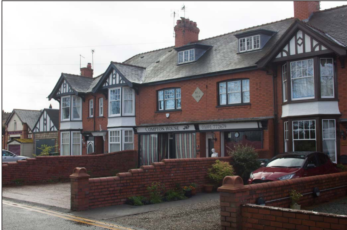
Plate 03: Shot of Compton House, 10 Station Avenue, Chirk, Wrexham - from the northwest - no scale
