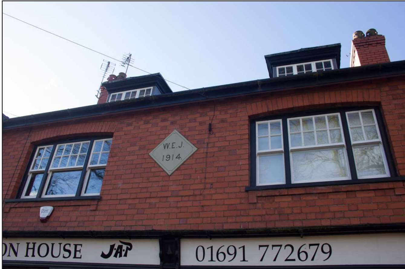
Plate 08: First floor date stone os Compton House, 10 Station Avenue, Chirk, Wrexham - from the northwest - no scale
