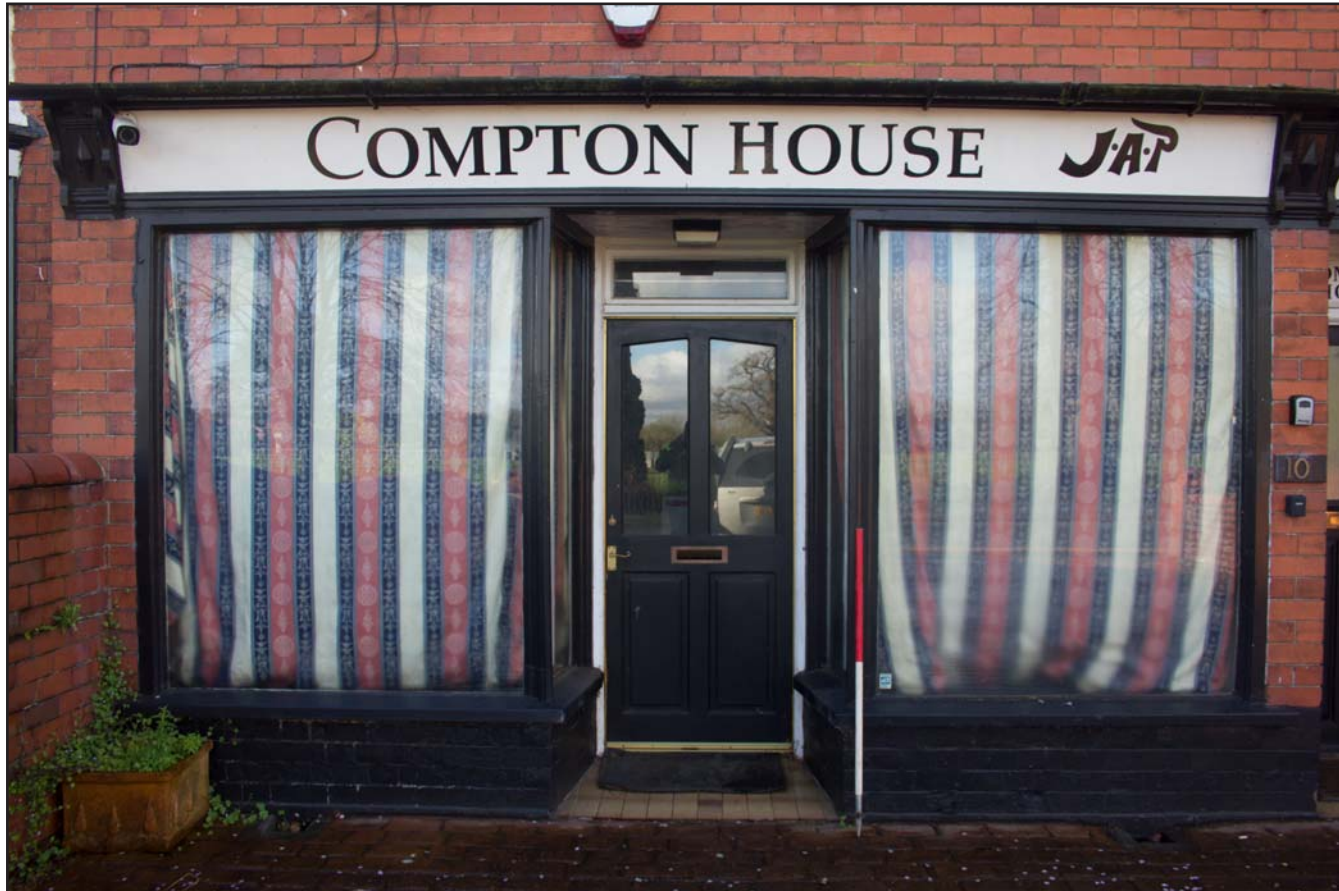
Plate 07: Former shop front of Compton House, 10 Station Avenue, Chirk, Wrexham - from the north - 1.00m scale
