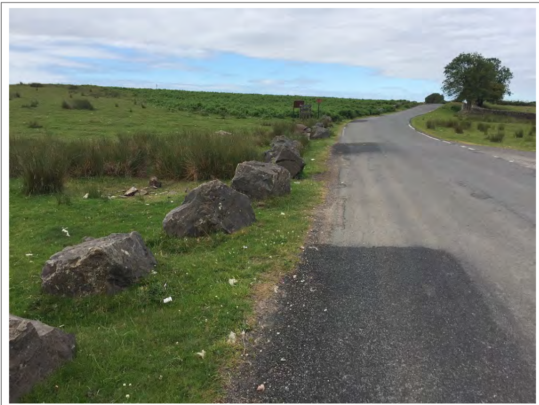
Plate 4. Example of how stone blocks will look upon completion
