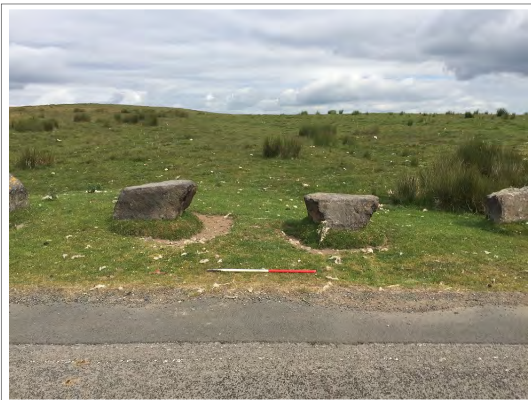
Plate 18. Roadblocks at GM556 showing wear from livestock, 1m scale
