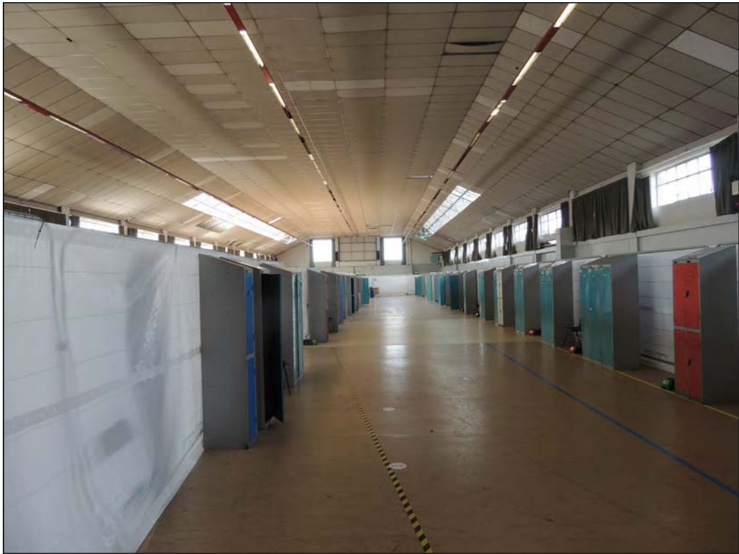
Plate 115. View of the sports hall looking NW
