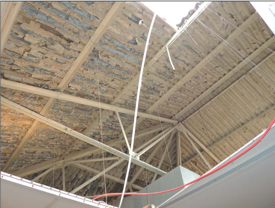
Plate 144. Oblique view of the roof structure above the food hall
