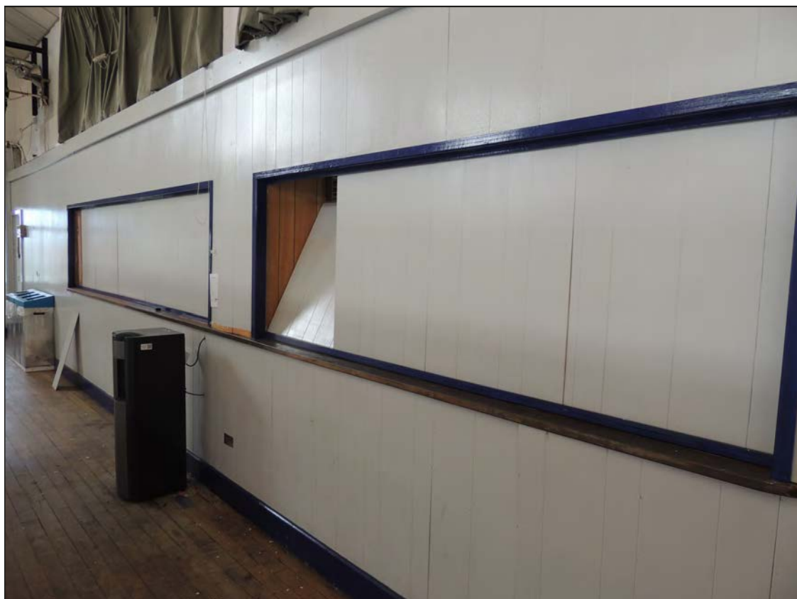
Plate 128. View of blocked hatches in the sports hall bar looking N
