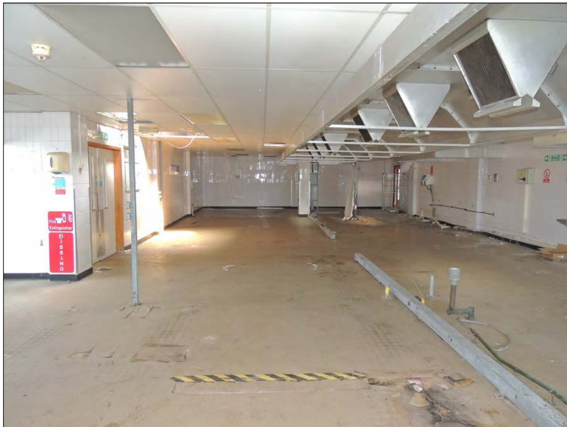
Plate 146. View of the kitchen looking NE
