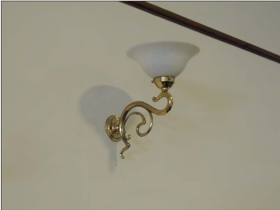
Plate 25. Oblique detailed view of the upright wall lights in the function room
