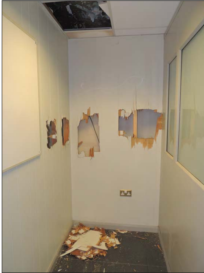
Plate 139. View of make-shift cupboard in office area looking NW
