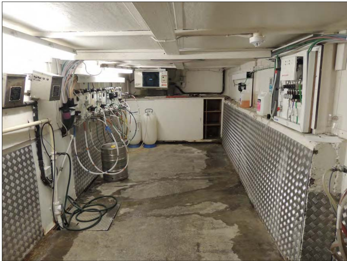
Plate 52. View of cellar beneath the bar looking NNE
