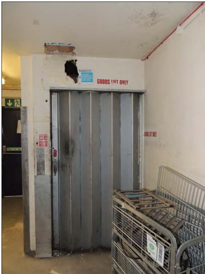
Plate 148. View of the lift looking SE
