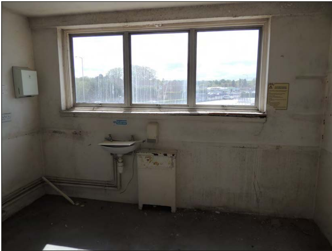
Plate 147. View of room off the kitchen looking S
