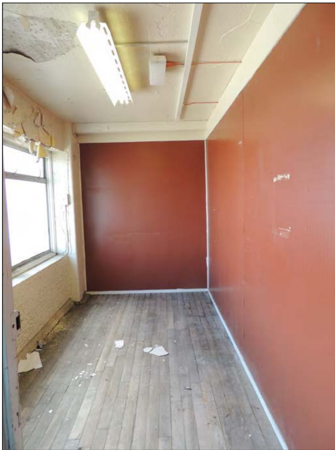
Plate 122. View of small room off the sports hall looking SE
