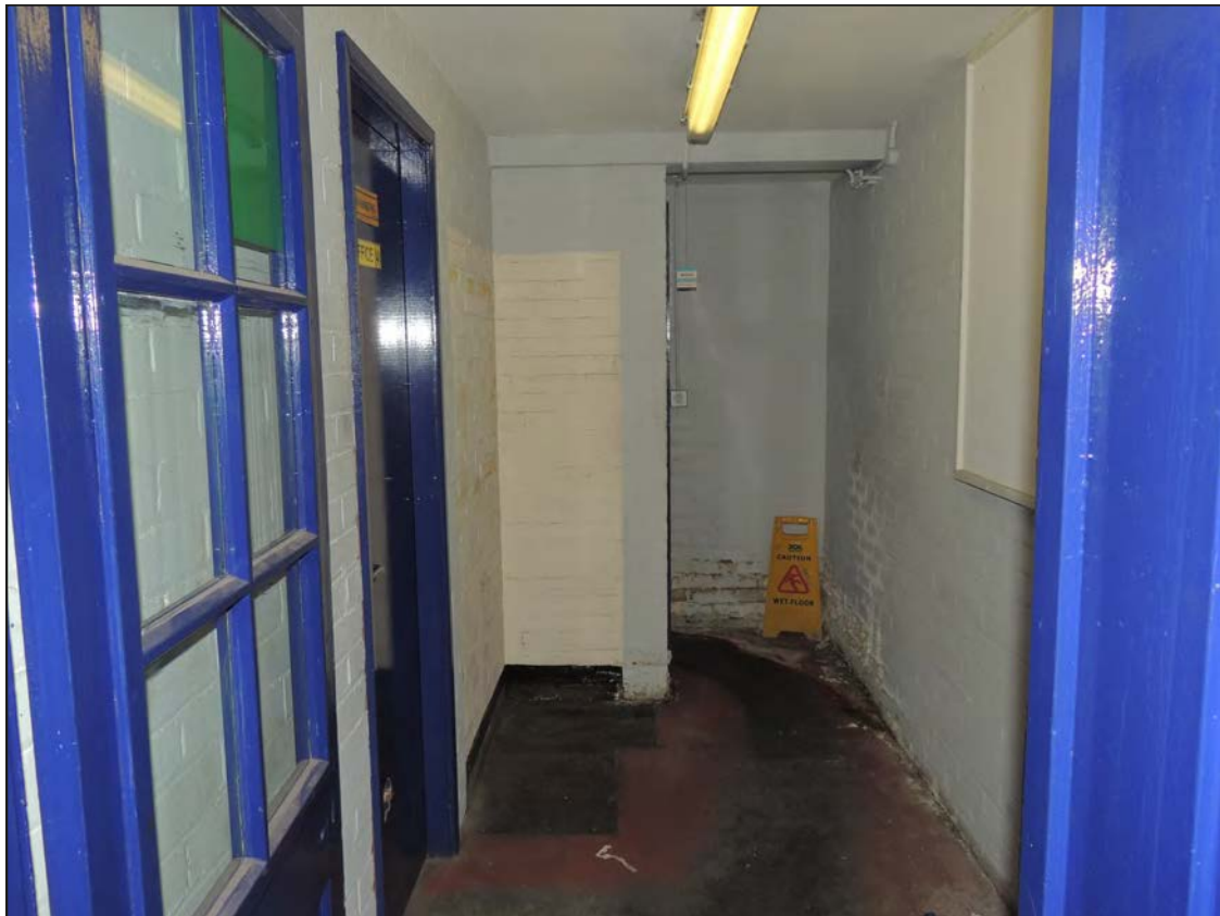
Plate 109. View of the corridor of the staff area in the garage looking SW
