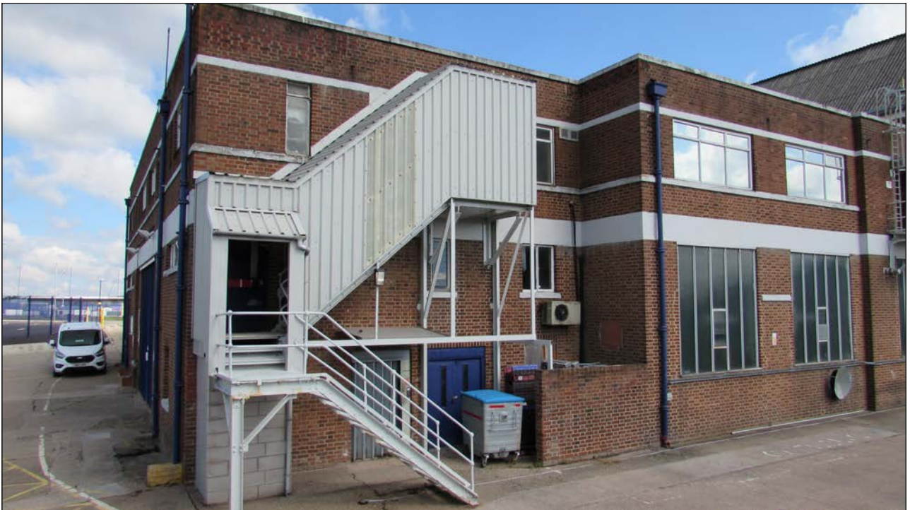
Plate 9. SE facing elevation, fire scape.
