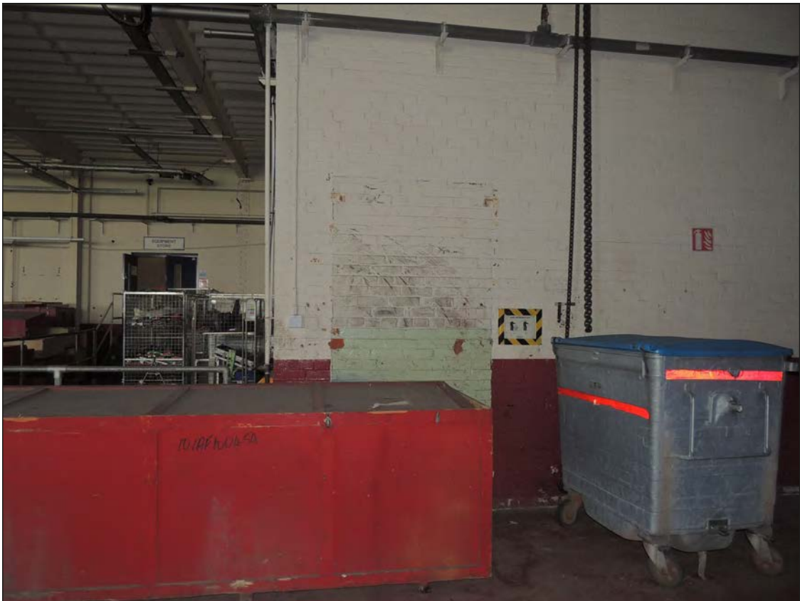
Plate 107. View of a blocked doorway in the garage looking NW
