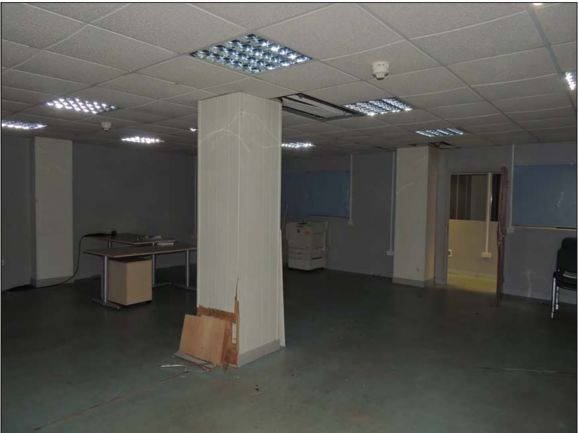
Plate 136. View of offices looking W
