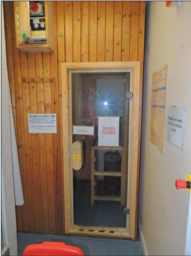
Plate 86. View of the sauna looking NW
