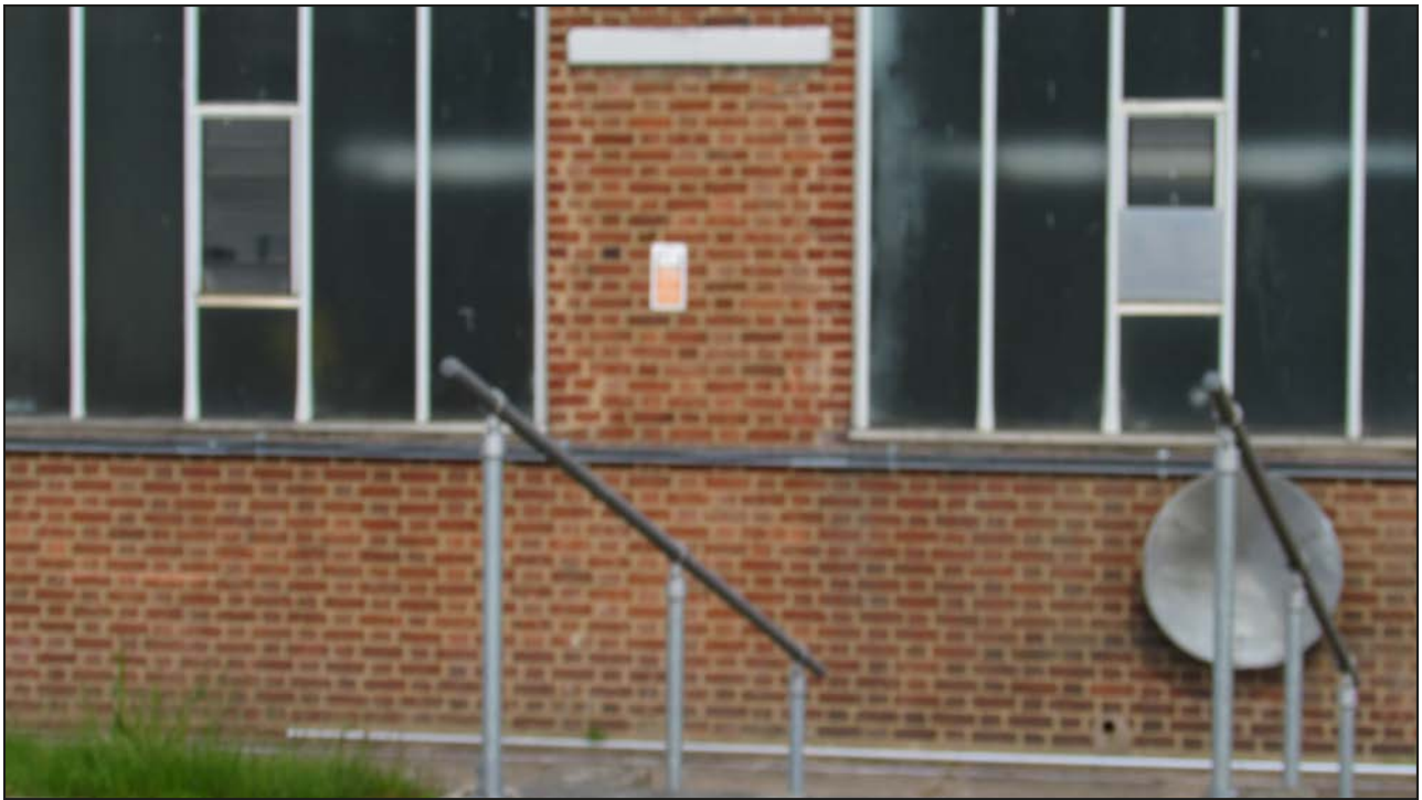
Plate 11. SE facing elevation, former door.
