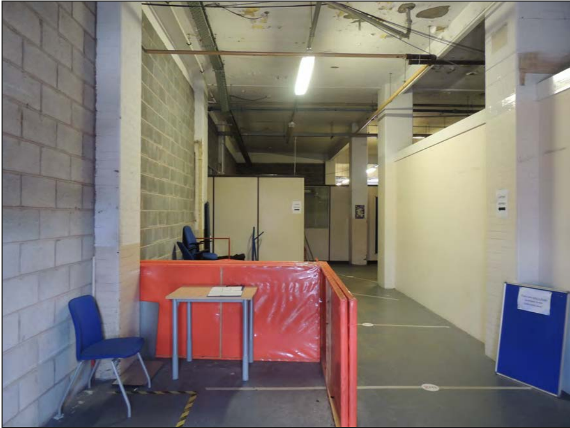
Plate 66. View of the entrance to the transport area looking NE
