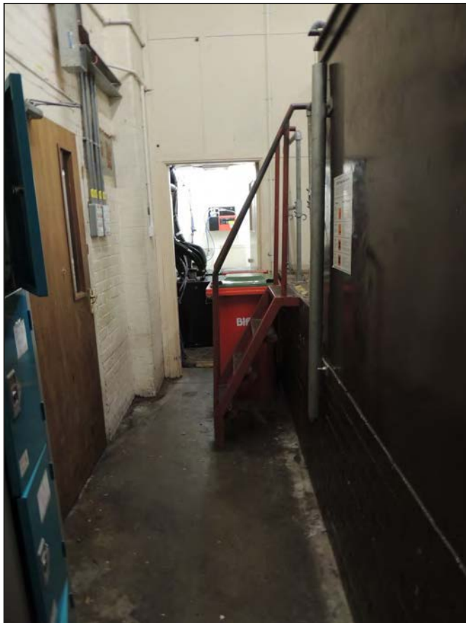
Plate 55. View of the lower levels of the beer store and bottle store looking NNE
