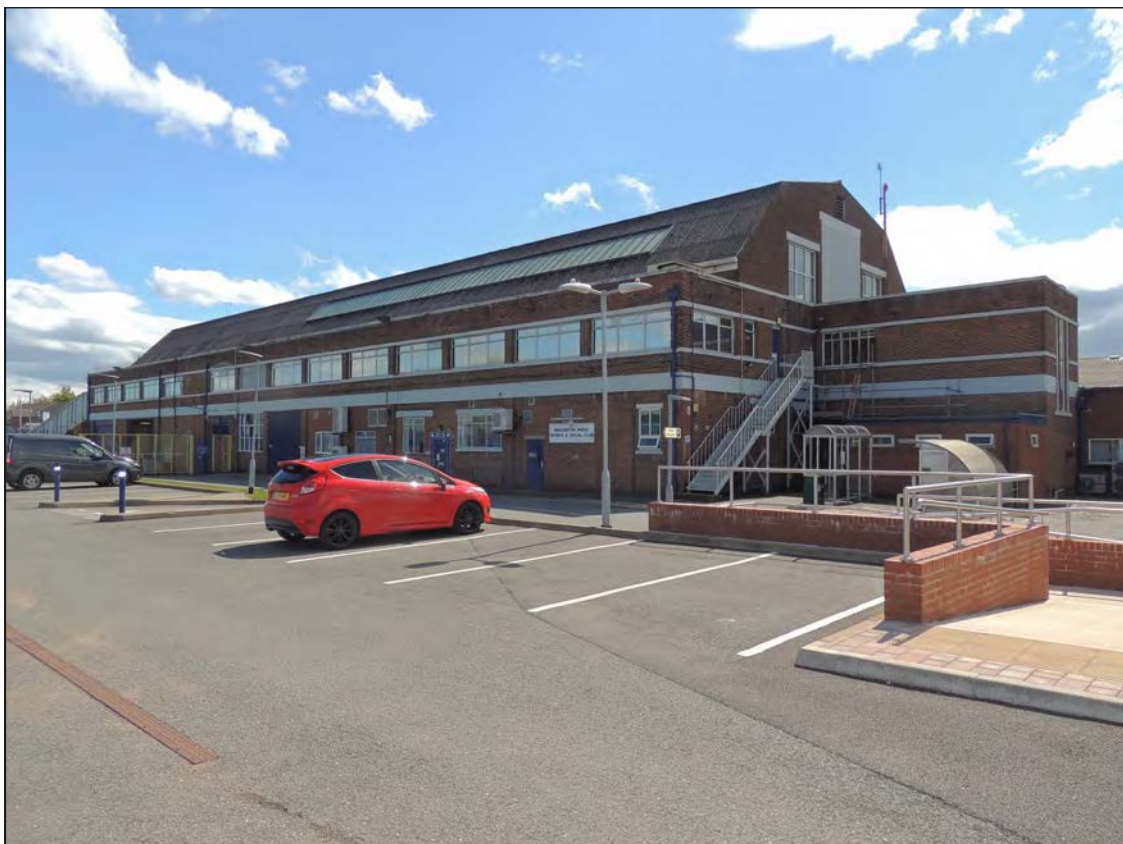
Plate 2. Oblique S facing shot of the NE facing elevation
