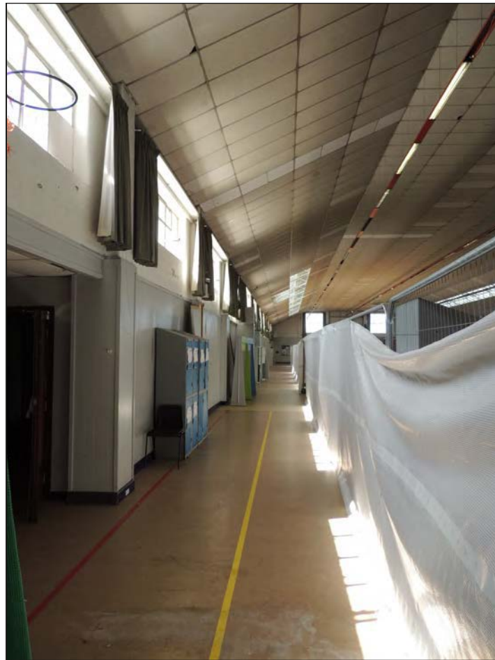
Plate 116. View of the sports hall looking NW
