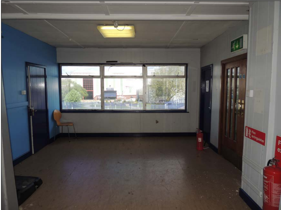
Plate 119. View of entrance to the sports hall from the SE end, looking NE
