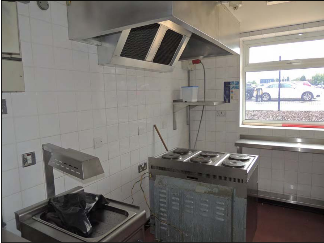
Plate 153. View of ground floor kitchen looking S
