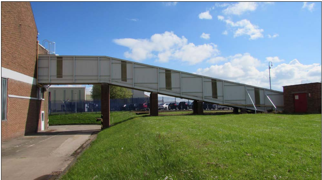
Plate 12. SE facing elevation, ramp.
