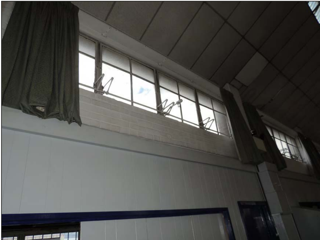
Plate 127. View of original windows in the sports hall
