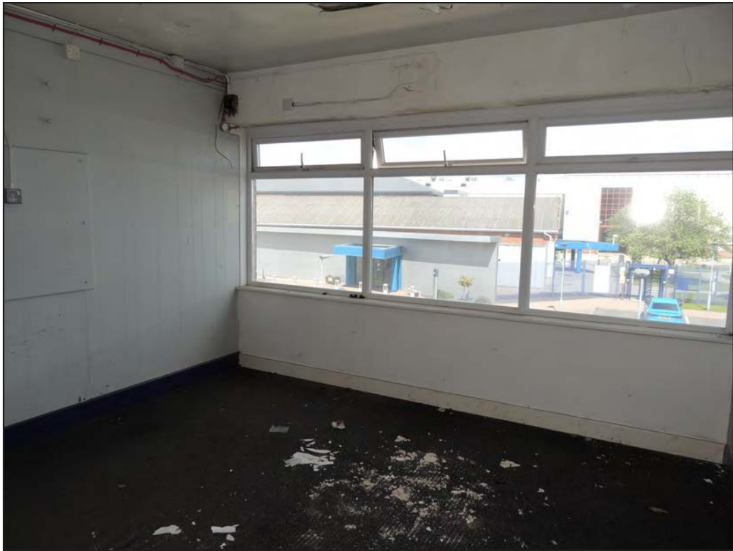
Plate 121. View of a upper bar storeroom looking NE
