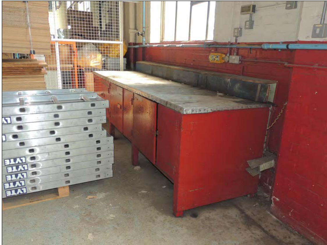
Plate 98. View of a workstation that may be original to the building, looking NEE
