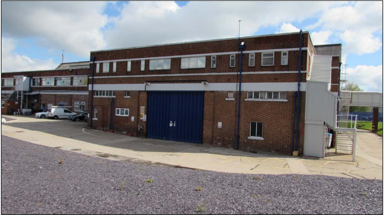
Plate 7. Projecting area from garage.
