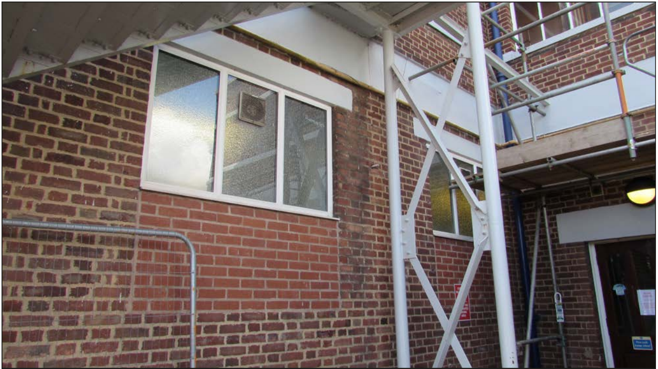
Plate 3. Repair details, NW facing elevation.
