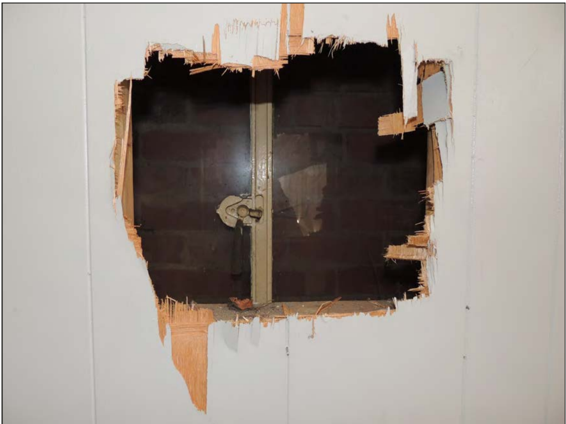
Plate 112. View of possible original windows behind wooden panels looking NW
