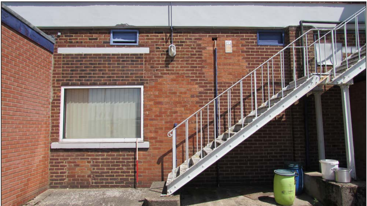
Plate 6. Alteration details, SW facing elevation.
