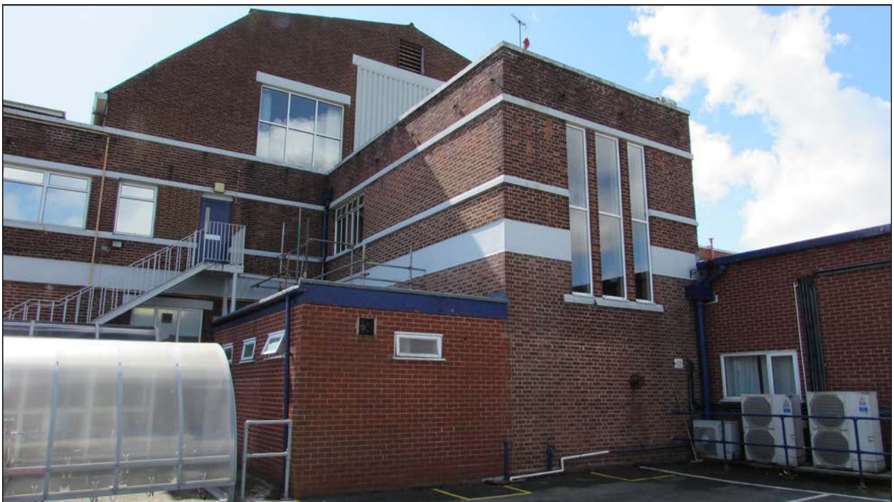
Plate 4. Repair details, NW facing elevation.
