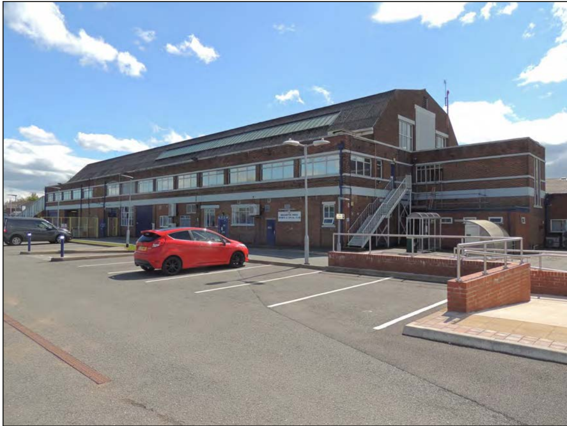
Plate 13. Oblique S facing shot of the NE facing elevation
