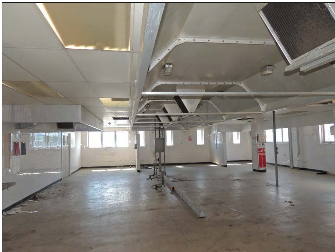
Plate 145. View of the kitchen looking SW
