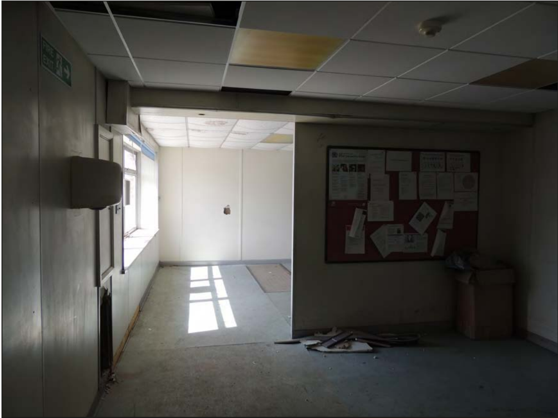
Plate 141. View of food hall area converted into offices looking NW
