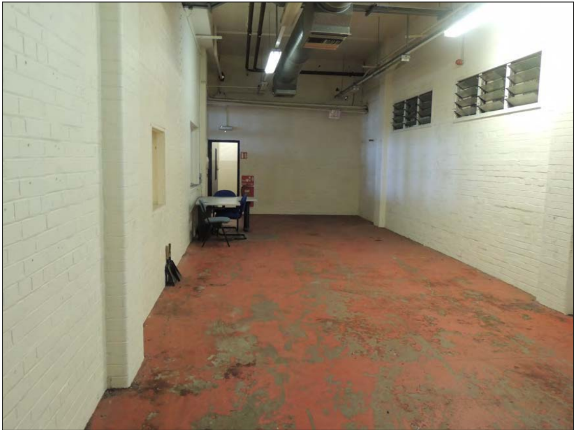
Plate 91. View of the long room between the transport and garage areas, looking SW
