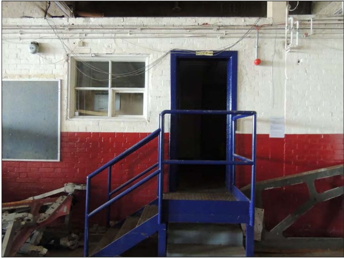
Plate 108. View of the staff area in the garage looking SW
