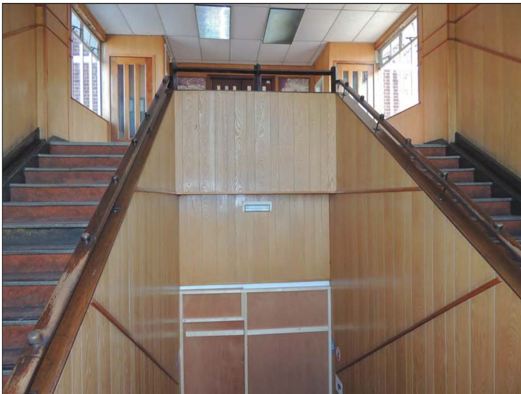
Plate 18. View of the main stairwell looking SEE
