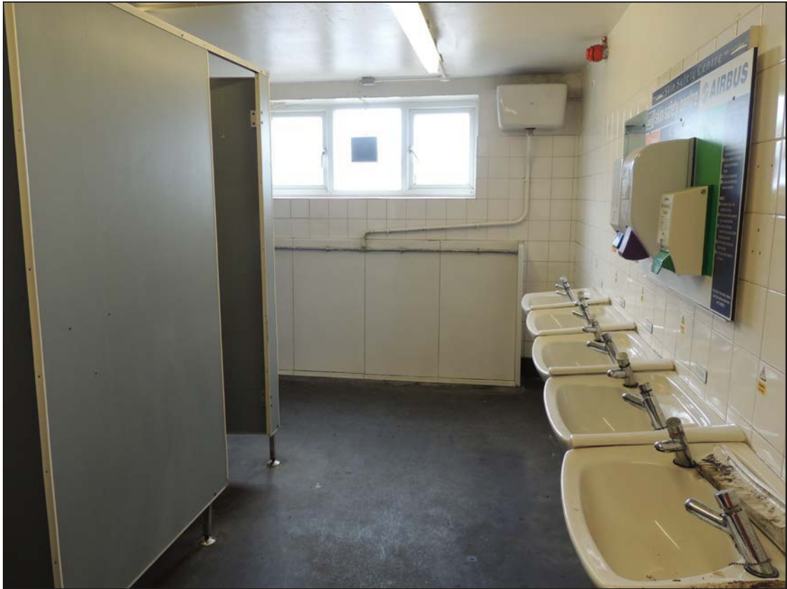
Plate 110. View of the mechanics toilets in the garage looking SW.
