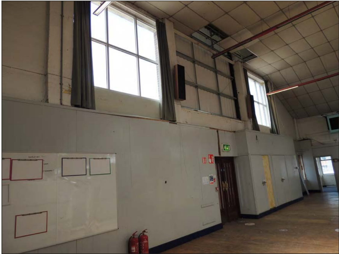
Plate 111. View of the entrance to the sports hall looking N
