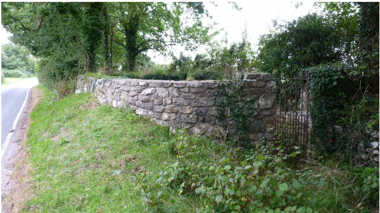
Photo 8: As above, view west showing the entrance to the pound.
