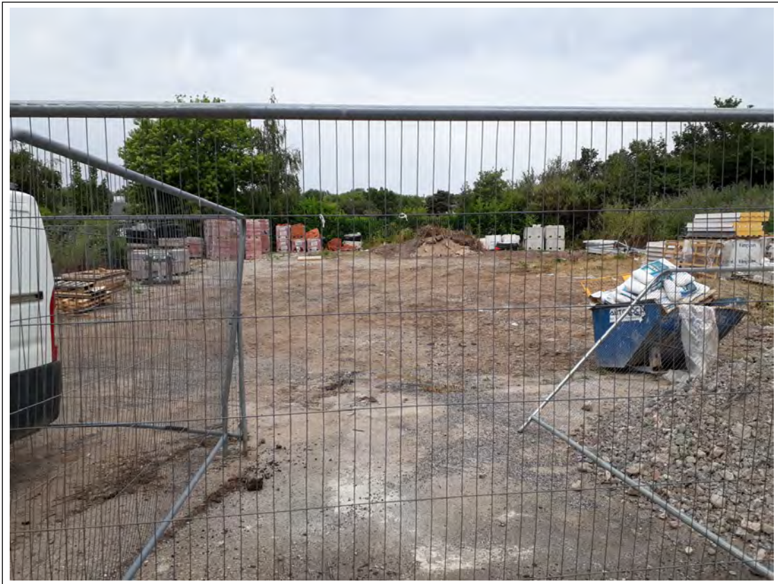
Plate 1. The site viewed from Earl Street. View NW
