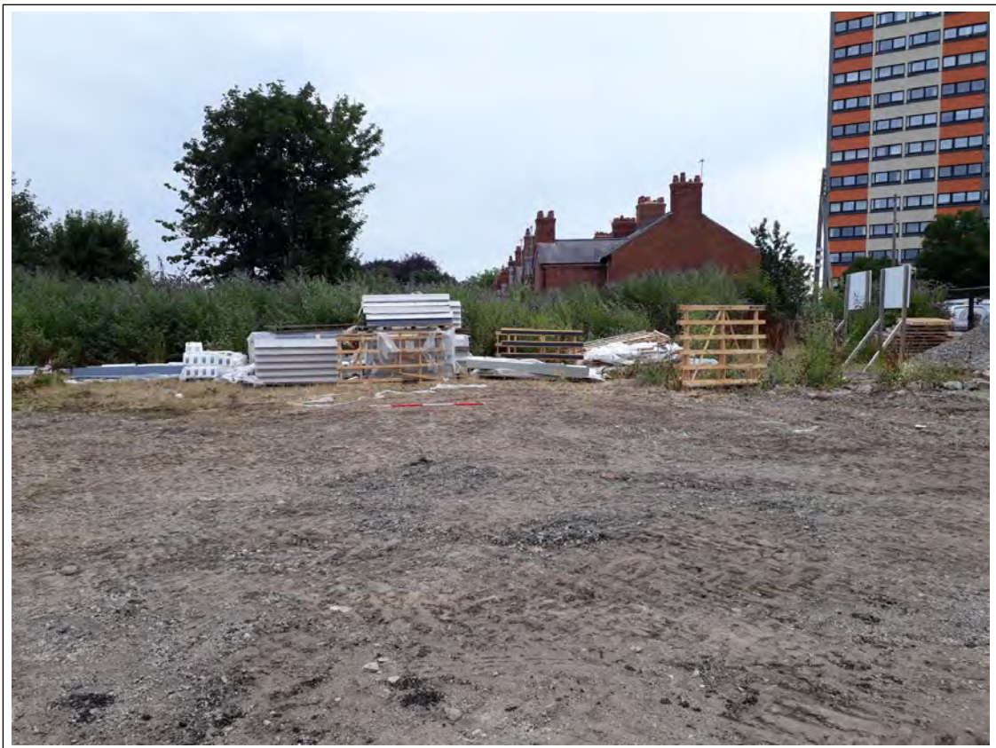
Plate 6. The site. View NE. 2m scale
