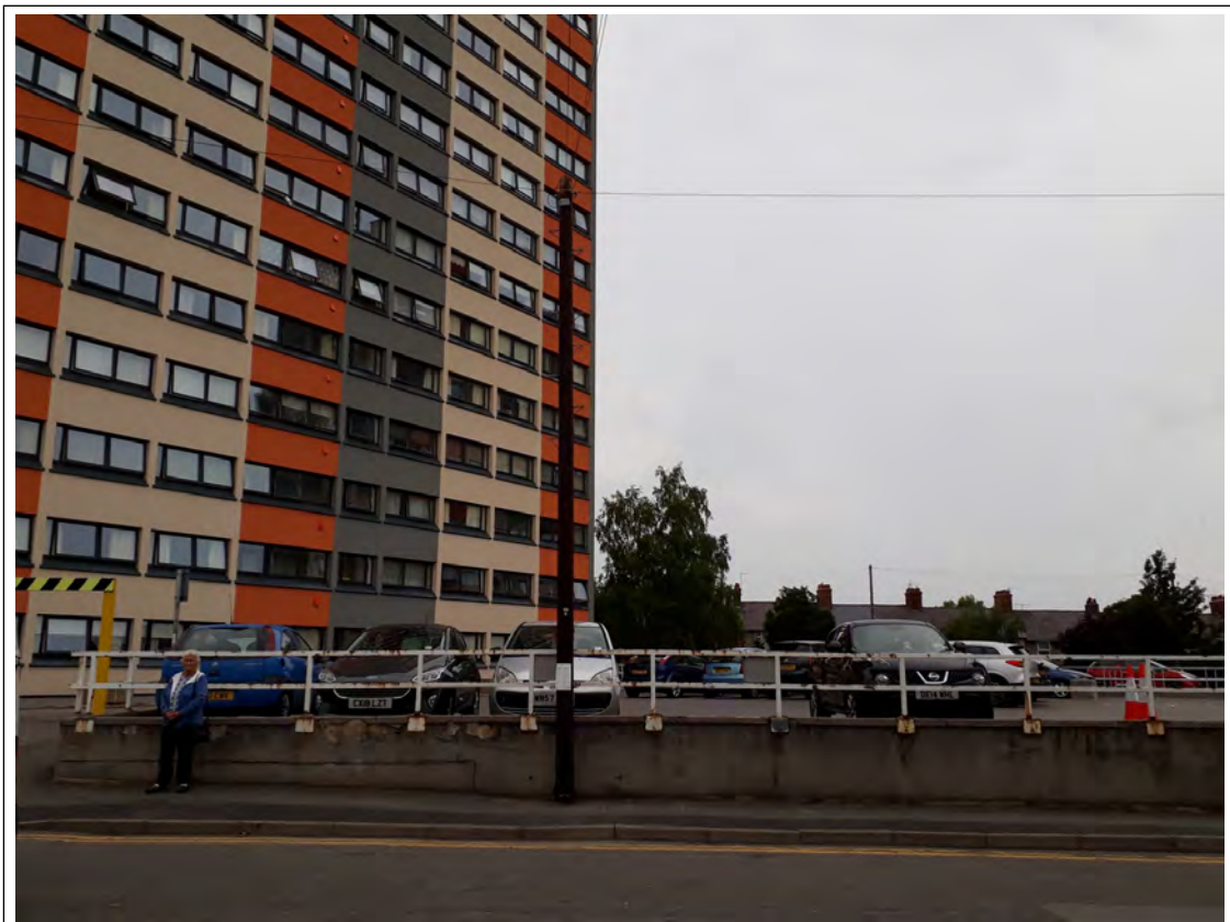
Plate 10. View from rear of LB 524 to the site. View NW
