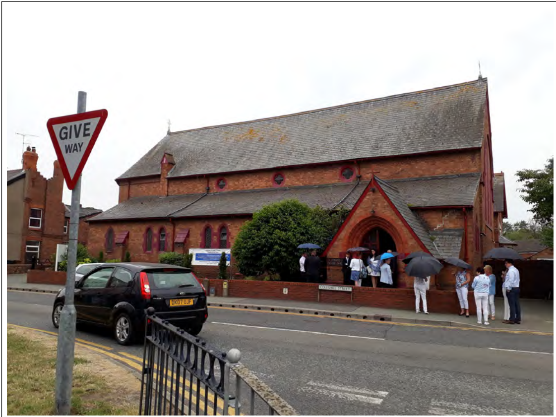
Plate 15. Flint Roman Catholic Chapel PRN 84179. View SW
