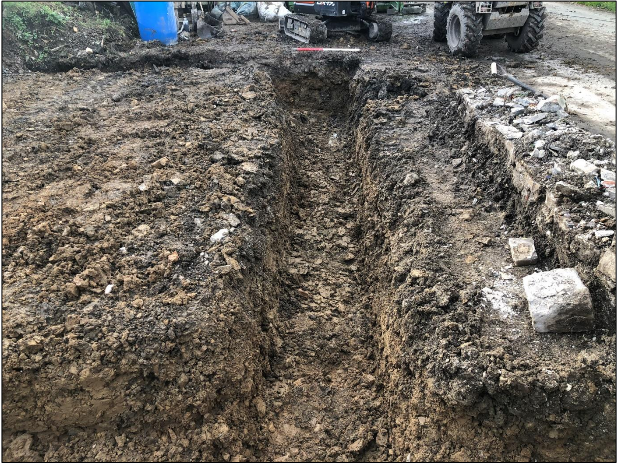
Plate 5. Footing trench 2, facing south-west, 1m scale
