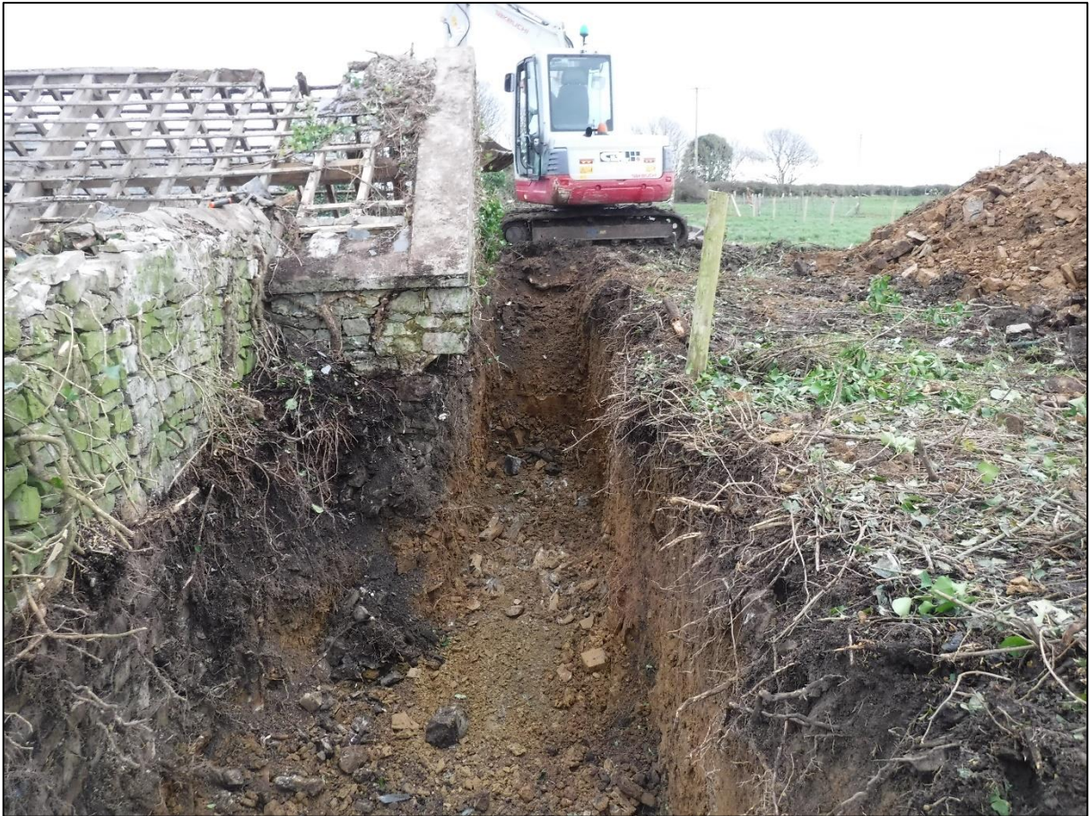
Plate 3. Working shot of phase one excavations, facing north-east
