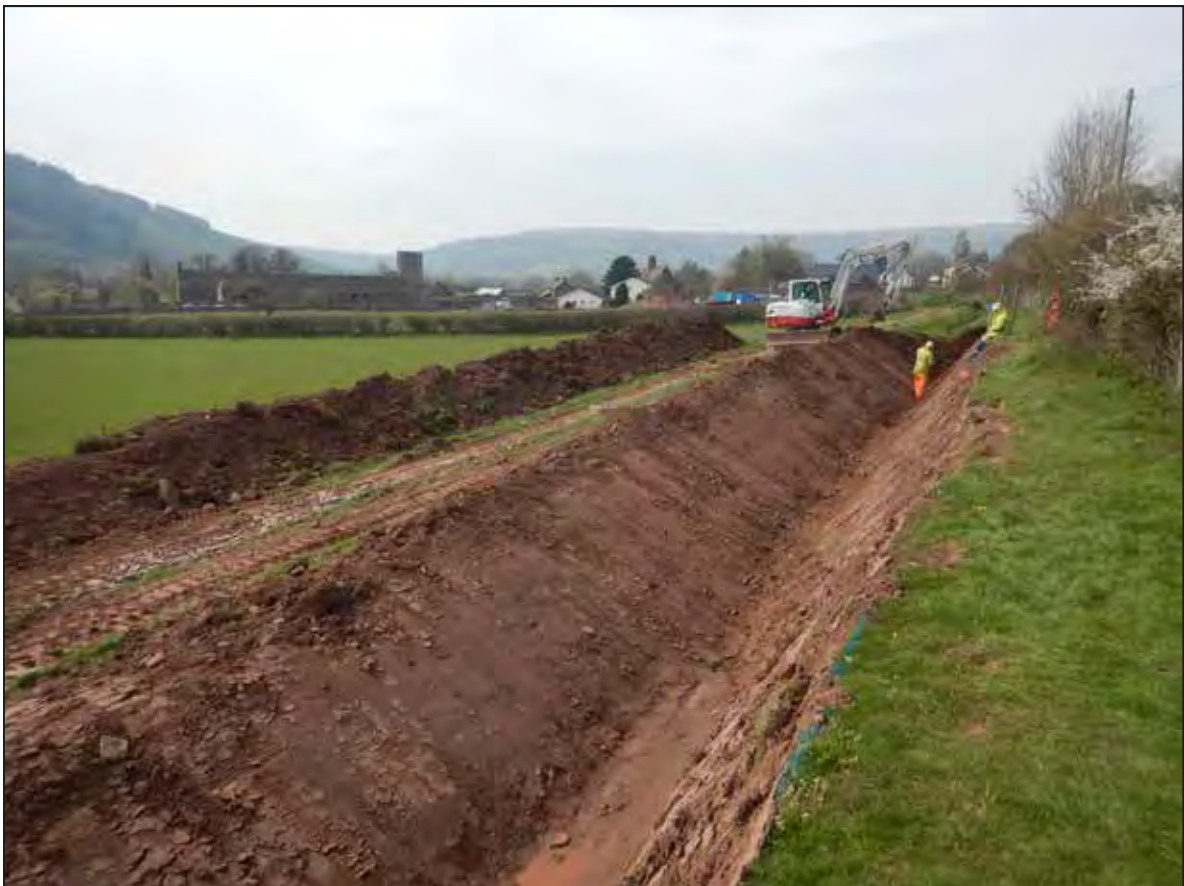
Plate 2. Trench 1, working shot, looking NW.
