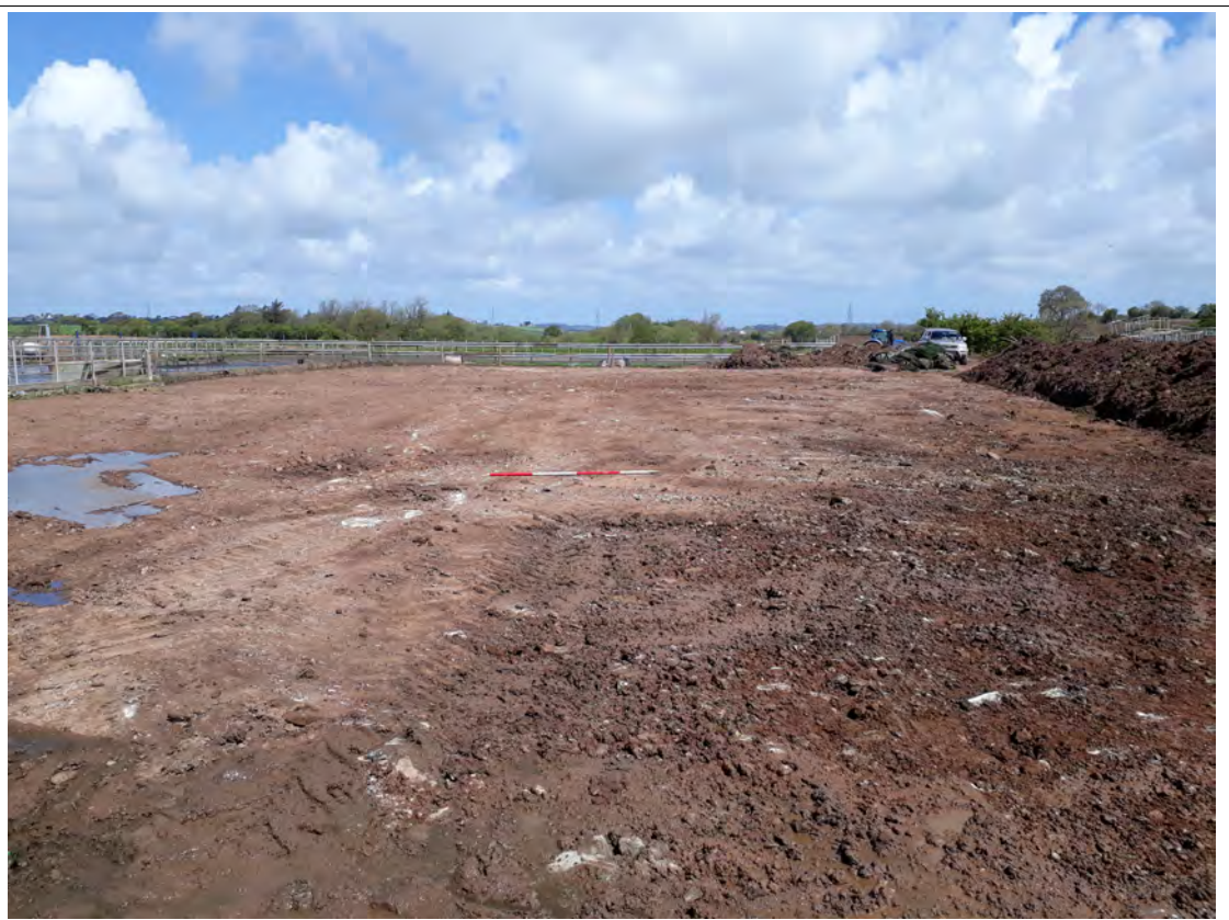
Plate 10. Site topsoil strip. View SW. 2m scale
