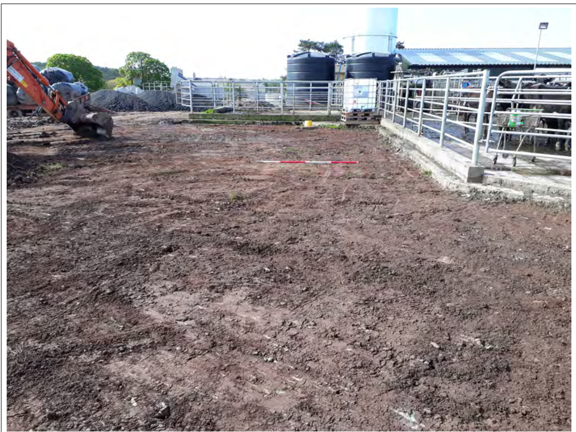
Plate 6. Site topsoil strip SW end of site. View SW. 2m scale
