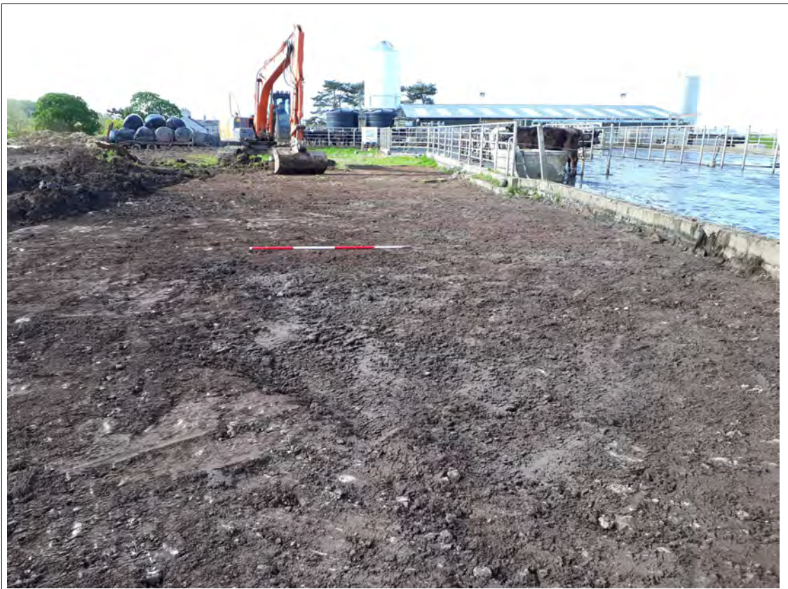
Plate 4. Site topsoil strip. View SW. 2m scale
