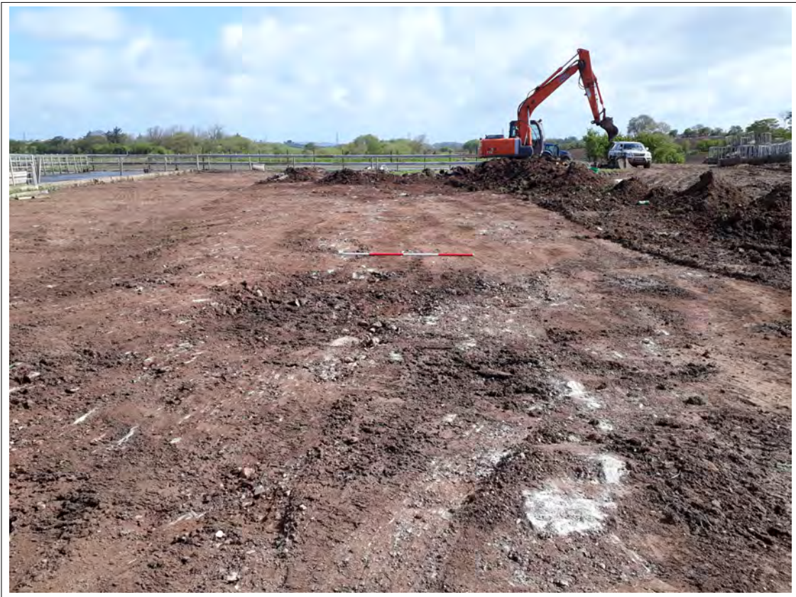
Plate 7. Site topsoil strip. View NE. 2m scale
