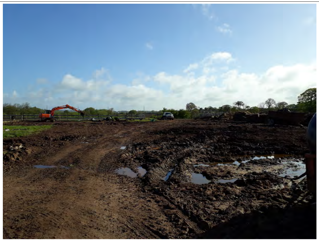
Plate 2. Site prior to topsoil strip. View NE. 2m scale
