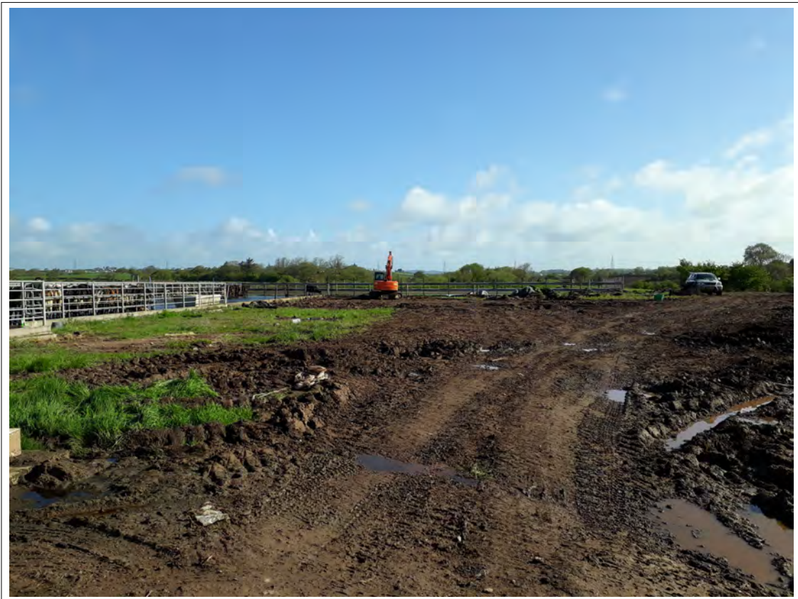
Plate 1. Site prior to topsoil strip. View NE. 2m scale
