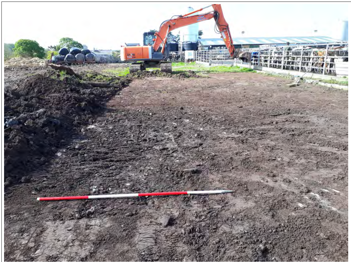
Plate 5. Site topsoil strip. View SW. 2m scale
