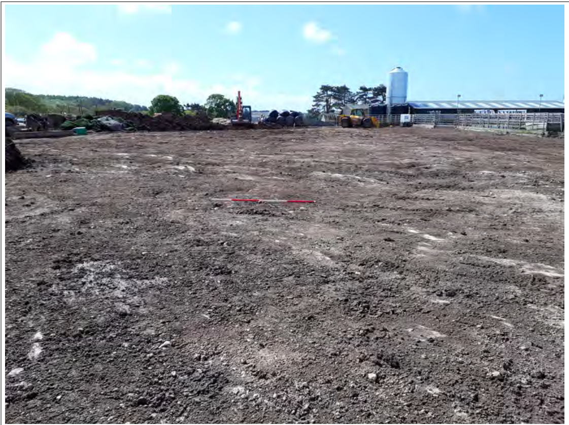
Plate 9. Site topsoil strip. View SW. 2m scale
