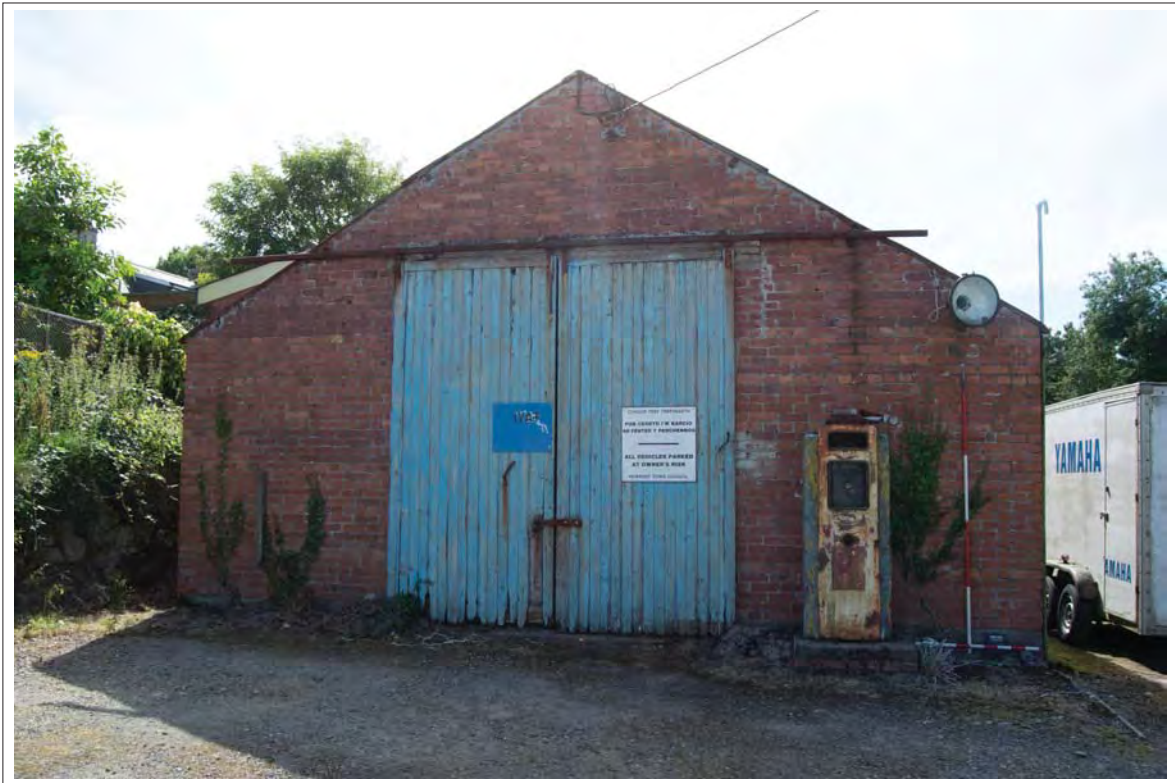
Plate 13. The southern area, garage detail. View west. 2m scale.
