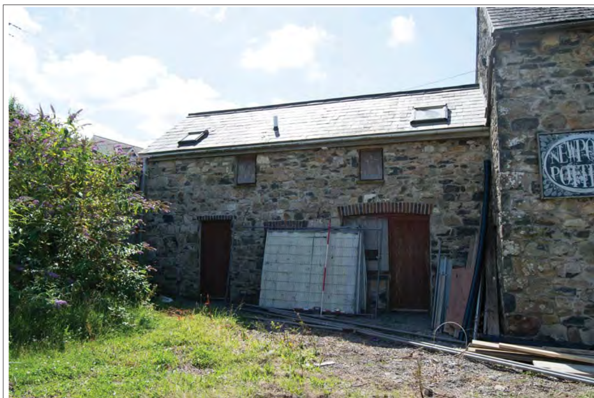
Plate 4. The Pottery elevation. View west. 2m scale.
