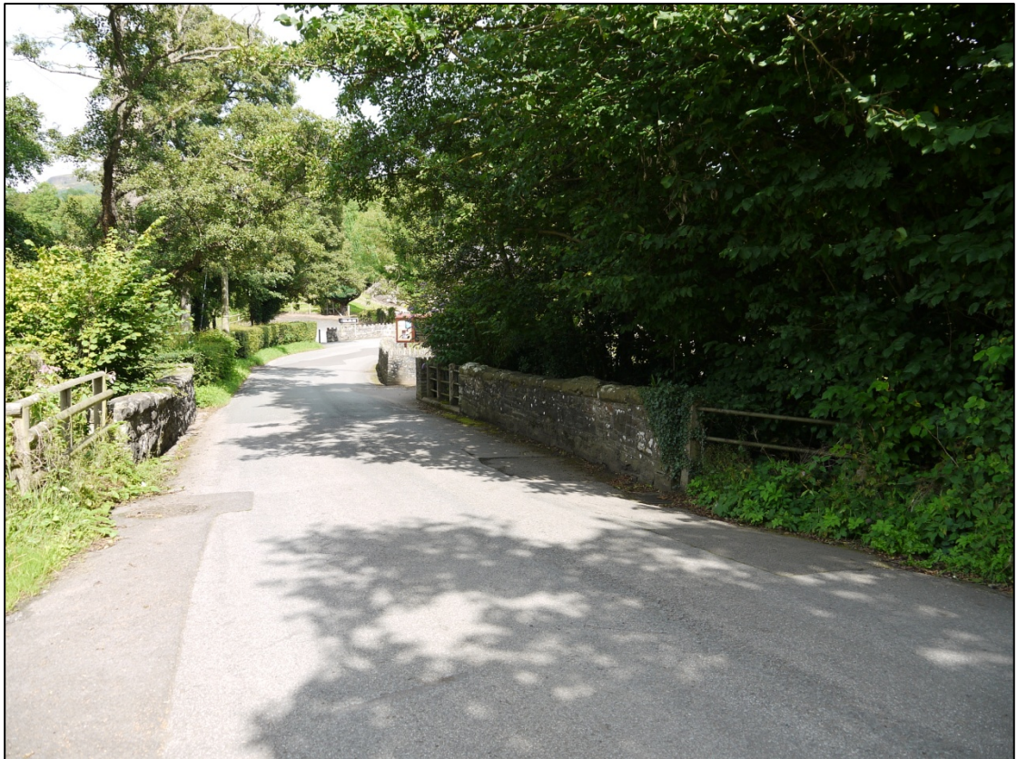
Photo 14: Stone bridge looking east
