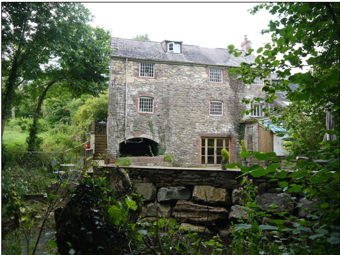
Photo 8: North end on east bank looking west to former corn mill
