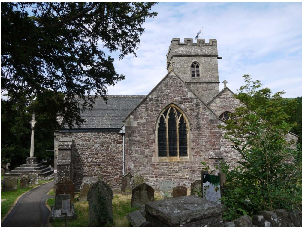
Photo 25: East end of St Teilos church, looking west
