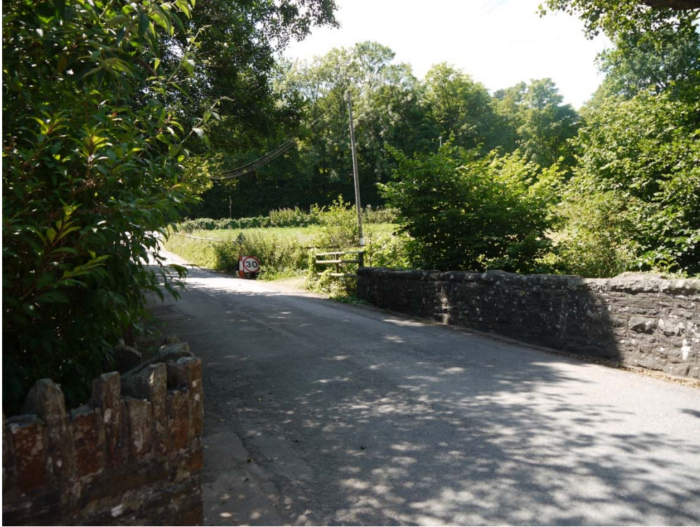
Photo 30: View from lychgate looking northwest across bridge to site
