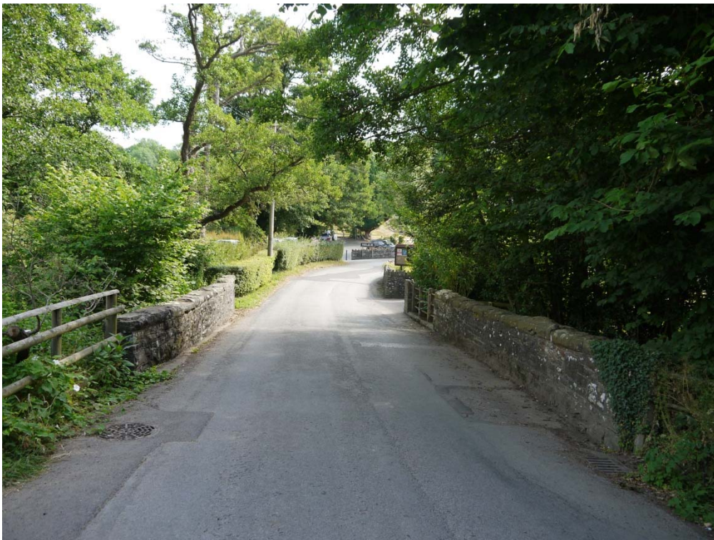
Photo 29: Stone bridge looking east
