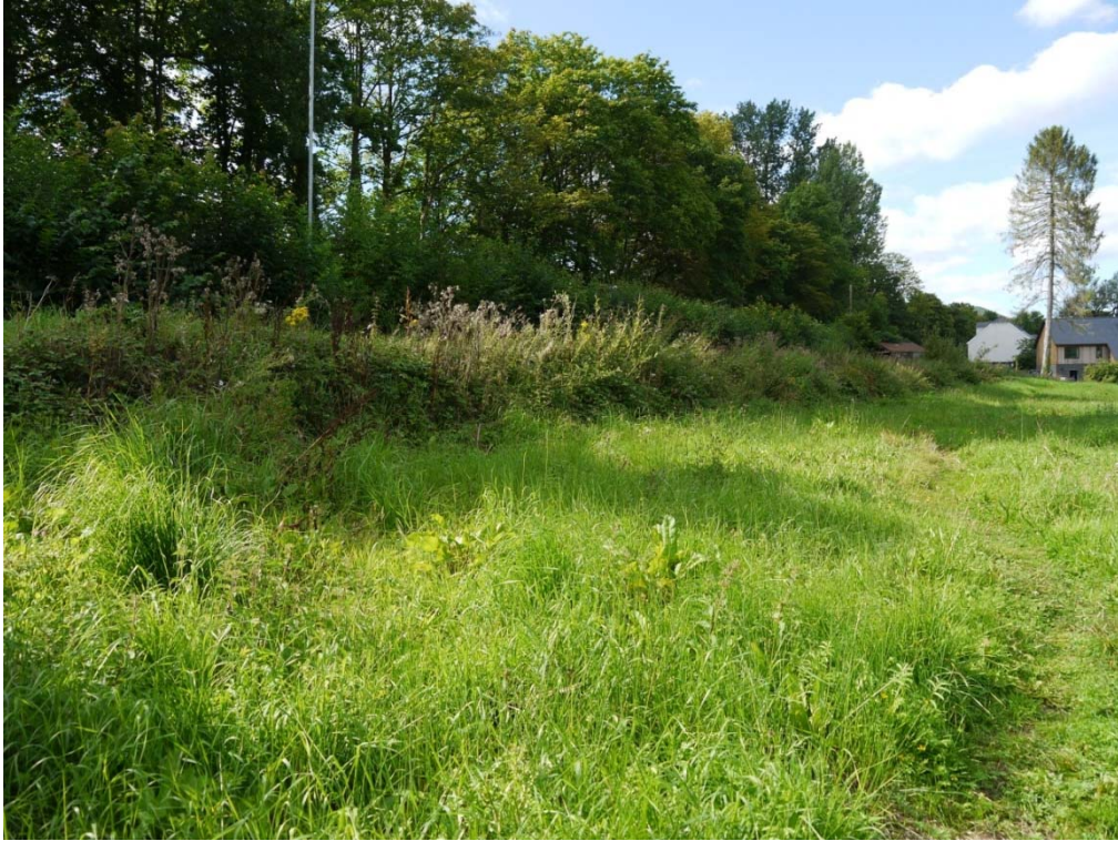
Photo 17: Tramway embankment as seen in 2017
