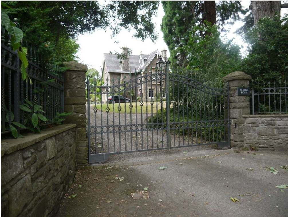
Photo 34: St Teilos House, looking southwest
