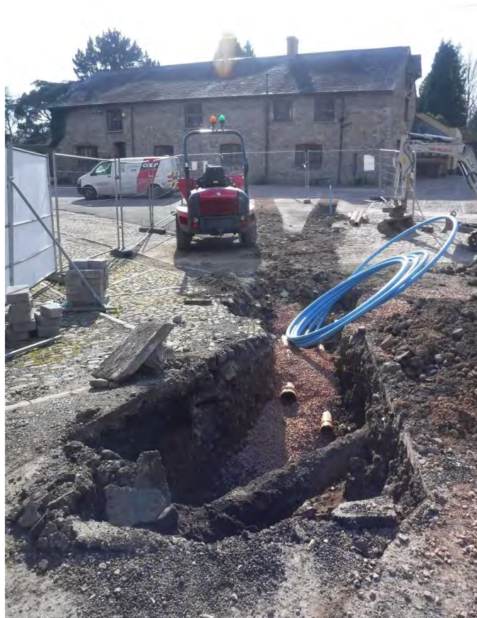
Photo 9: General shot looking southwest along the partially backfilled Trenches 1 & 2.
