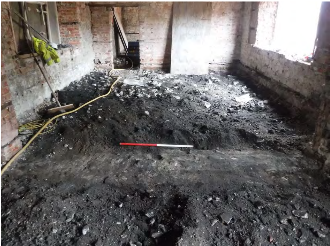
Photo 32: Laundry Building, Room 5, viewed from Room 4. Shot facing west, showing wall foundations (174) in the foreground. 1m scale.
