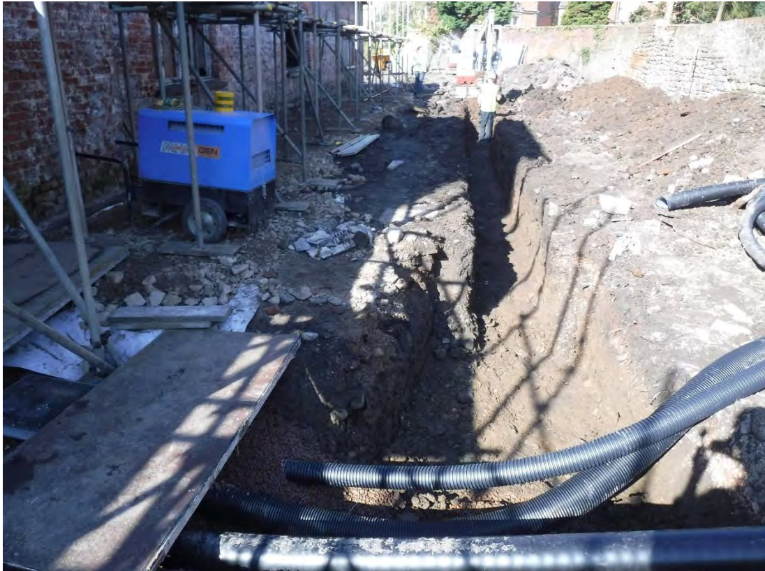
Photo 35: Trench 4 under excavation, shot facing west.
