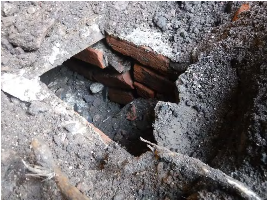
Photo 26: Laundry Building, Entranceway. Shot facing northeast, showing the partial revealed remains of drain (179).
