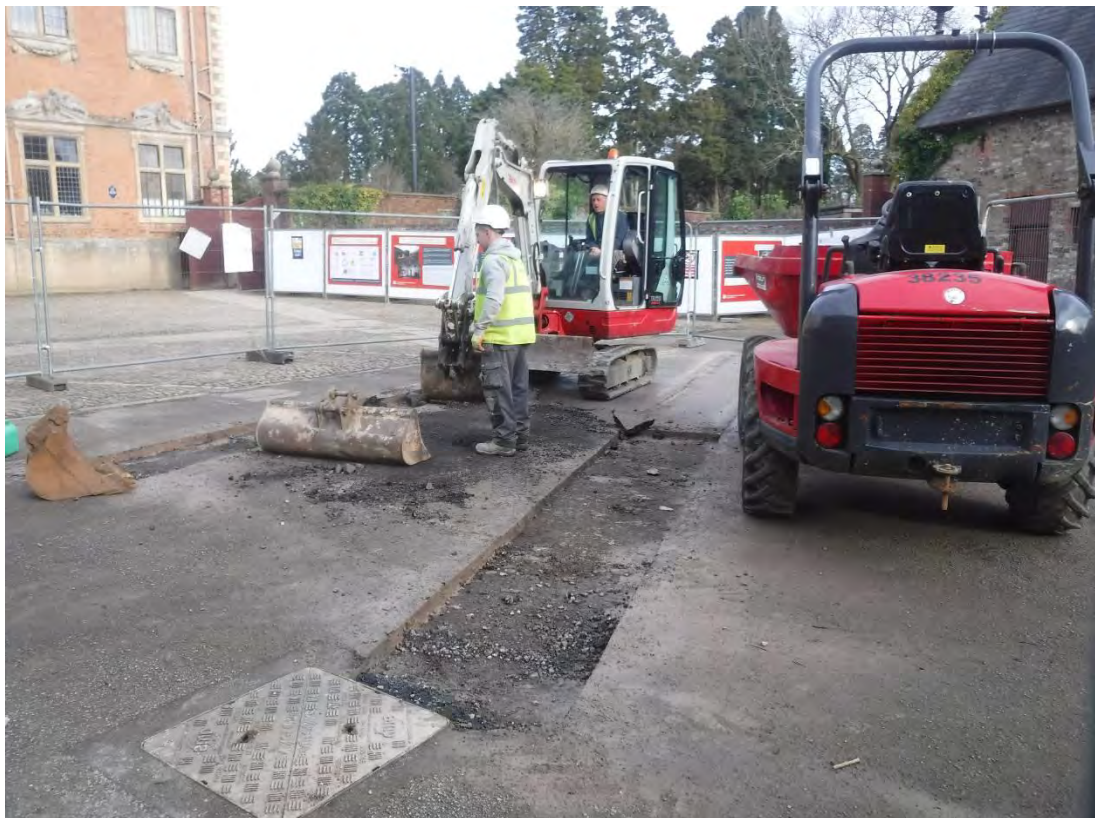
Photo 2: Shot facing northeast showing the commencement of groundworks, excavating Trenches 1 & 2.
