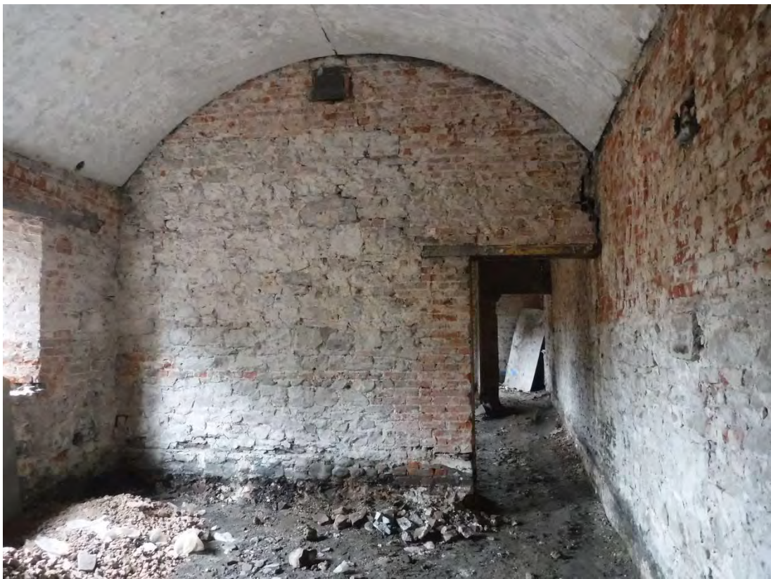
Photo 22: Laundry Building, Room 3. Shot facing east, showing internal wall.
