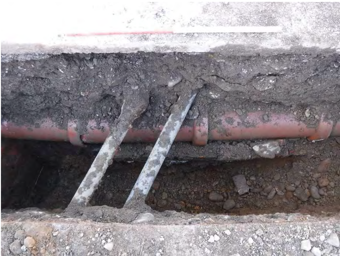
Photo 4: Trench 1, shot facing northwest showing ceramic drainpipe 107. 1m scale.
