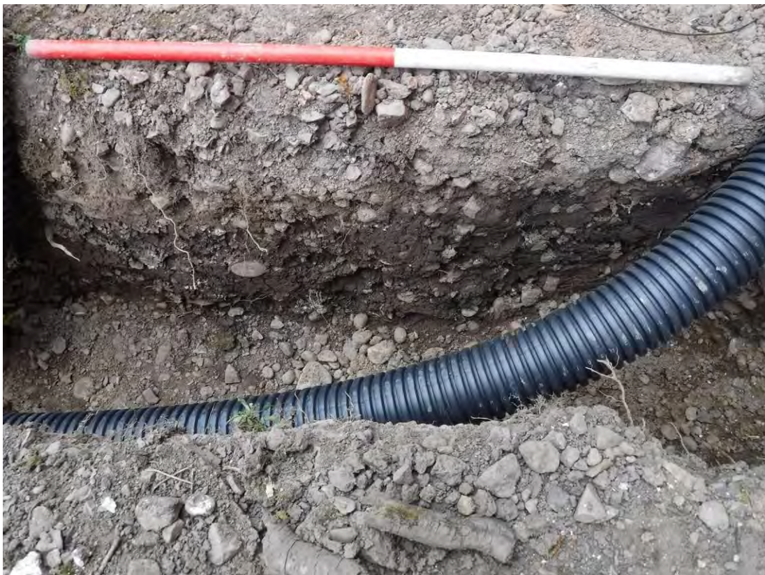
Photo 46: Trench 8, shot facing east, showing deposits (212) and (209). 1m scale.
