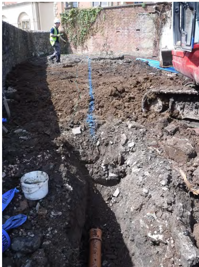
Photo 40: Trench 6 under excavation, shot facing west.
