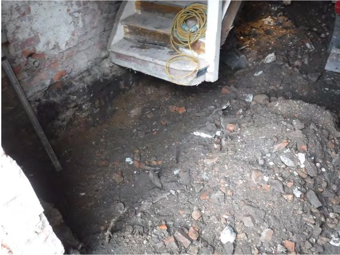
Photo 27: Laundry Building, Entranceway. Shot facing southeast, showing deposit (172).
