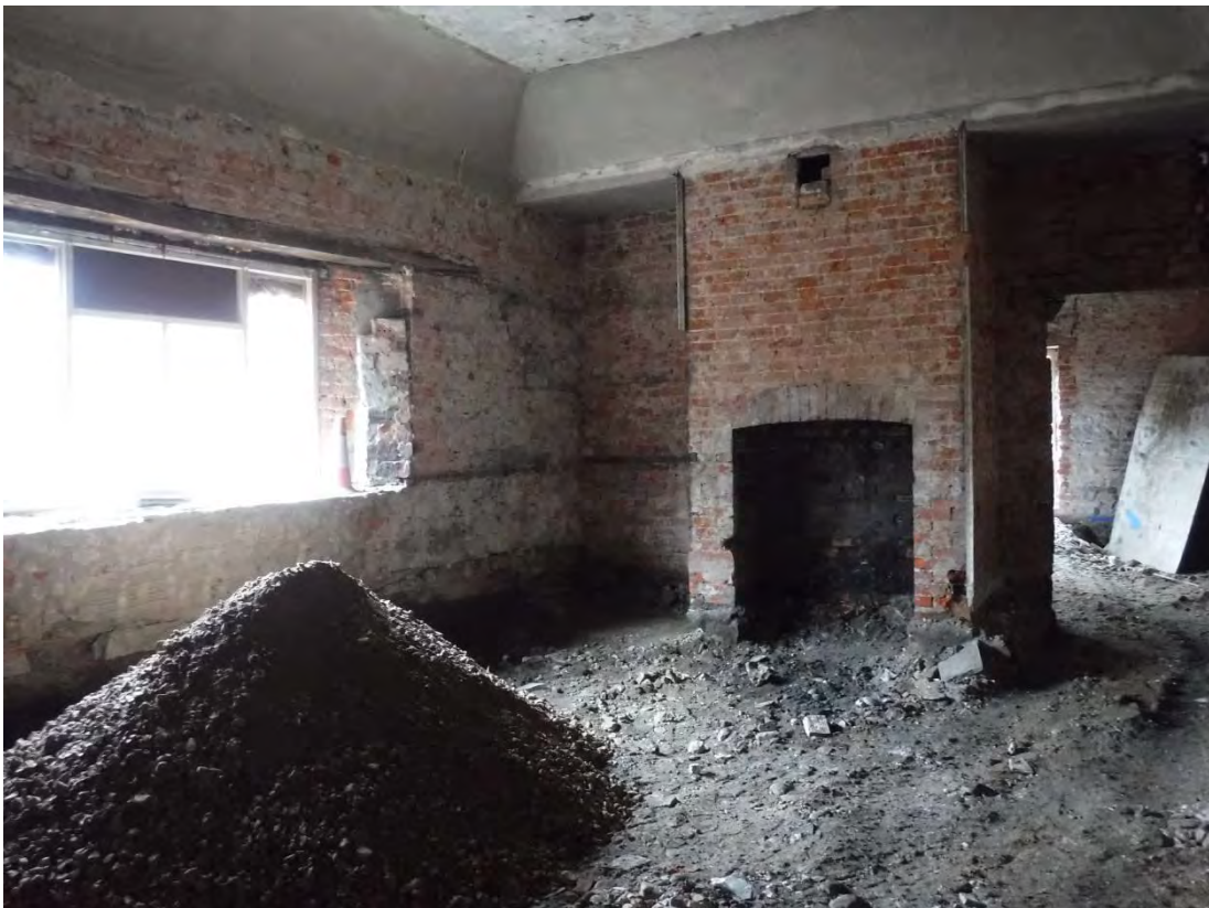
Photo 20: Laundry Building, Room 2. Shot facing ENE, showing deposit (176) and eastern wall.
