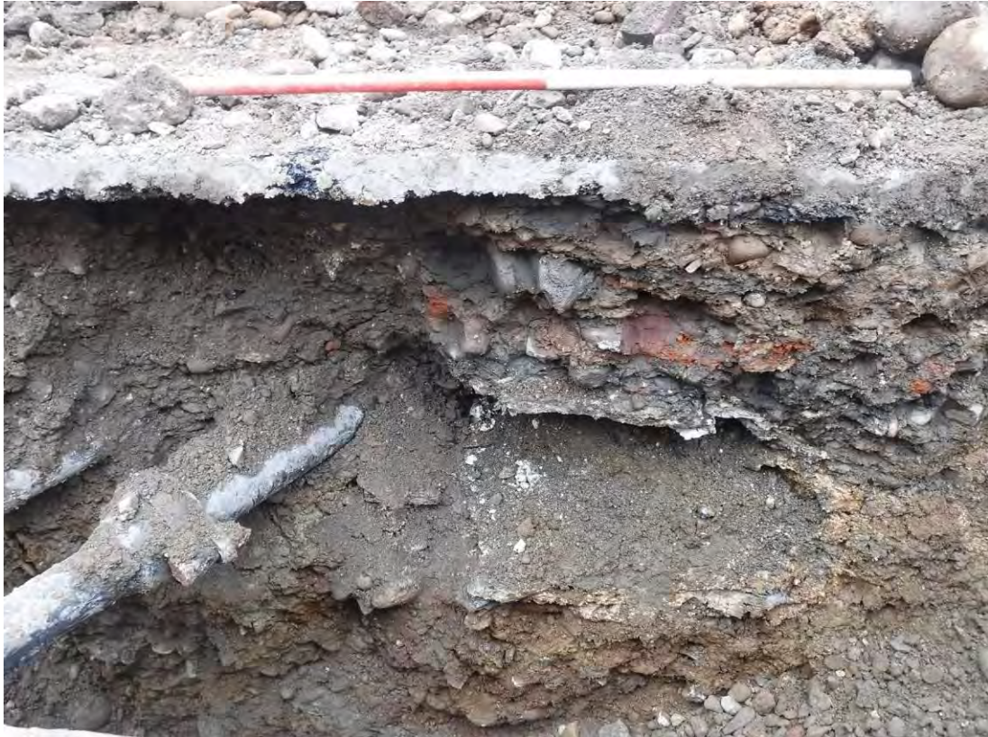
Photo 13: Trench 2, shot facing southeast showing the possible stone drain/culvert 116, and modern services. 1m scale.
