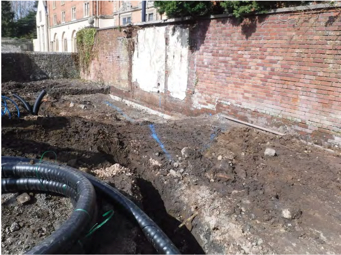
Photo 43: Trenches 4a, 4b and 7 under excavation. Shot facing southwest.
