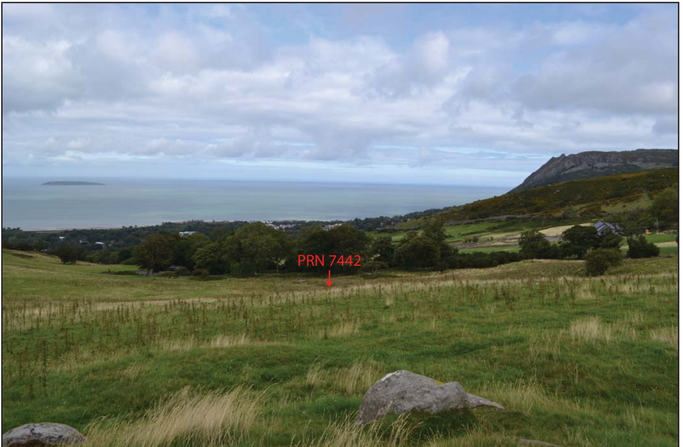
Plate 08: Viewpoint 4, view N from the Cae'r Haidd Deserted Rural Settlement Scheduled Monument (CN330) over the terraced fields (GAT HER PRN 7443) towards the proposed development, the broadly contemporary rectangular building (GAT HER PRN 7442) and Llanfairfechan, viewed from the N (archive ref: G2783_HASIA_004).
