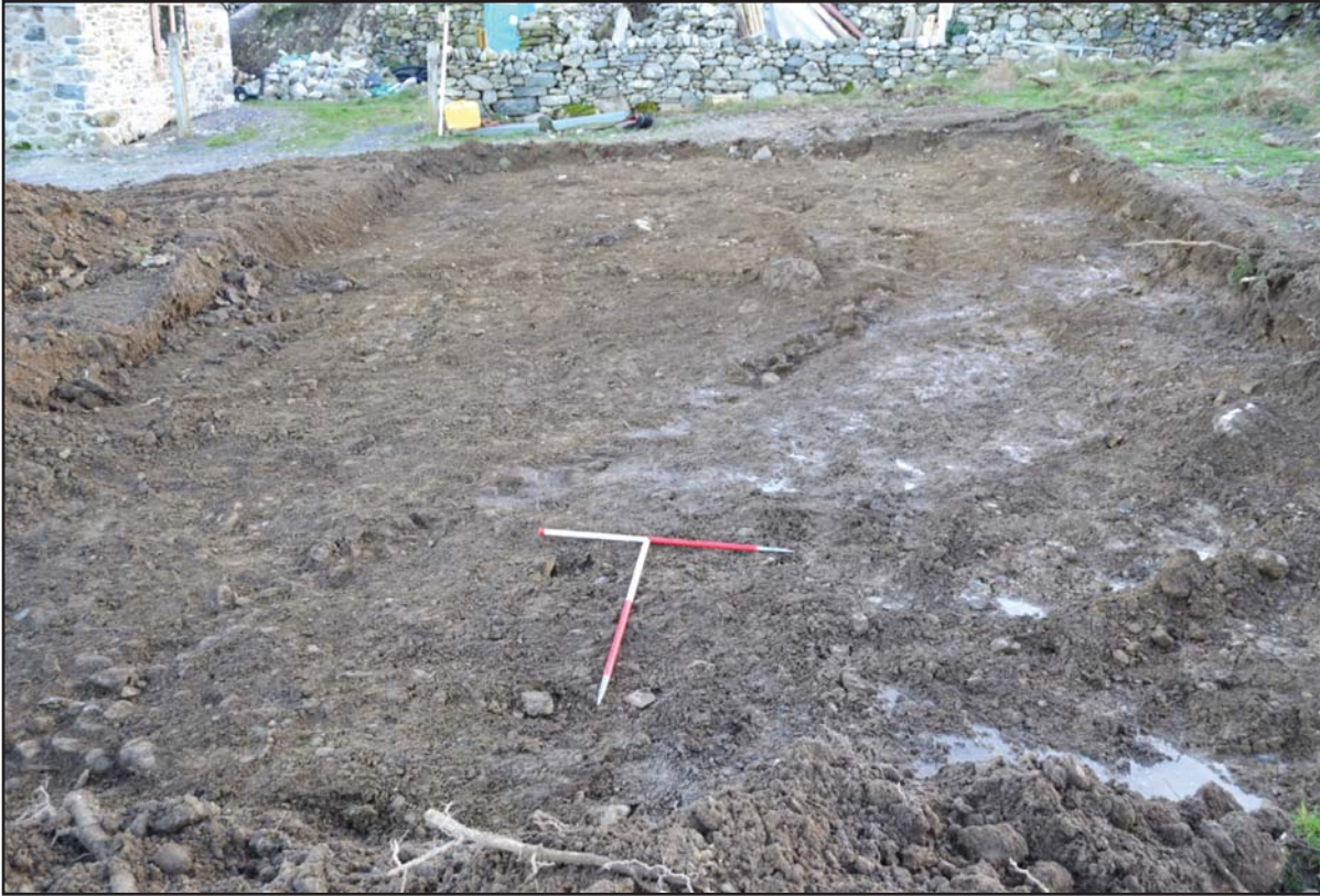
Plate 3: Area stripped showing land drain; from W (archive reference: G2783_032).
