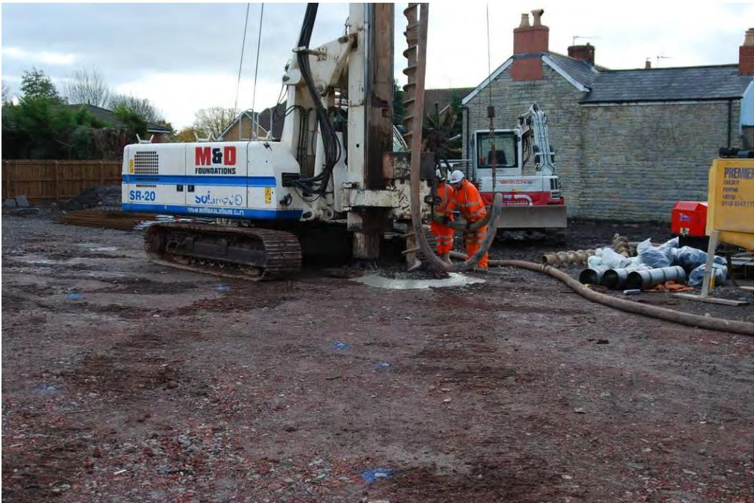
Photo 12: Foundation piling underway.
