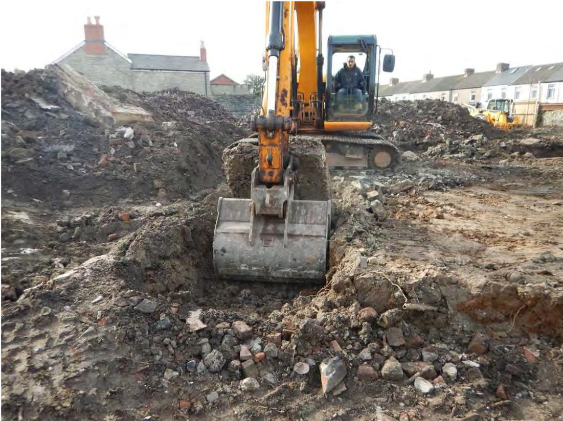
Photo 9: Concrete foundation of wall {009/016} during removal, looking north.
