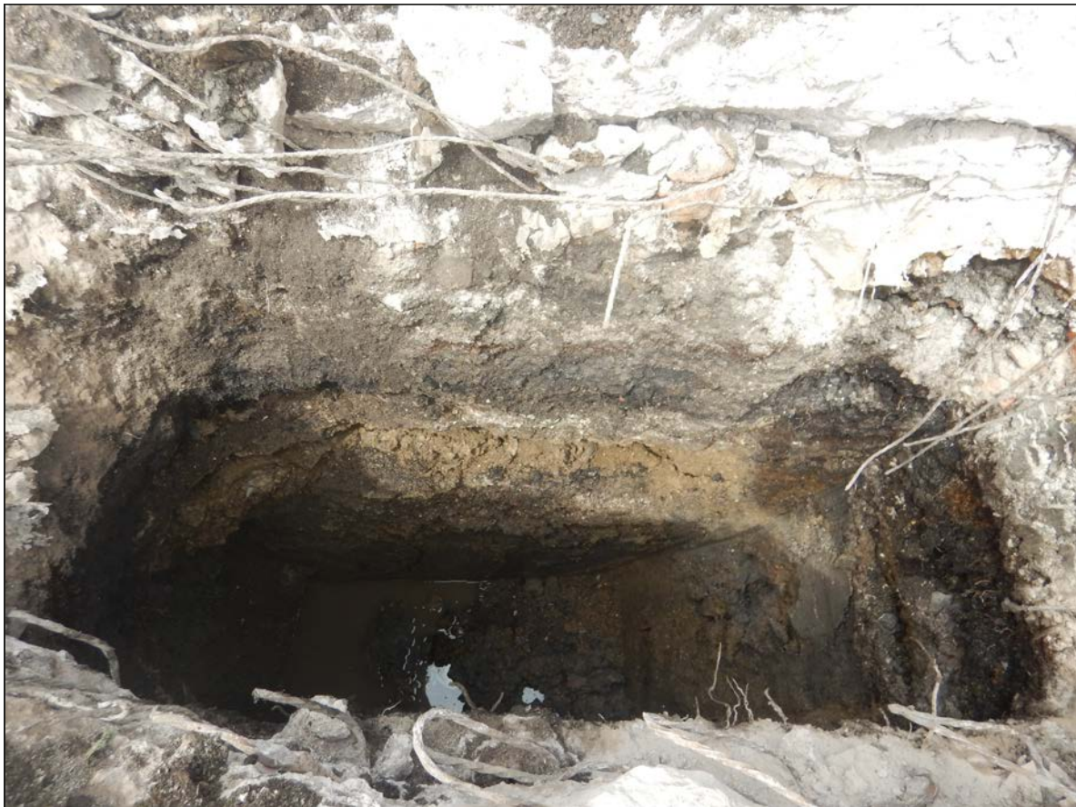
Plate11. TP 9 after excavation
