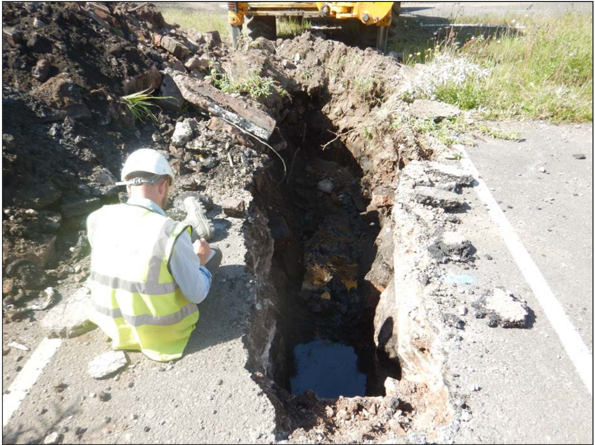
Plate 3. T2 during excavation
