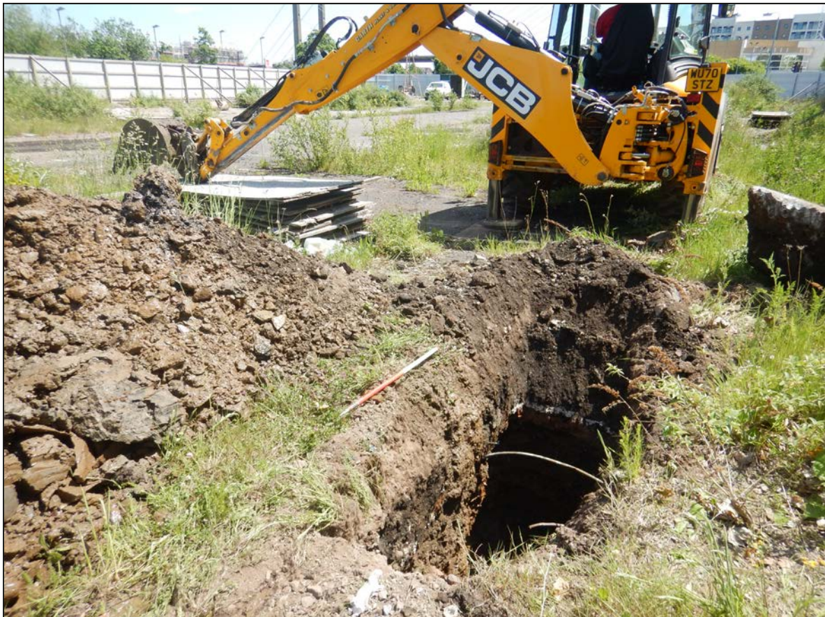
Plate 6. TP 4 during excavation
