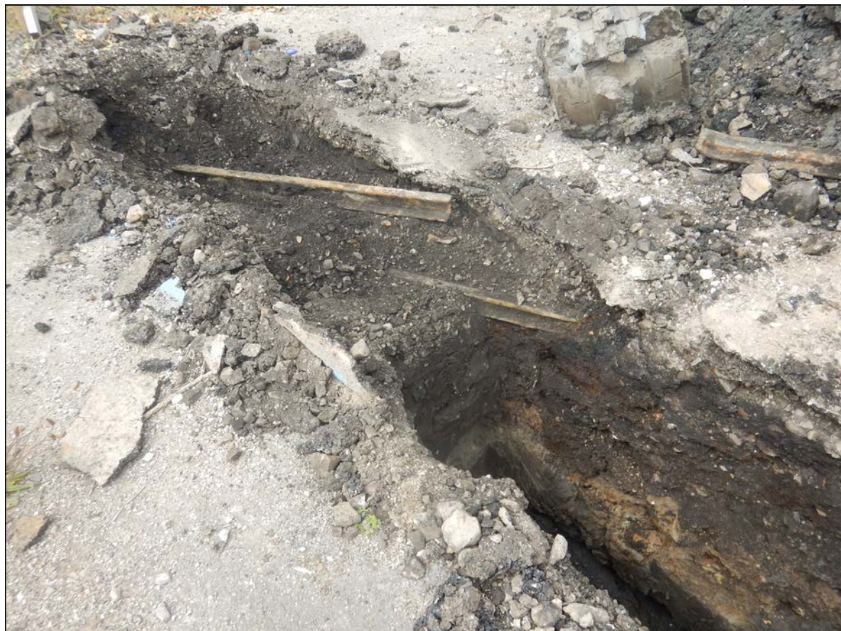
Plate 12. TP 8 SE facing section, oblique
