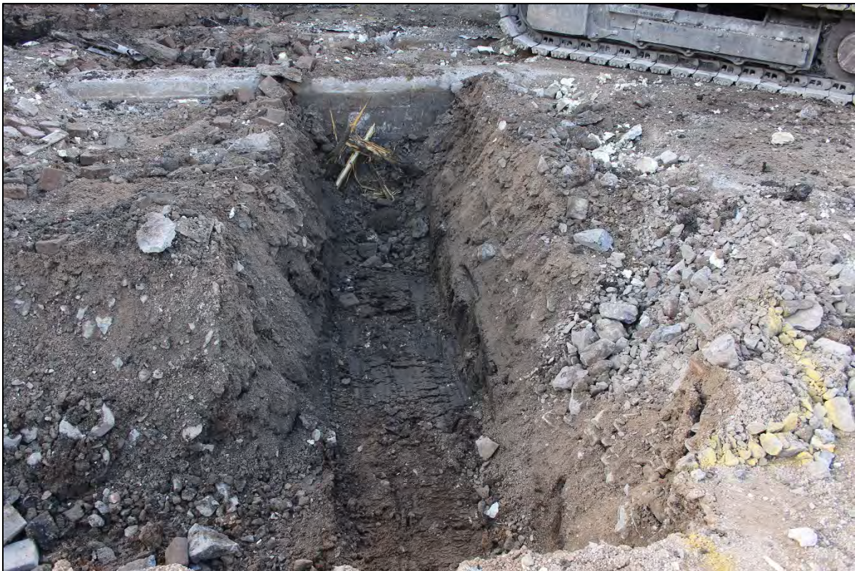
Plate 2: Footing 2 fully excavated, looking NW.
