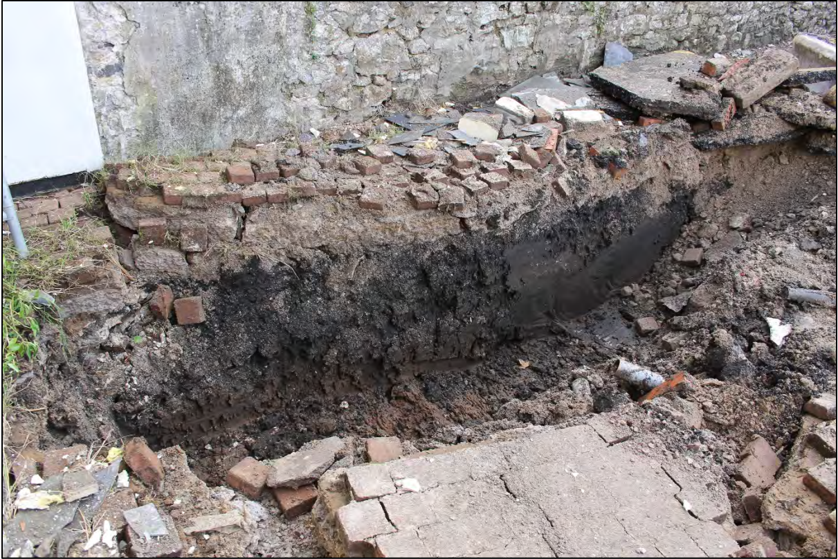
Plate 3: Footing 3, fully excavated, Looking NW.
