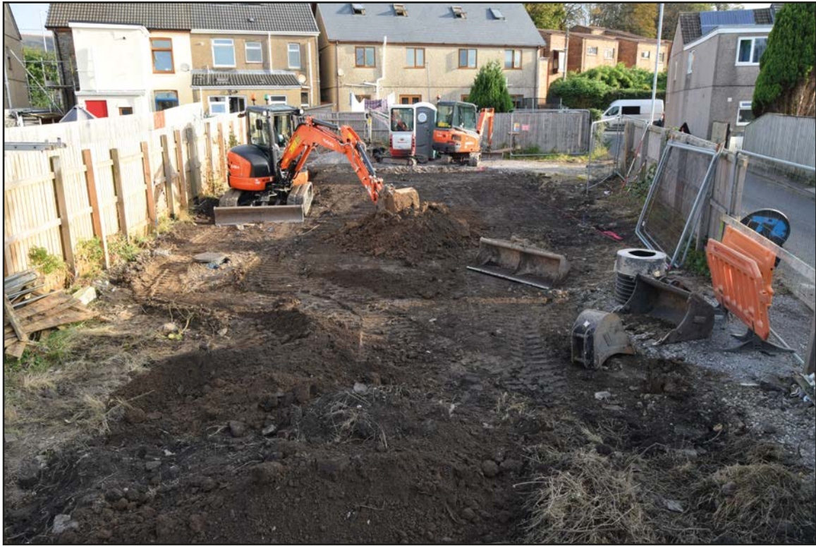
1. Working shot looking N.
