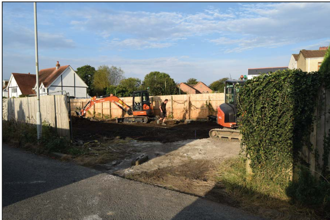
2. Working shot looking SW.
