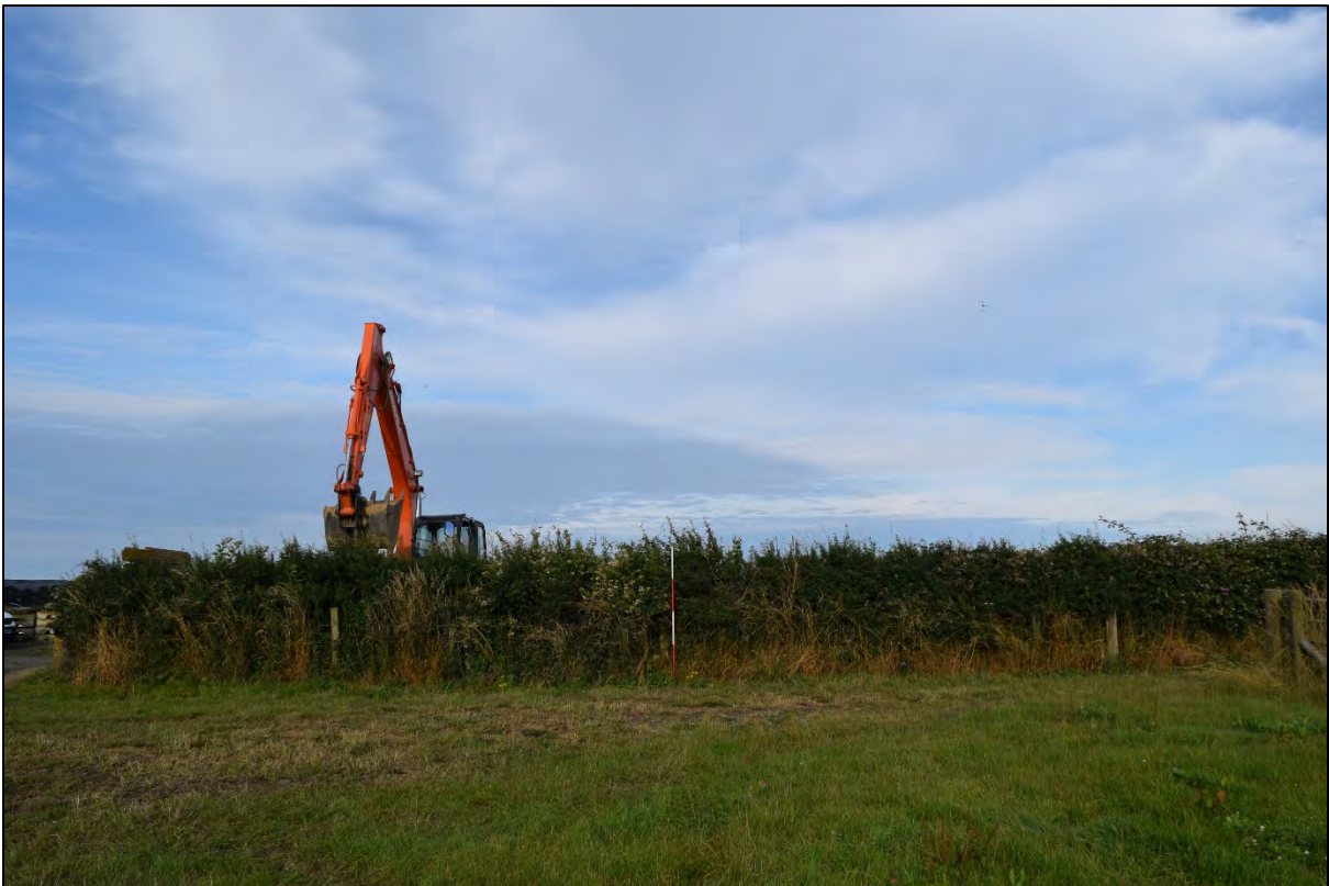
Plate 2: View of hedge bank prior to removal, looking W, 2m scale.
