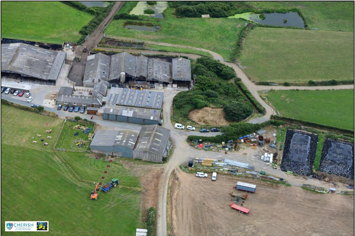
Plate 1: Aerial Photograph of Pointz Castle Farm during the groundworks
