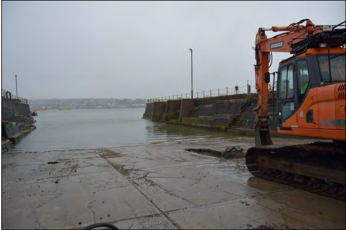
Plate 3: Slipway 1, view to the NNE.
