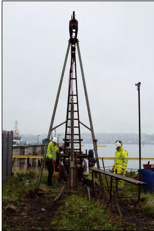
Plate 7: BH101 drilling rig in action, view to the north.
