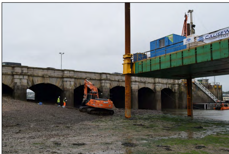
Plate 40: STP403 working shot, view to the west.
