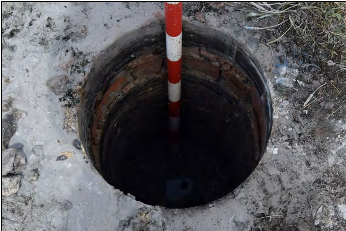
Plate 10: BH105 showing brickwork (1052) and lower concrete layer (1053) below, 0.5m scale.
