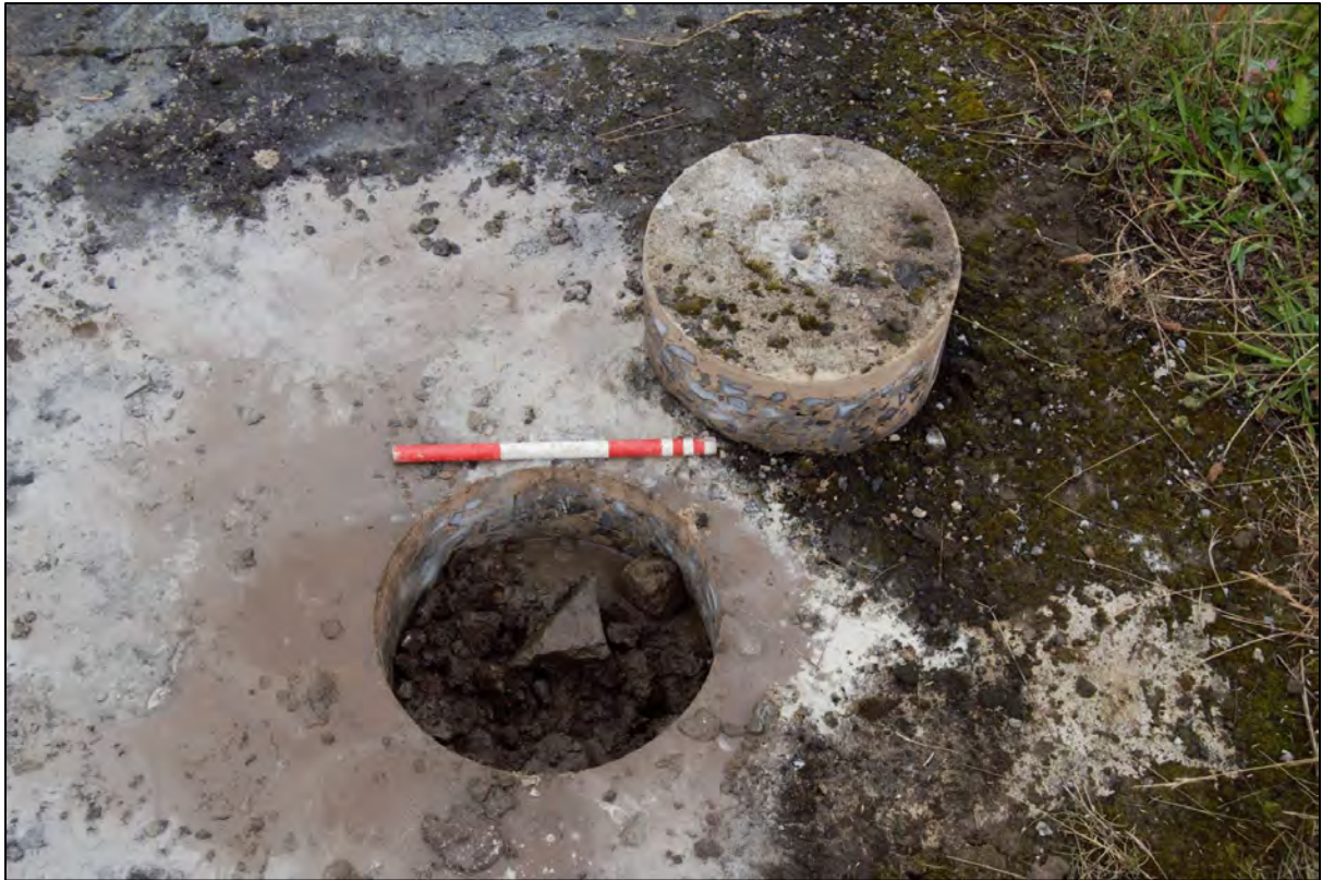
Plate 11: BH107, concrete (1071) removed to reveal hard core layer (1072), 0.3m scale.
