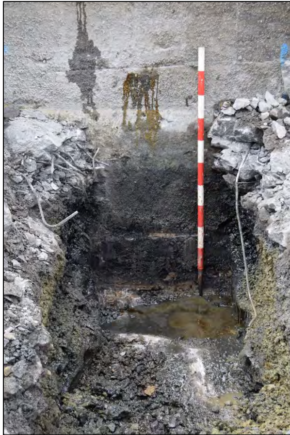
Plate 15: STP204 the base of east face of the western wall of Slipway 1, view to the west, 1m scale.
