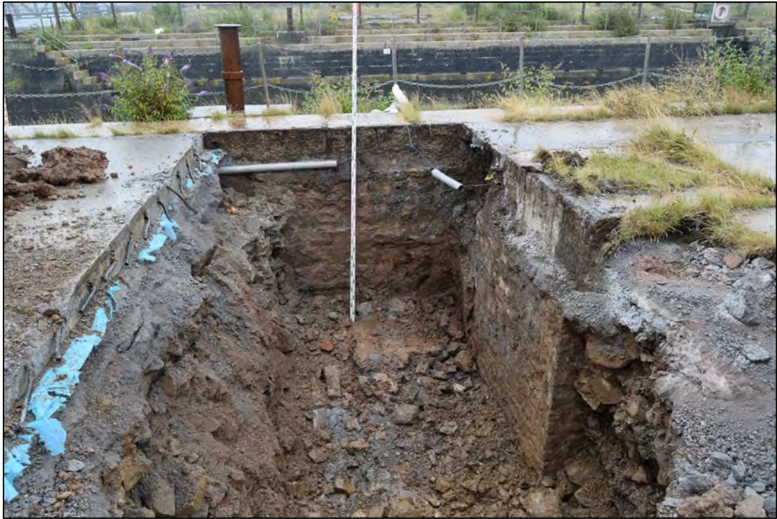
Plate 45: CPWIT East, west face of western wall of Slipway 2 and plinth [6005], view to the east, 4m scale.
