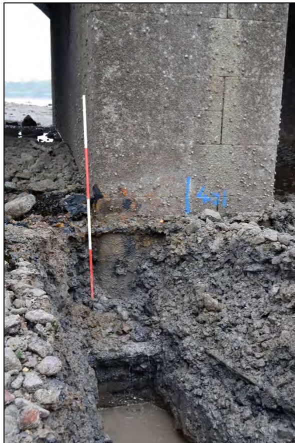
Plate 36: STP401 east facing section, showing Carr jetty arch supports, view to the west, 2m scale.
