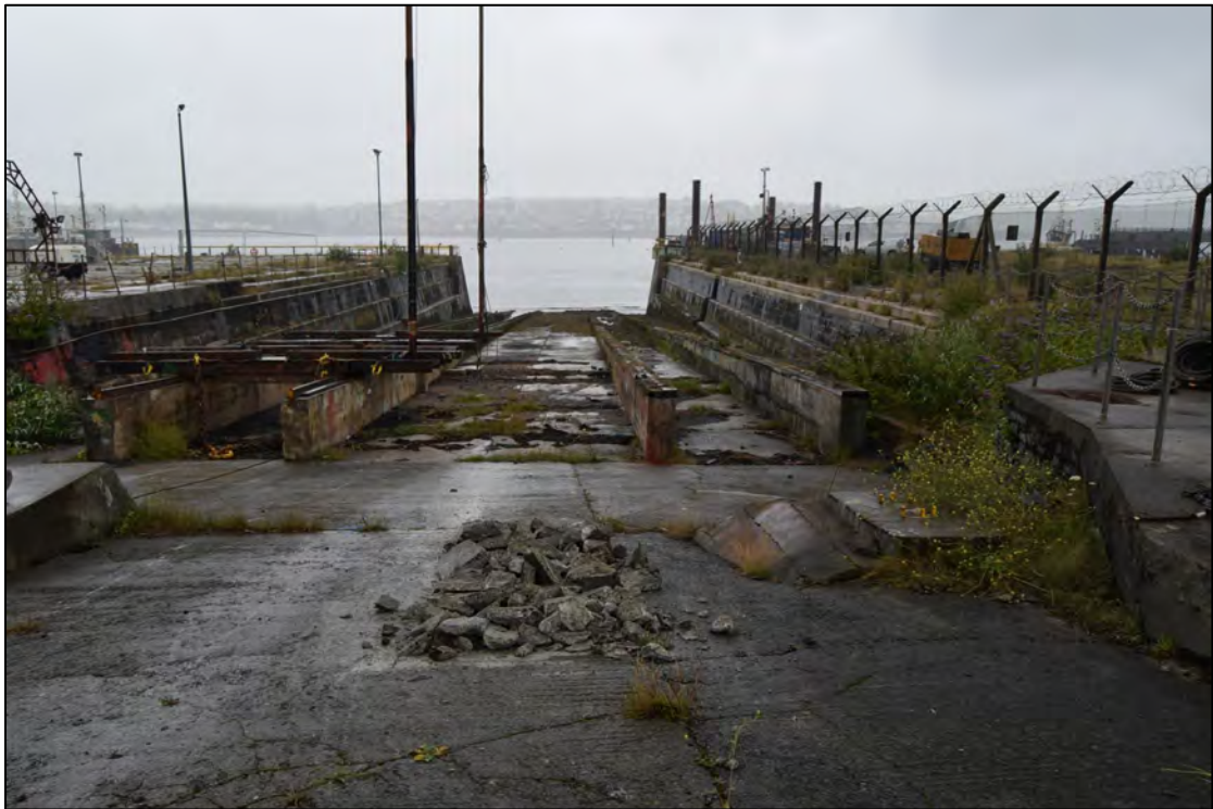
Plate 4: Slipway 2, View to the N.
