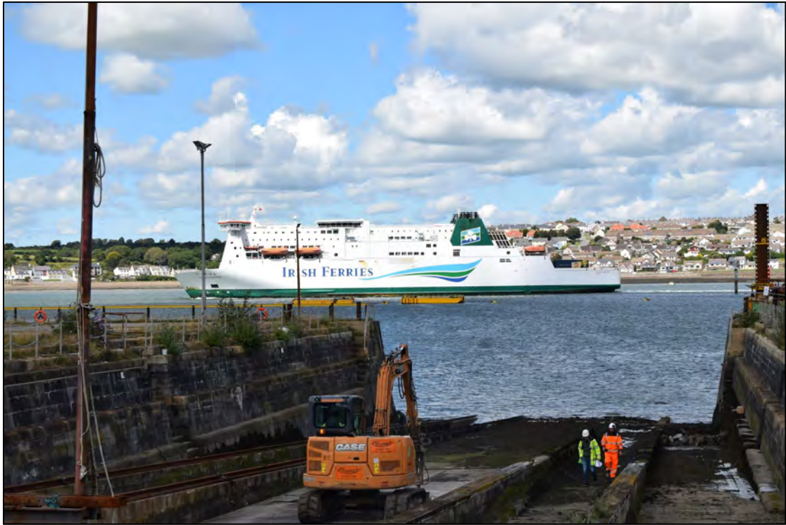
Plate 1: Historic Building Slip Number 1, view to NNW.
