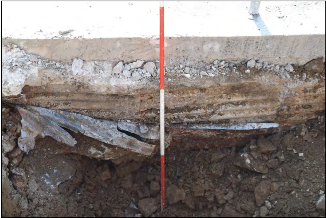
Plate 13: STP202 west face of Slipway 1 western wall [2025] and corrugated iron shuttering (2027), view to east, 2m scale.
