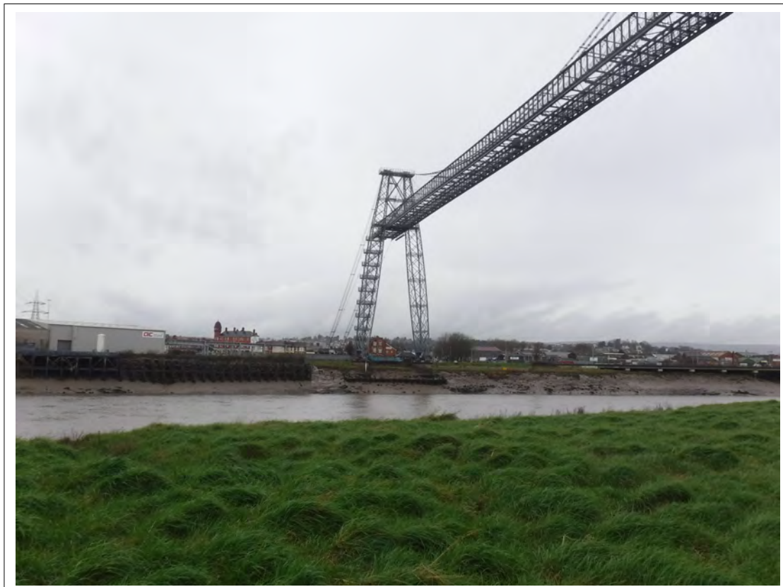
Plate 12. View of Transporter Bridge from western side of River Usk
