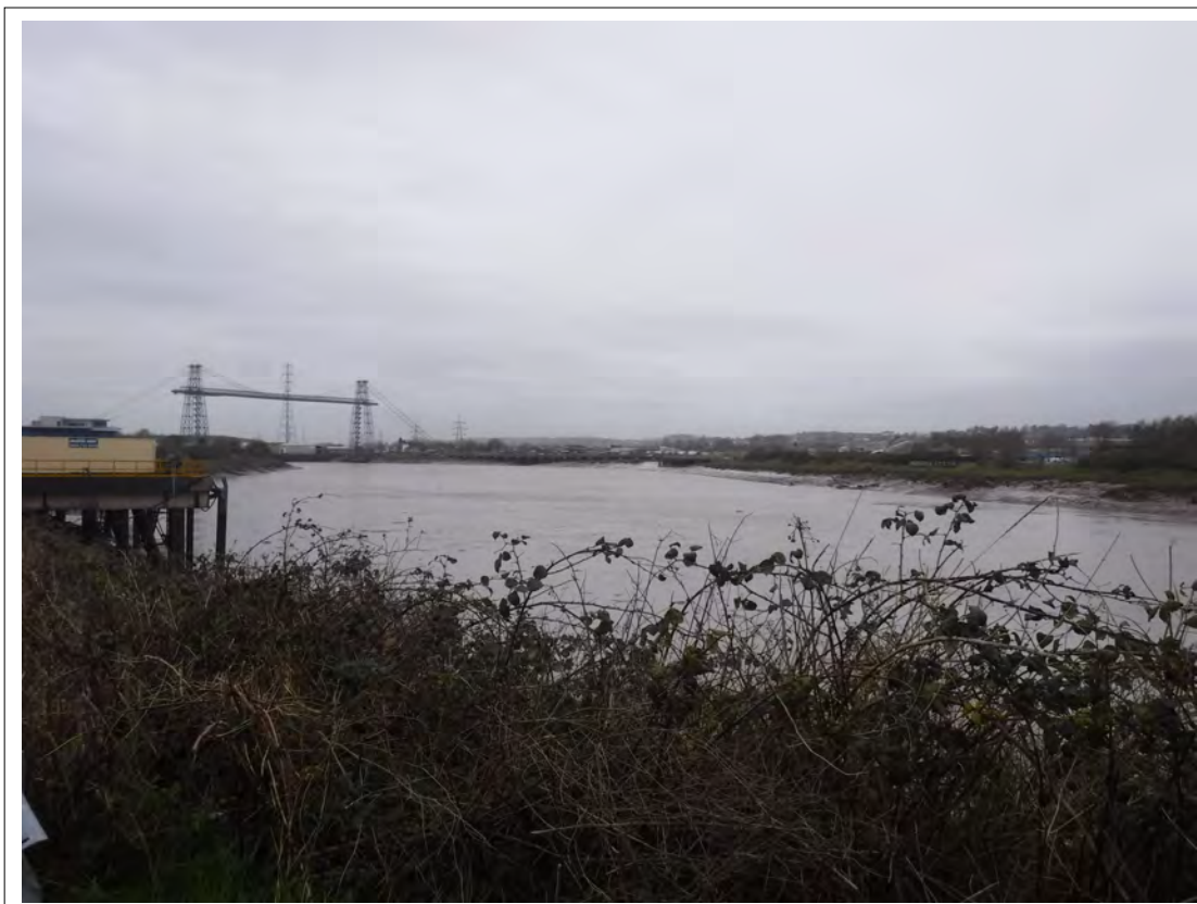
Plate 11. View of Transporter Bridge from western bank, looking NE
