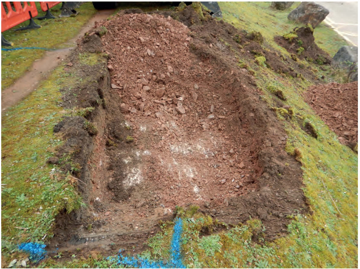
Plate 5 Extent of excavation TP006. West facing.
