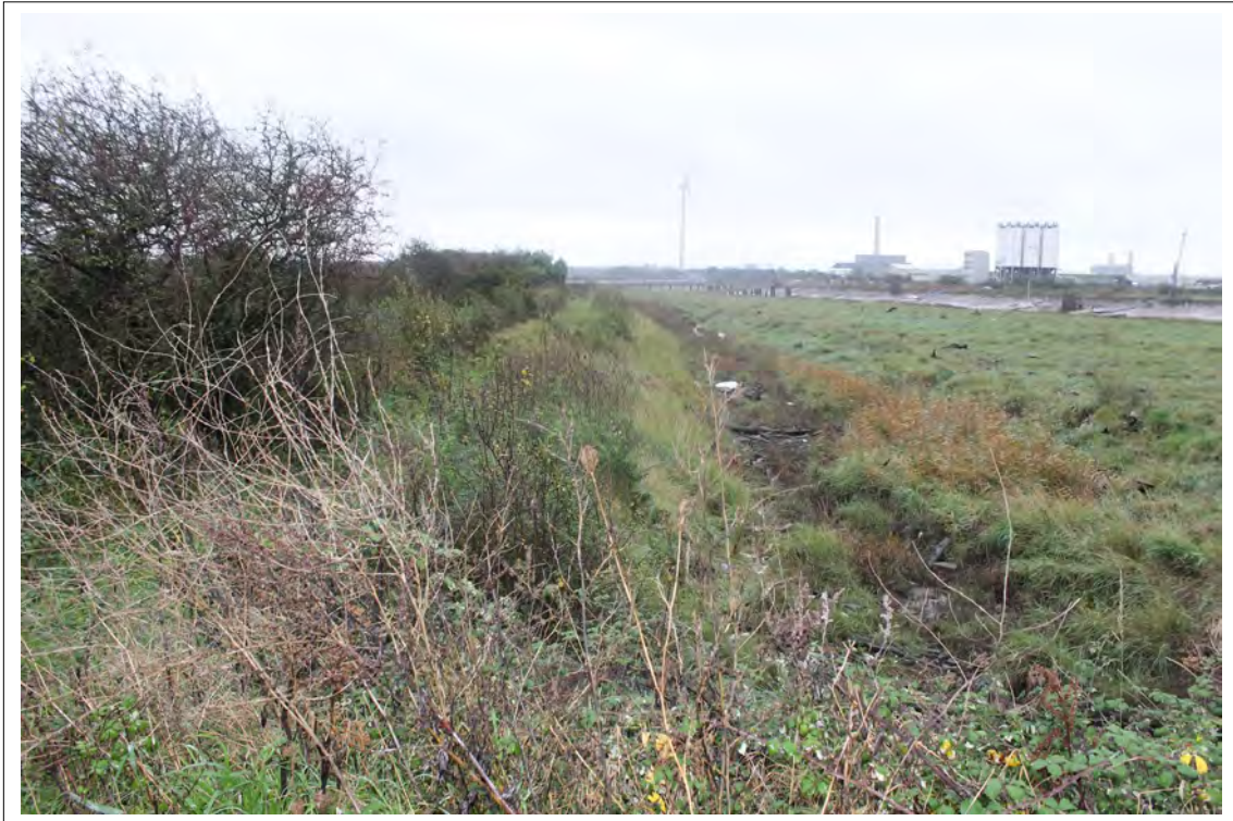
Plate 9. View to the south showing the line of the existing flood defences.
