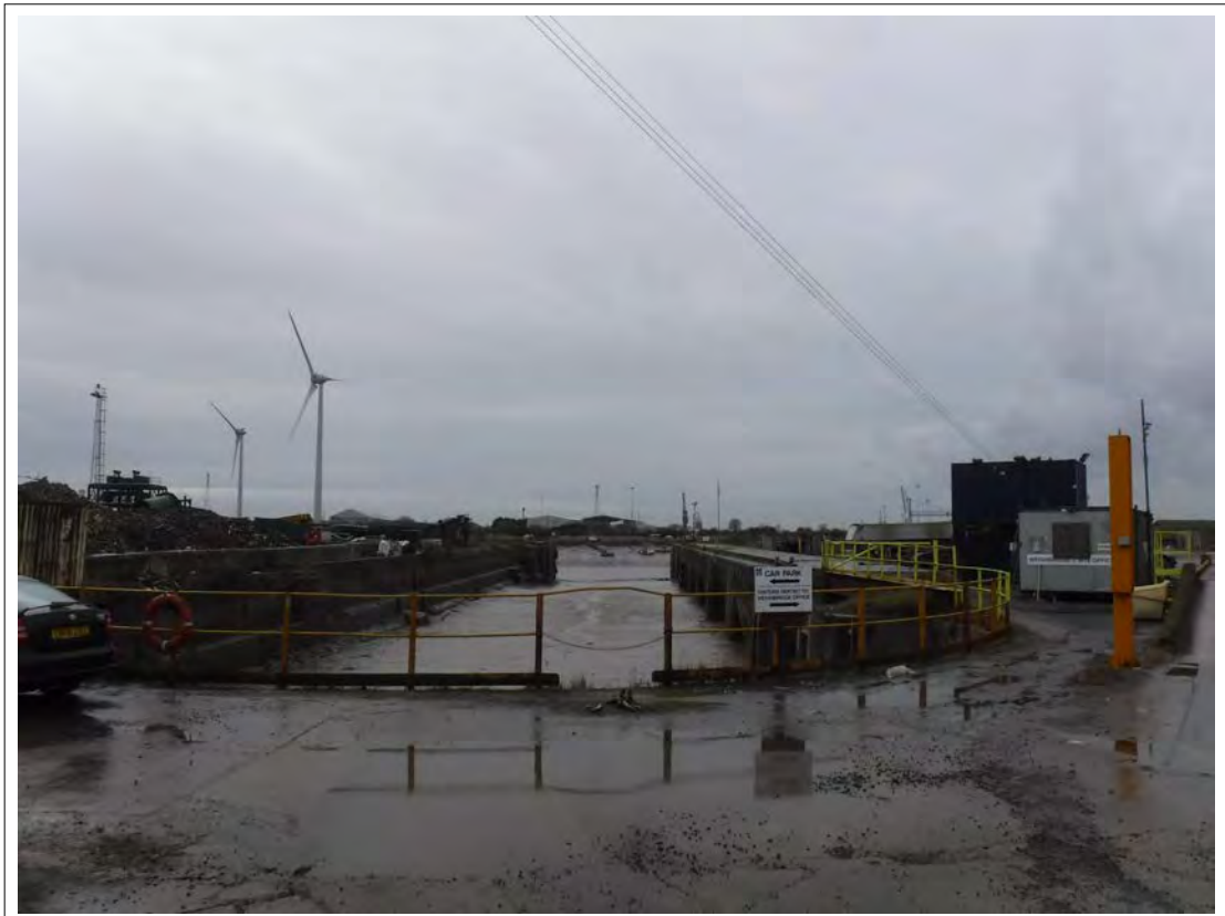
Plate 5. Southern section, view of dry dock, looking SW
