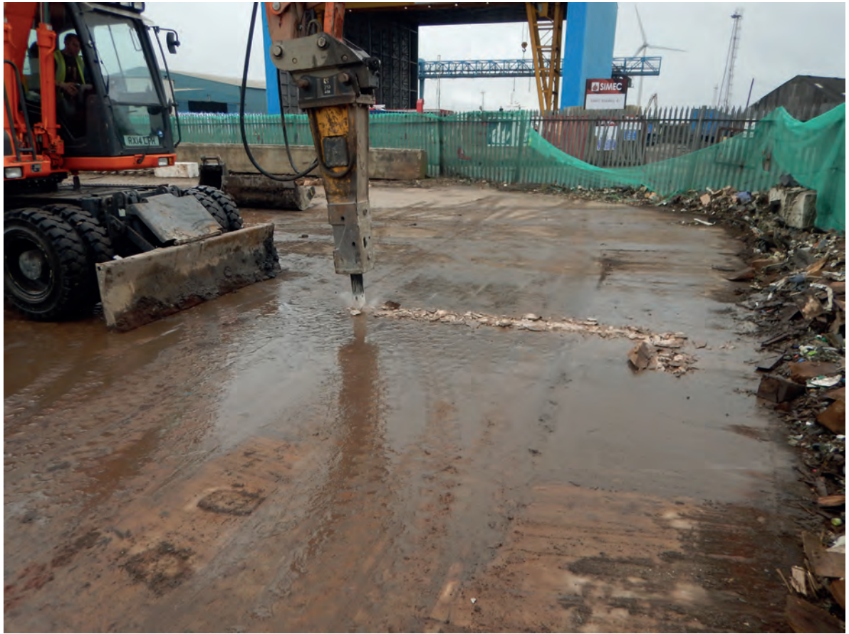
Plate 1 Working shot of 16-tonne excavator and hydraulic pecker. South facing.
