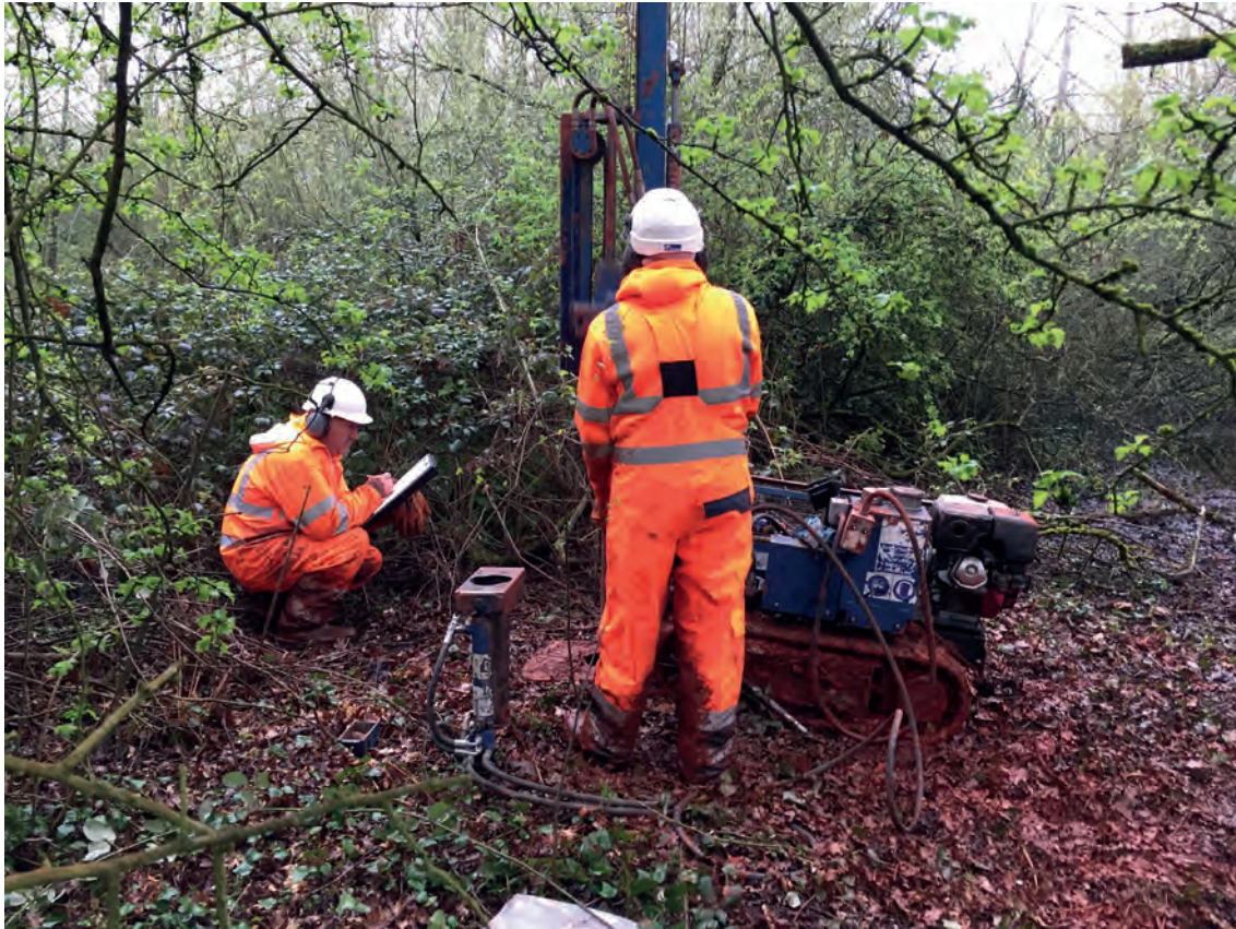
Plate 3 Working shot of dynamic probe drilling taking place. South facing.
