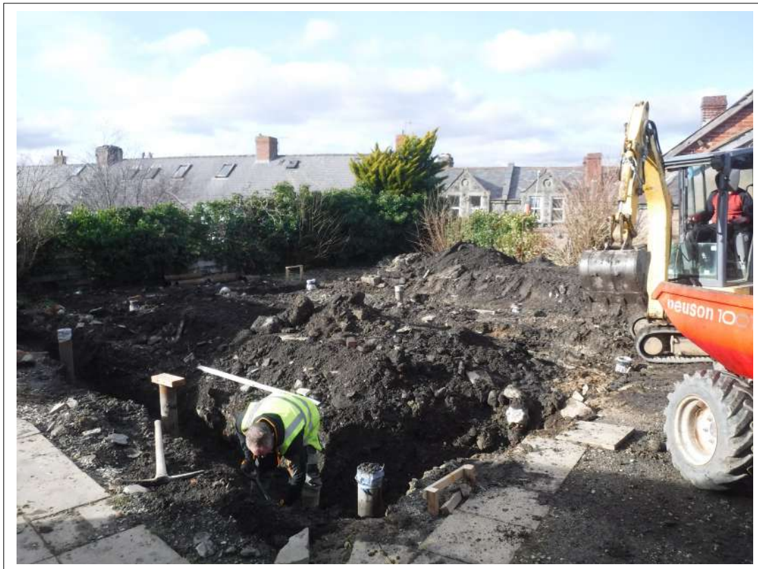
Plate 1. East facing view of trench being excavated (with metal piles)
