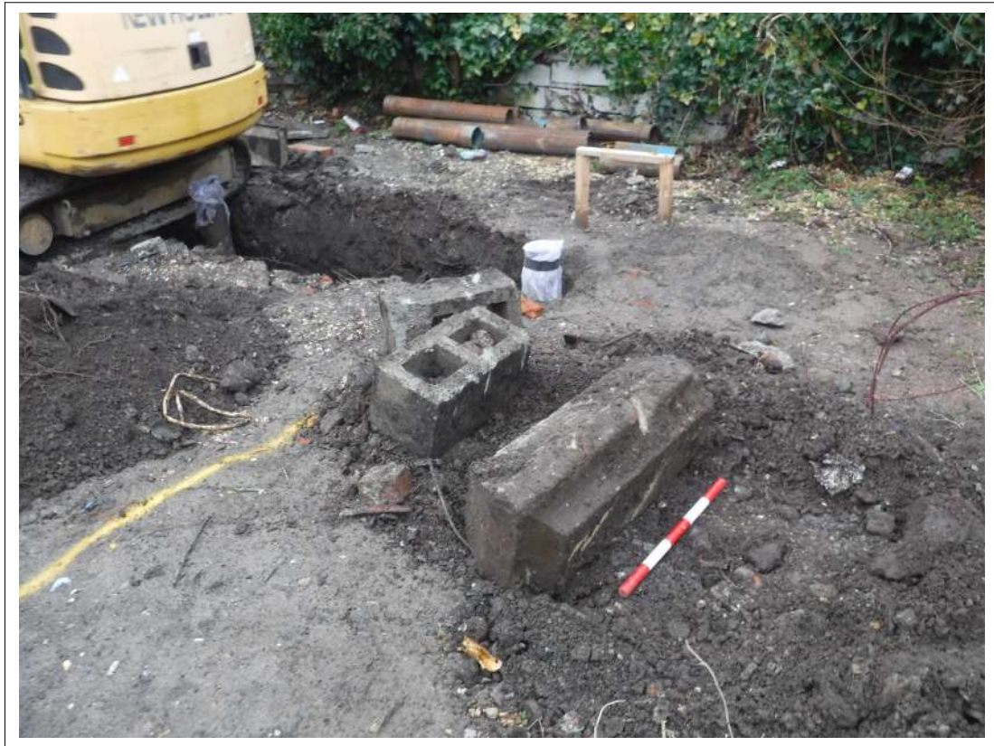
Plate 3. South East view of worked stone with bevelled edges
