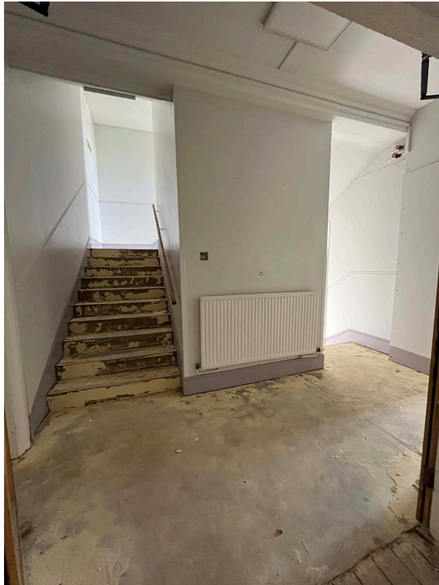
View of existing Stair
