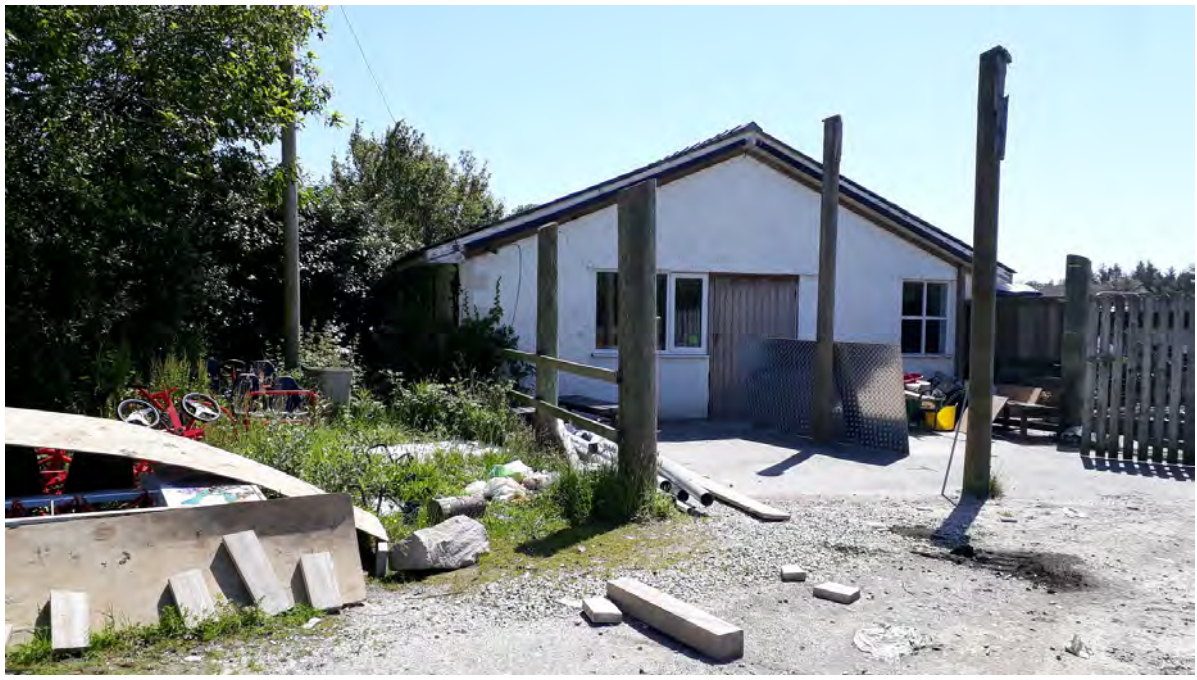
Plate 13. Disused shed on the eastern site boundary . View SE
