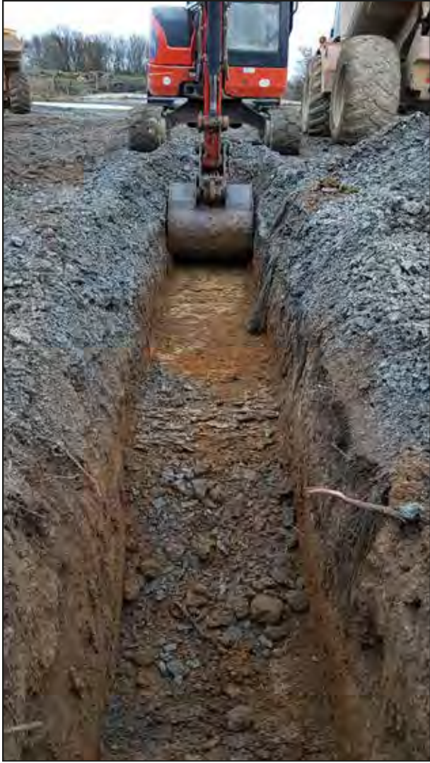
Plate 11. Trench 2, working shot, looking E.
