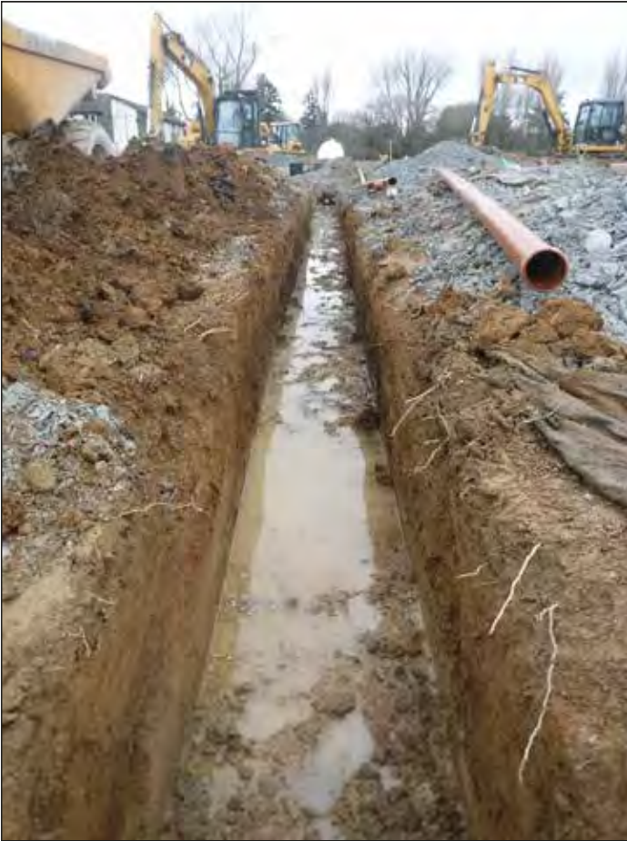
Plate 25. Trench 5, working shot looking W
