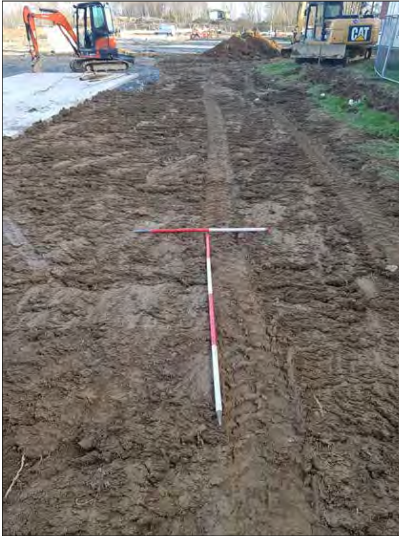
Plate 3. Topsoil strip, looking E.
