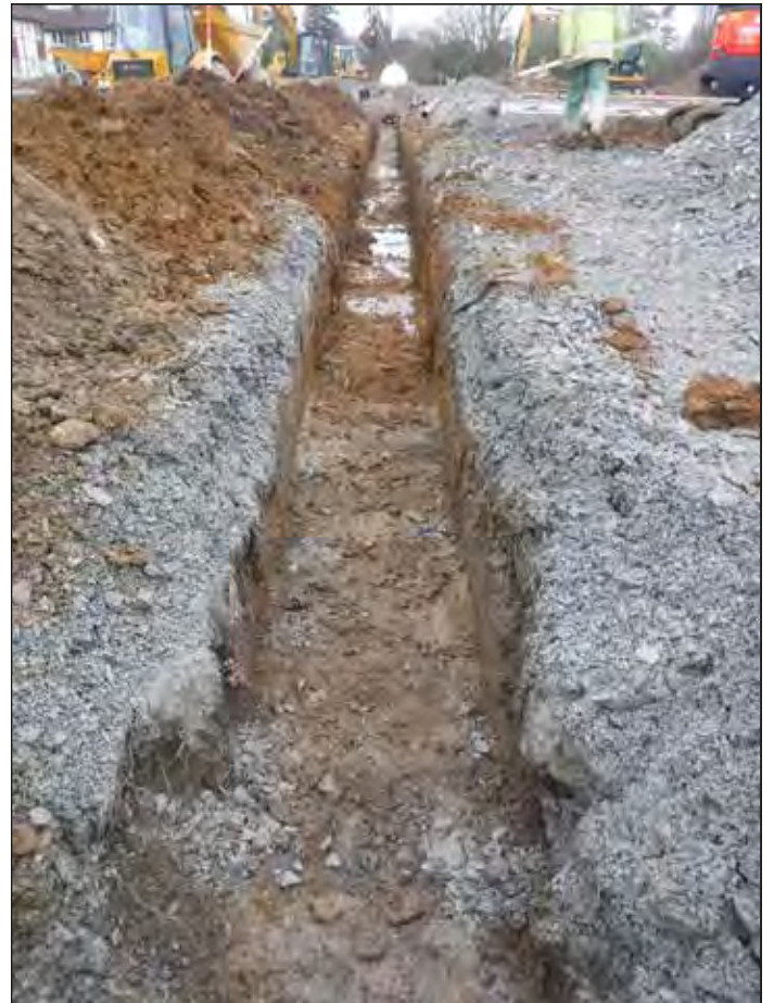
Plate 26. Trench 5, working shot looking W.
