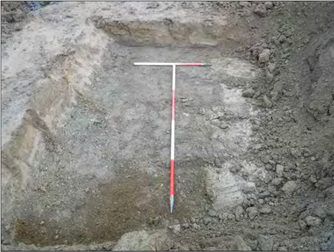
Plate 23. Working Shot of slot for pump looking S.
