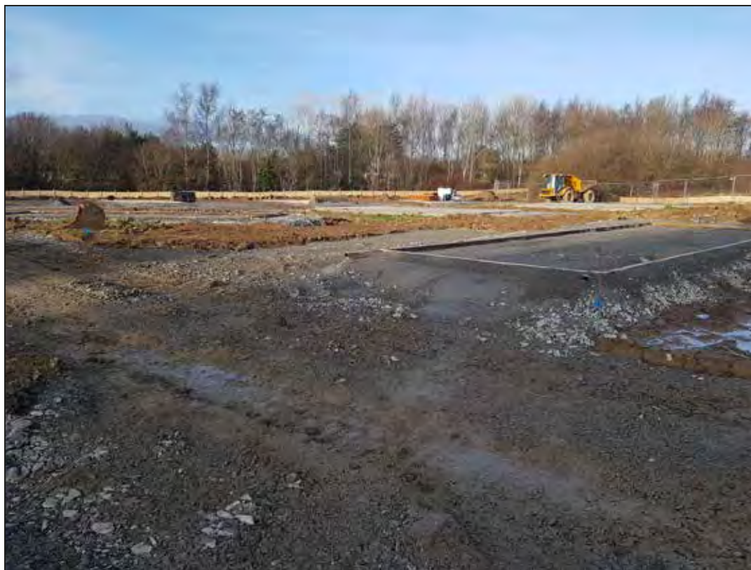
Plate 1. Watching Brief, working shot, looking NW.
