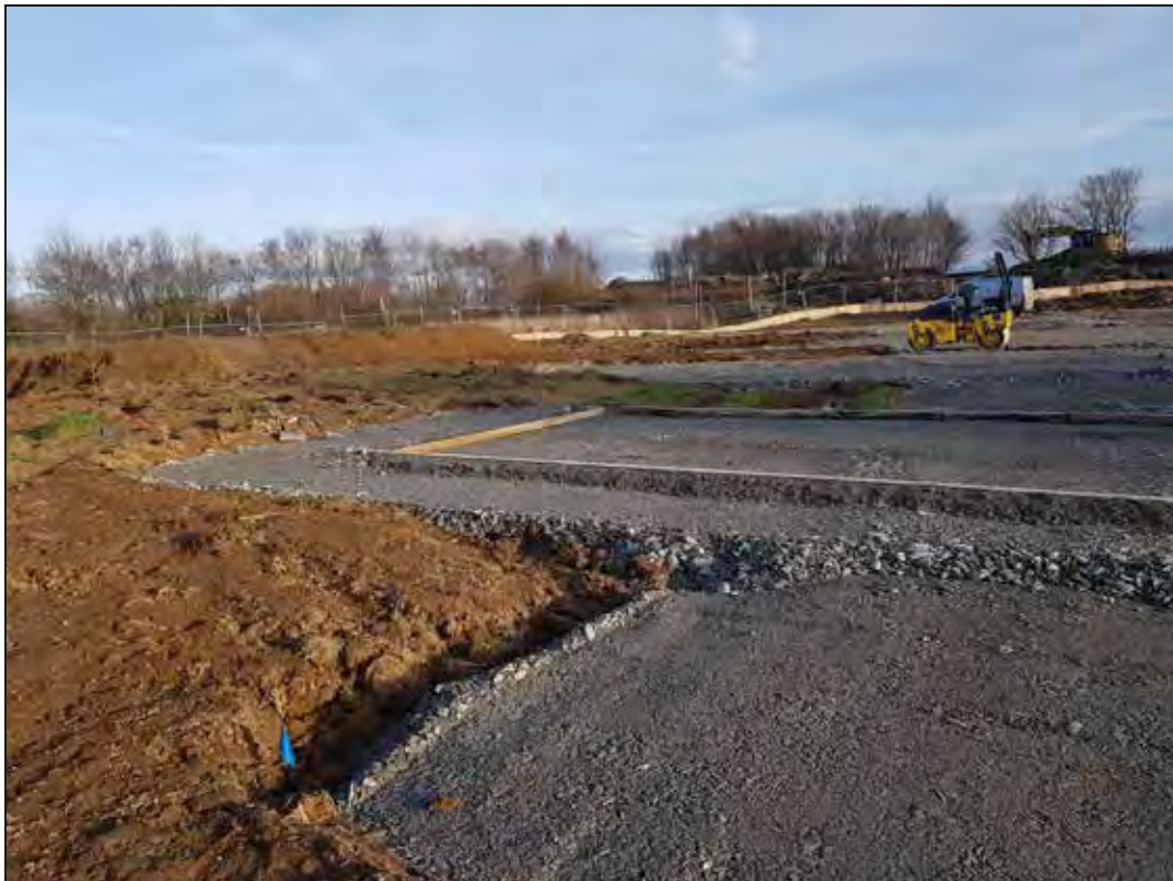
Plate 4. Watching Brief, working shot looking NE.
