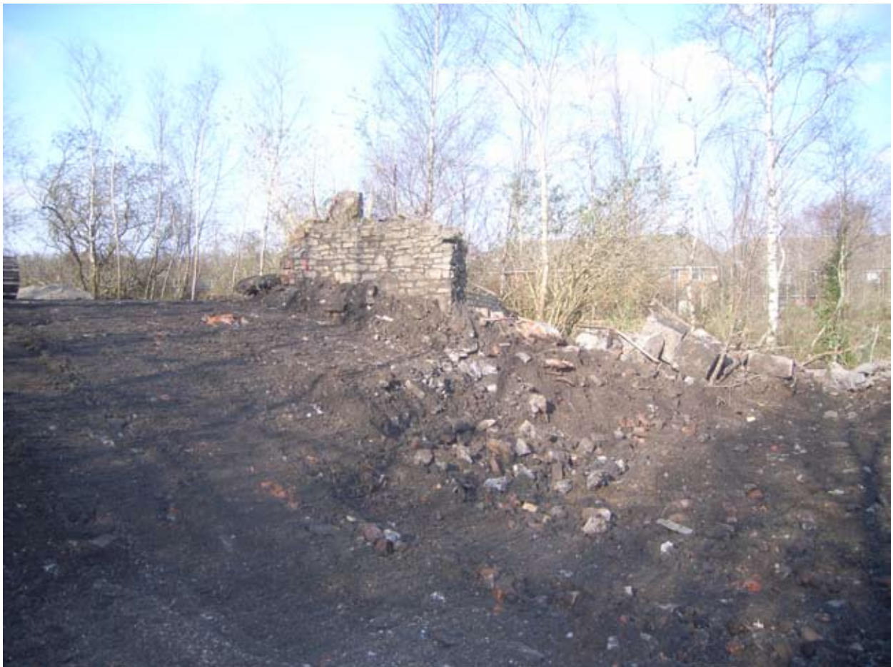
Plate 2: Wall 102 and soil bund
