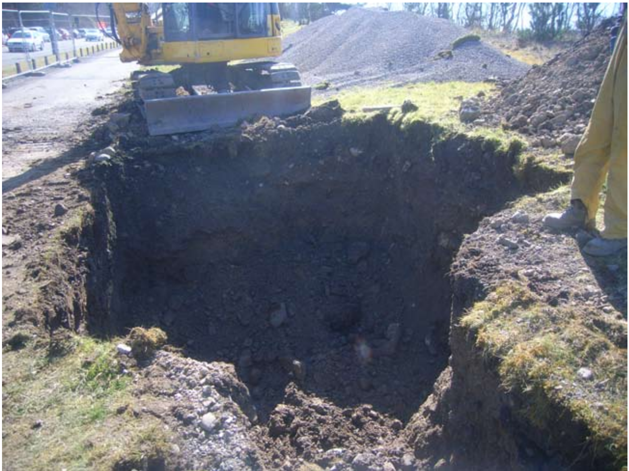
Plate 17: Excavation of access chamber adjacent to the A4217
