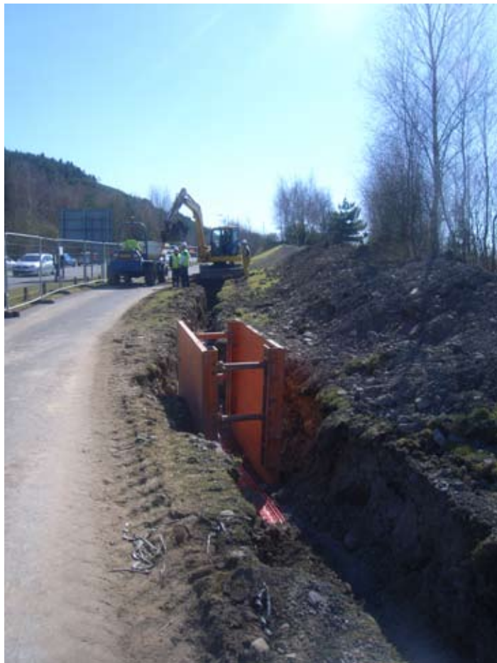
Plate 16: Pipe trench along the A4217
