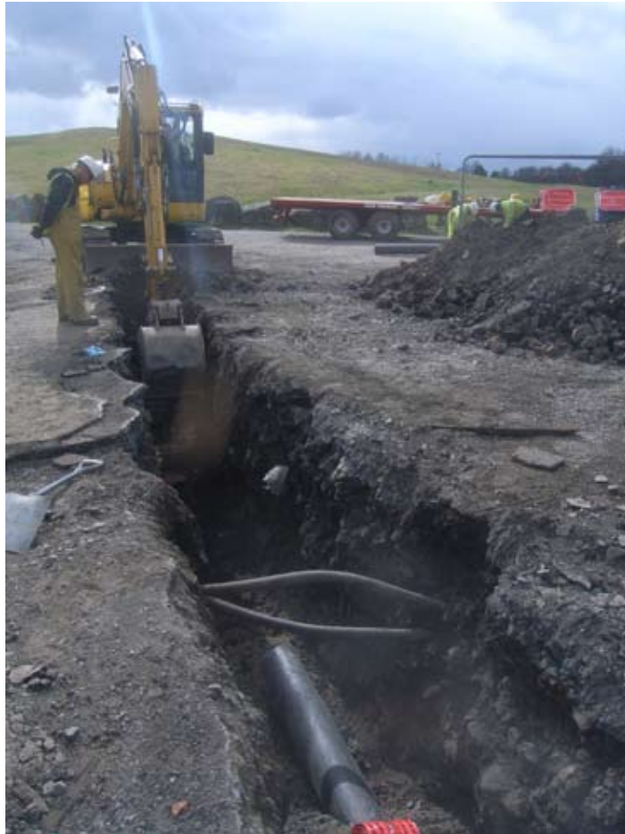
Plate 15: Pipe trench within White Rock car park
