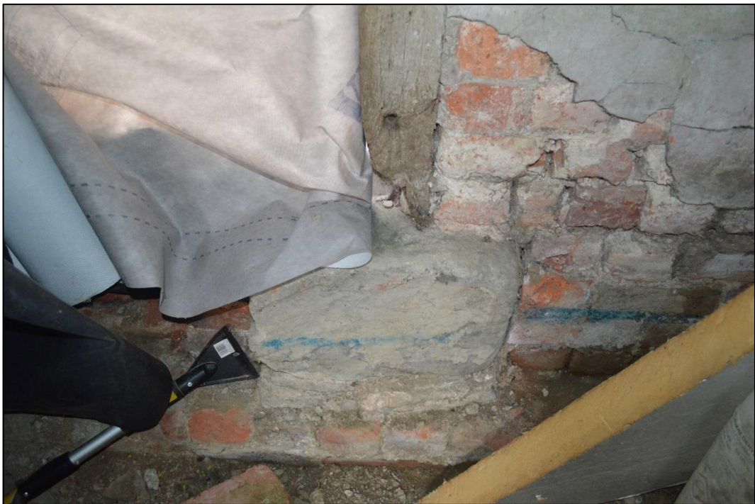
Figure 17: Base of external doorway into loose box. Facing south. CPAT 5046_0084
