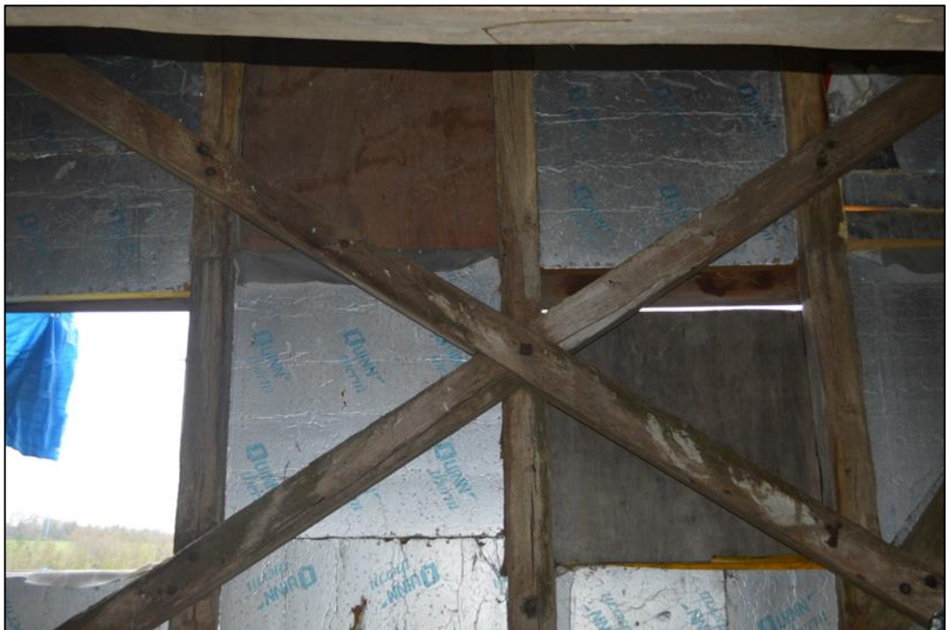
Figure 19: Cross beams on the north wall. CPAT 5046_0030
