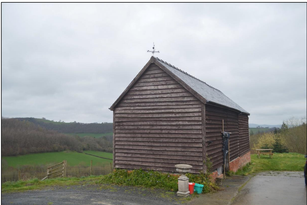
Figure 11: West gable of barn with south wall visible. Facing north east. CPAT 5046_0079
