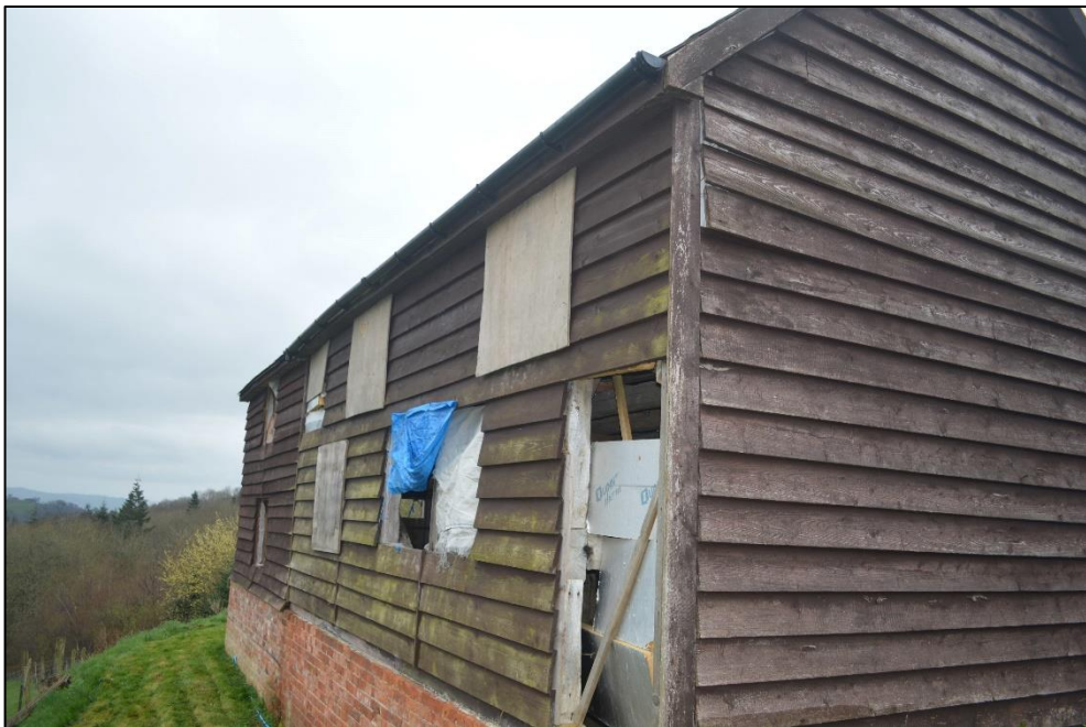
Figure 9: North wall of barn. Facing north east. CPAT 5046_0076
