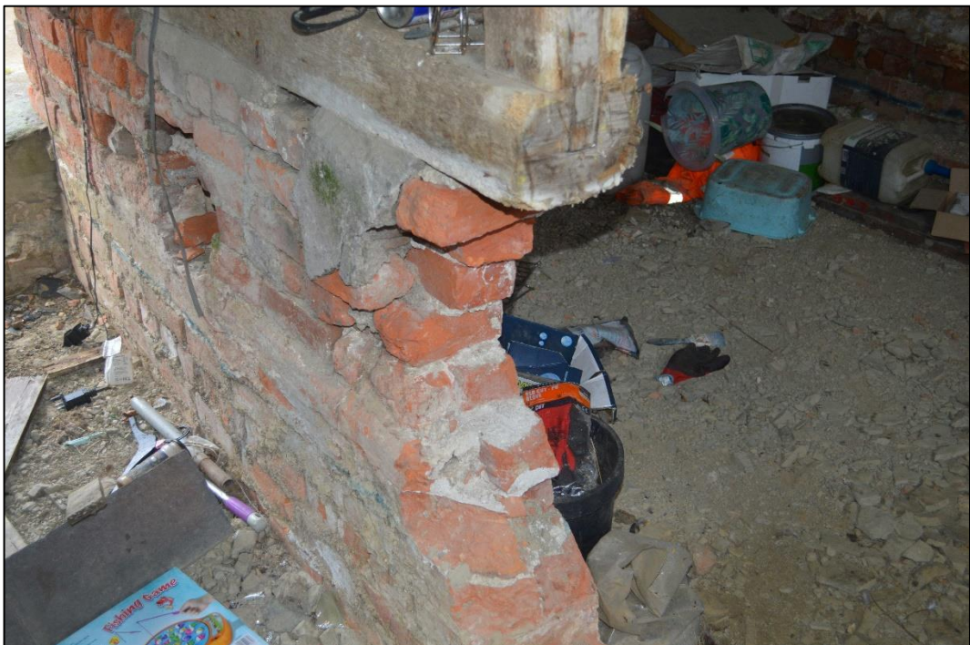
Figure 23: Brick plinth for wall partition with cut beam above. Facing south west. CPAT 5046_0086
