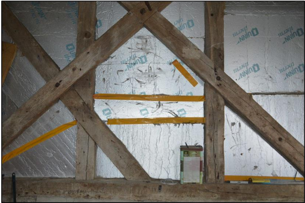
Figure 18: Cross beams on the south wall. Facing south. CPAT 5046_0006
