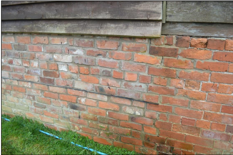
Figure 14: Modern brick plinth with damp proof membrane visible. Original brick coursing to the right. Facing south east. CPAT 5046_0067
