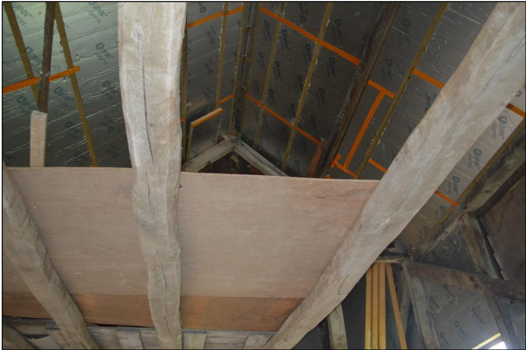
Figure 28: Hand cut beams of the hayloft. Facing west. CPAT 5046_0107
