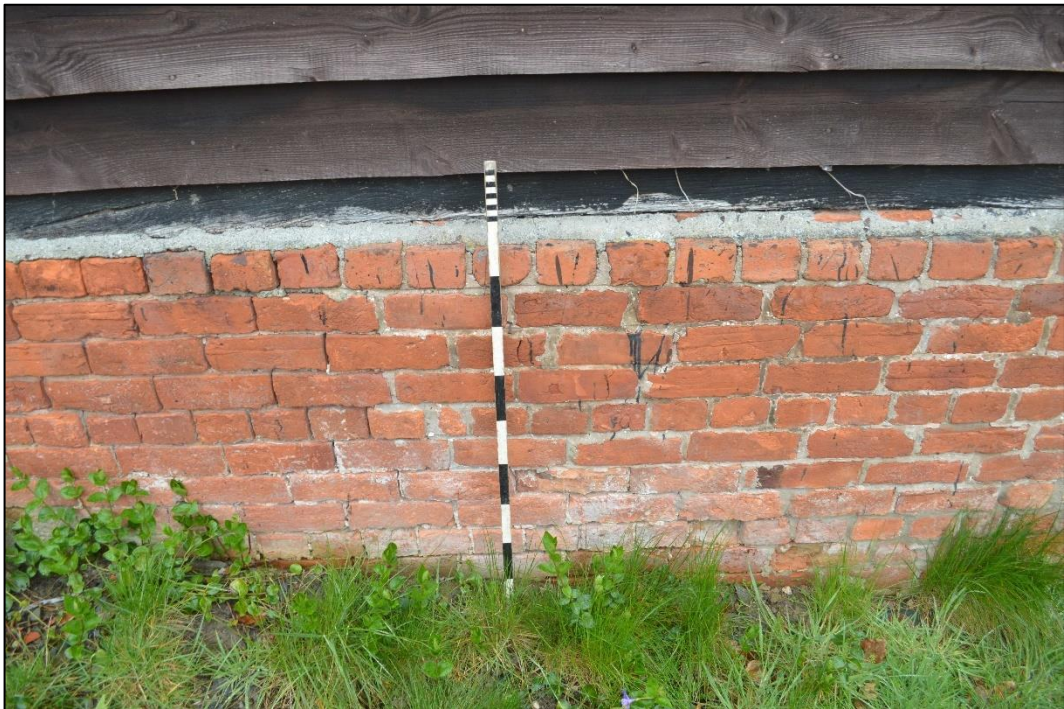
Figure 13: Brick foundation plinth. Facing north. CPAT 5046_0064
