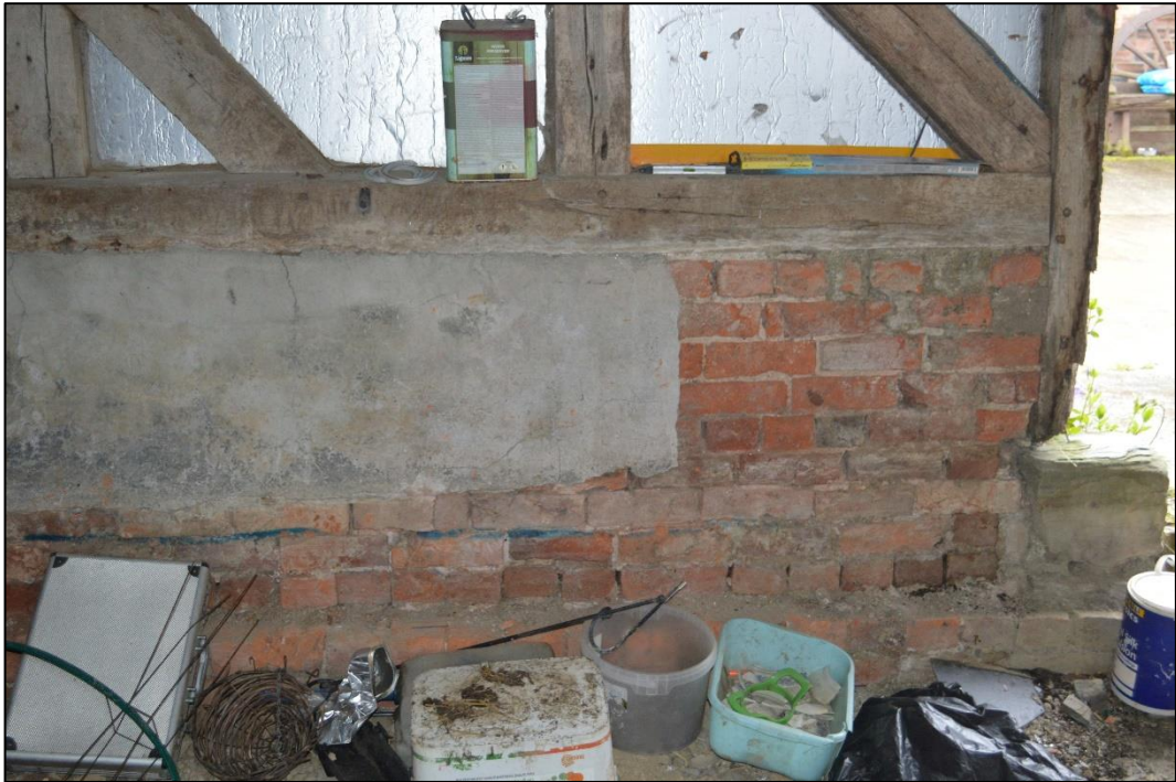
Figure 16: Brick step foundation at base of wall. Facing south. CPAT 5046_0003
