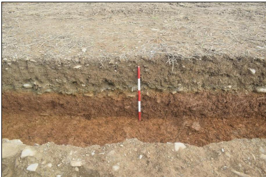
*Fig. 7 South-west facing section showing the road construction Photo CPAT 4963-033*
