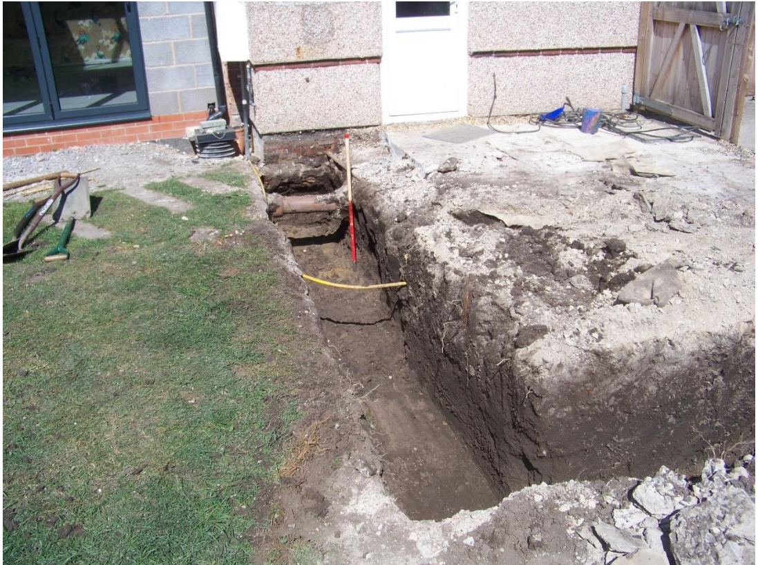
Figure 5 Western footing facing north
