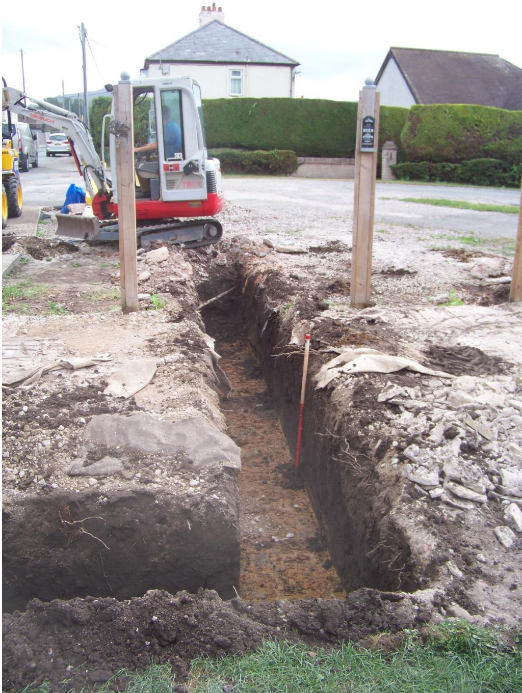
Figure 5 Southern footing facing east
