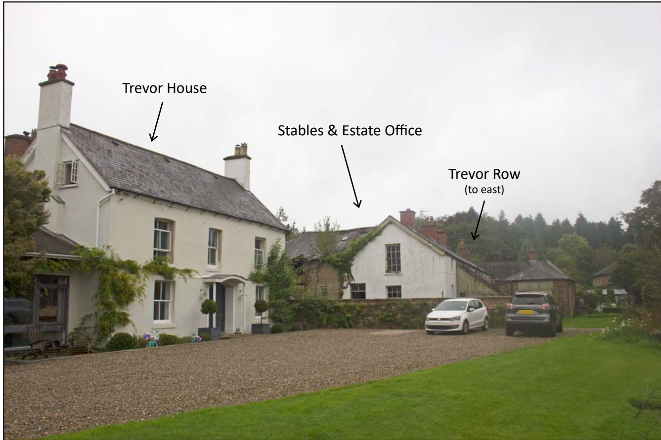
Plate 02: From Trevor House, context shot, former Estate Offices & Stables, Trevor Road, Chirk - from the west/southwest - no scale
