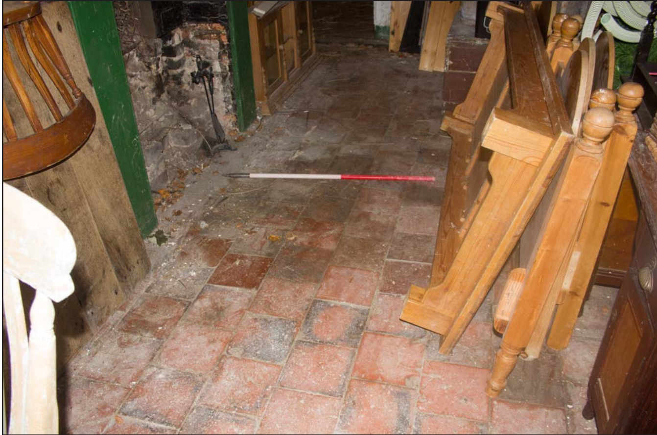
Plate 32: Internal shot of workshop floor, Estate Offices & Stables, Trevor Road, Chirk - from the north - 2.00m scale
