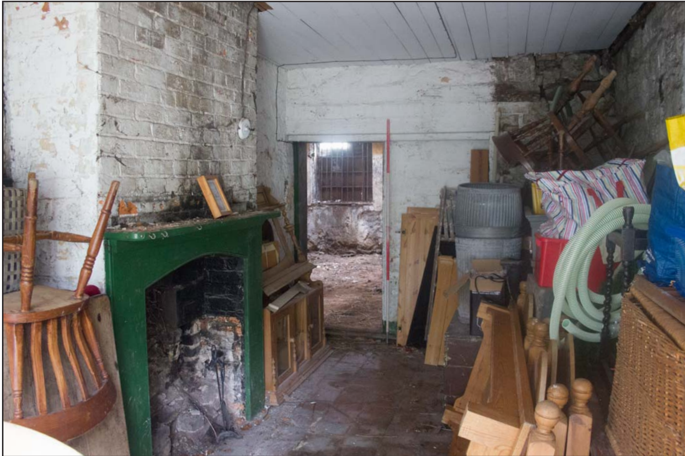
Plate 30: Internal shot of workshop, Estate Offices & Stables, Trevor Road, Chirk - from the south - 2.00m scale
