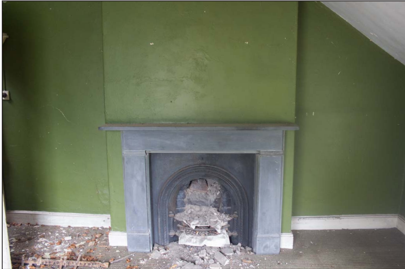
Plate 41: Internal shot of First Floor Office - Fireplace, Estate Offices & Stables, Trevor Road, Chirk - from the west - no scale
