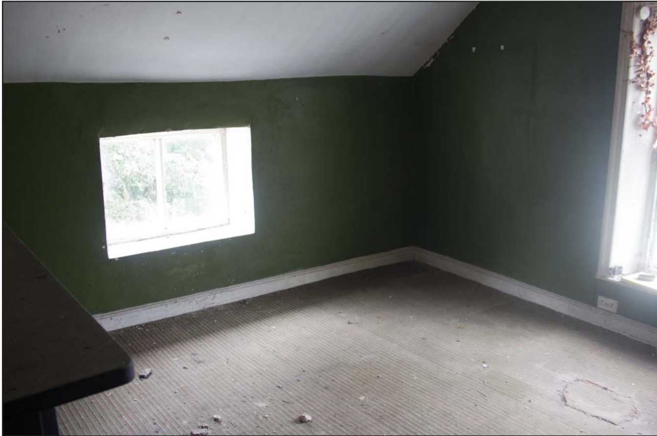
Plate 39: Internal shot of First Floor Office, Estate Offices & Stables, Trevor Road, Chirk - from the northeast - no scale
