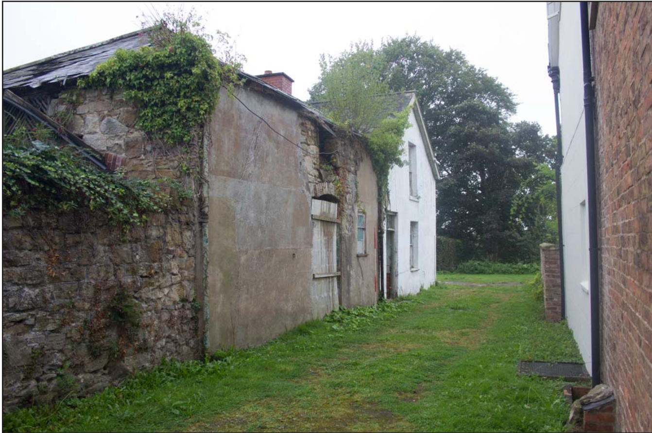
Plate 04: Western elevation, oblique shot, former Estate Offices & Stables, Trevor Road, Chirk - from the northwest - 2.00m scale
