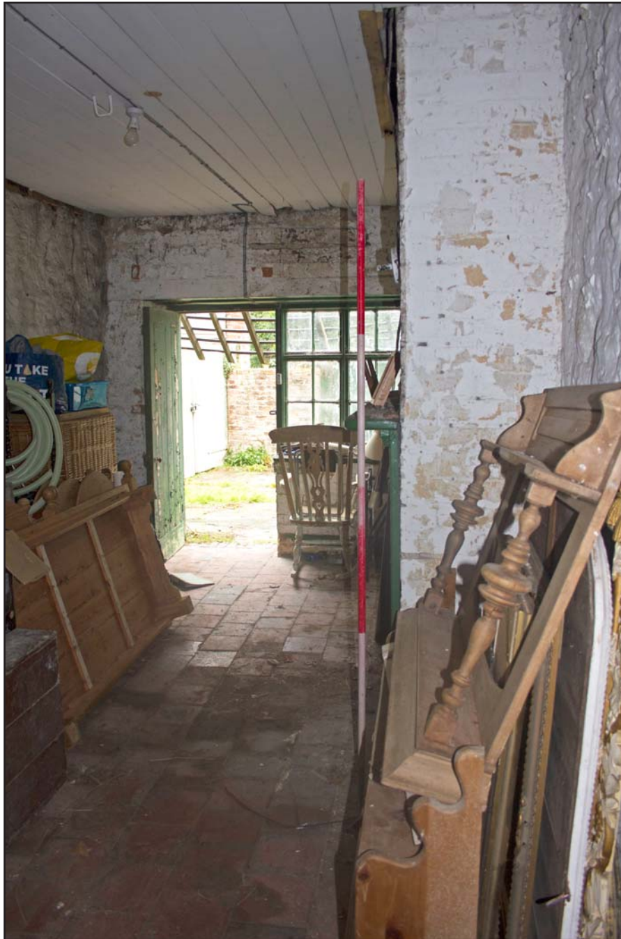
Plate 31: Internal shot of workshop, Estate Offices & Stables, Trevor Road, Chirk - from the north - 2.00m scale
