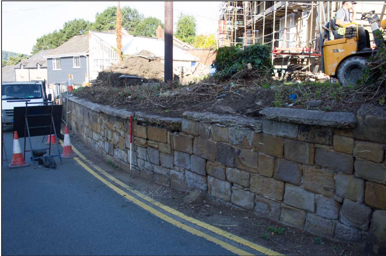
Plate 09: Fron Deg boundary wall, from the east. Scale 1.0m.
