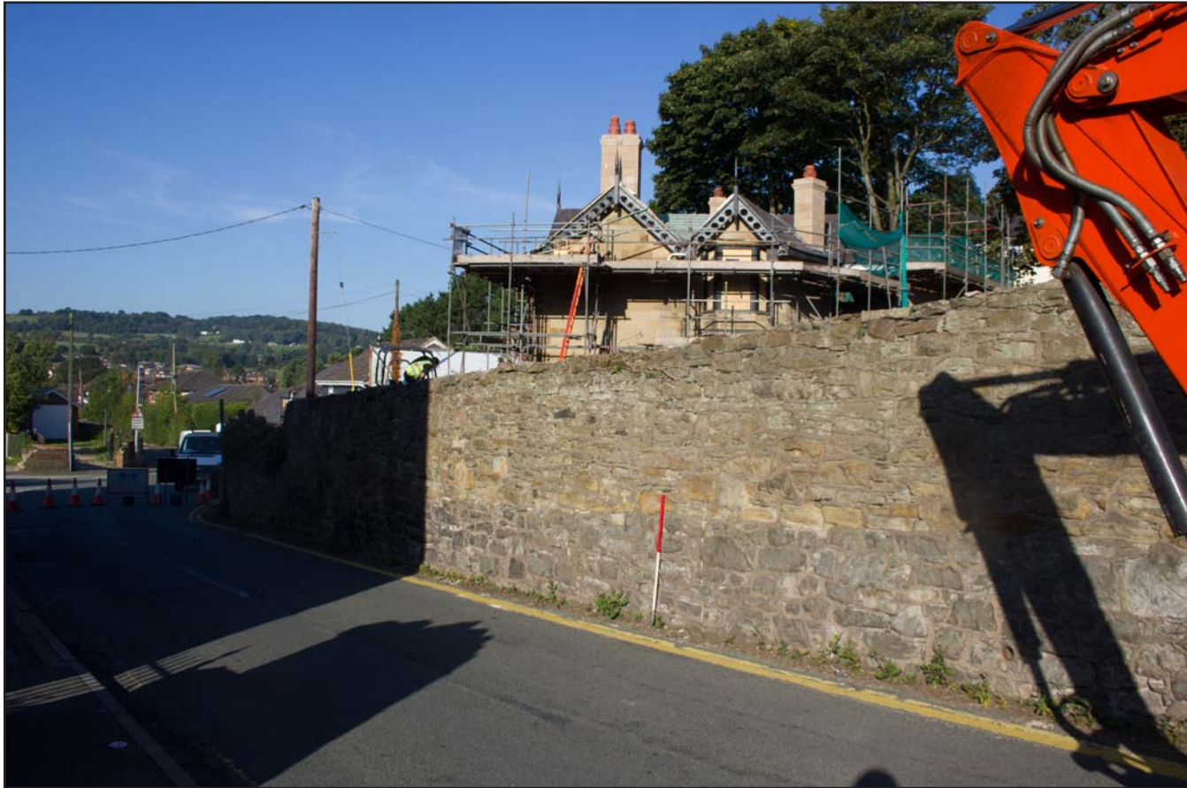
Plate 08: Fron Deg boundary wall, from the east. Scale 1.0m.
