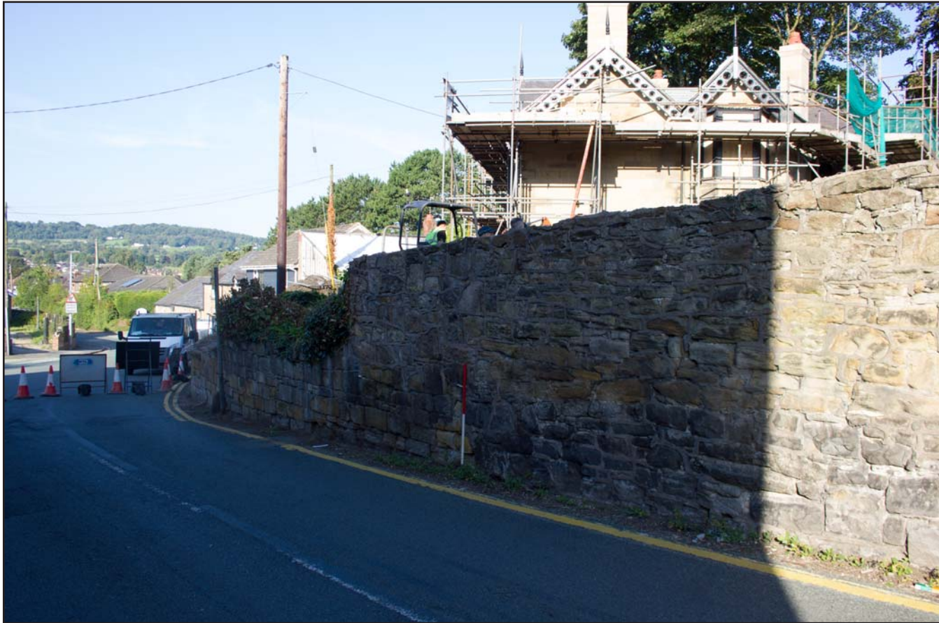
Plate 04: Fron Deg boundary wall, from the east. Scale 1.0m.
