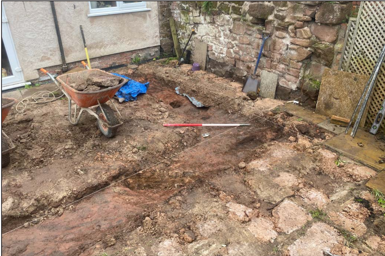
Plate 11: Post excavation shot of site, on land to rear of Rose Avon, Bridge Street, Holt, Wrexham - from the southeast - 1.00m scale
