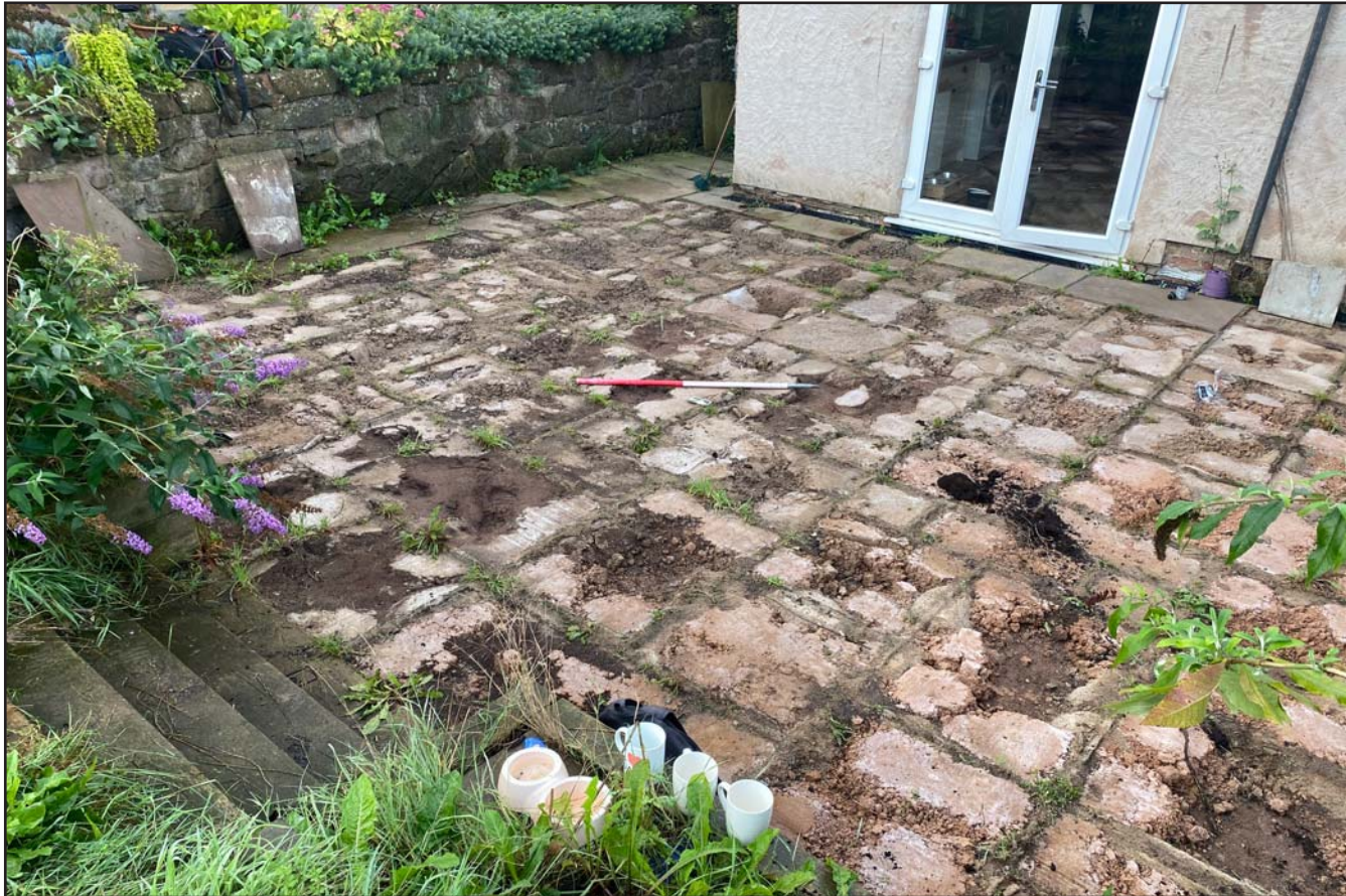
Plate 03: Pre excavation shot of site, on land to rear of Rose Avon, Bridge Street, Holt, Wrexham - from the northeast
