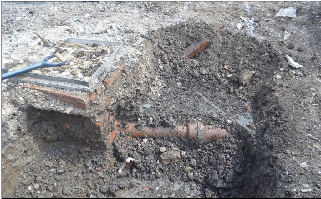
Figure 7: Sewage pipes on site. Facing east. CPAT 5074-0013.
