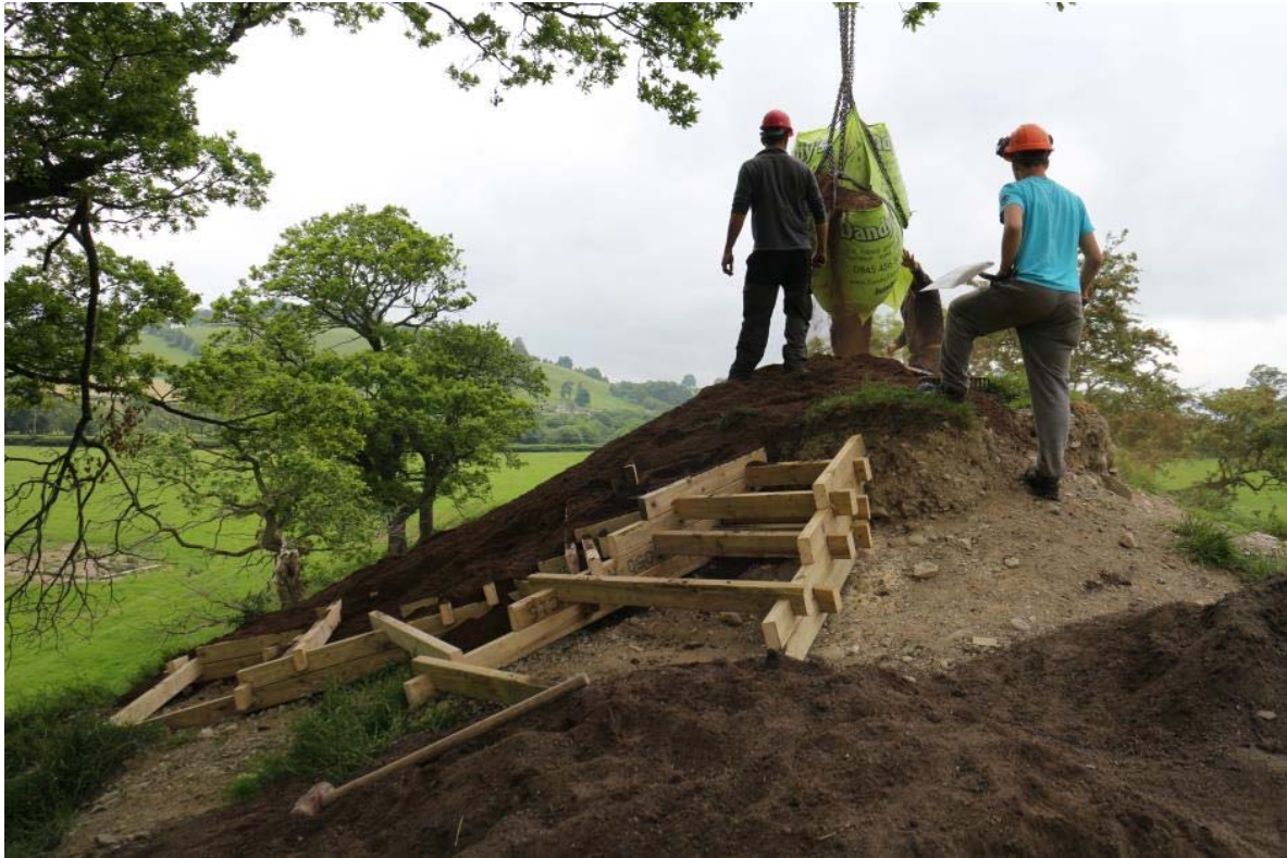
Topsoil delivery by crane to timber crib, IMG_7178, 25.06.2015
