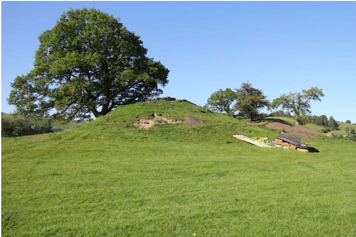
North side, early stages of repair, IMG_6989, 23.06.2015
