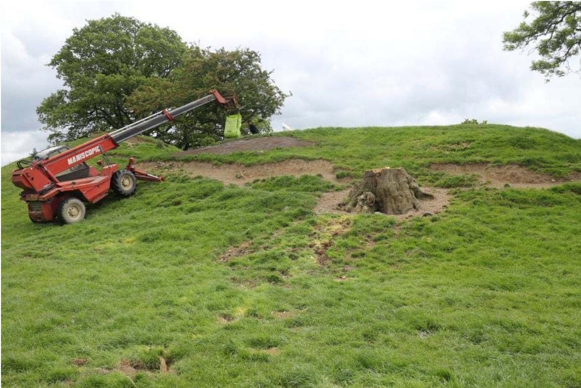
Commencing infilling of scars, IMG_6938, 22.06.2015
