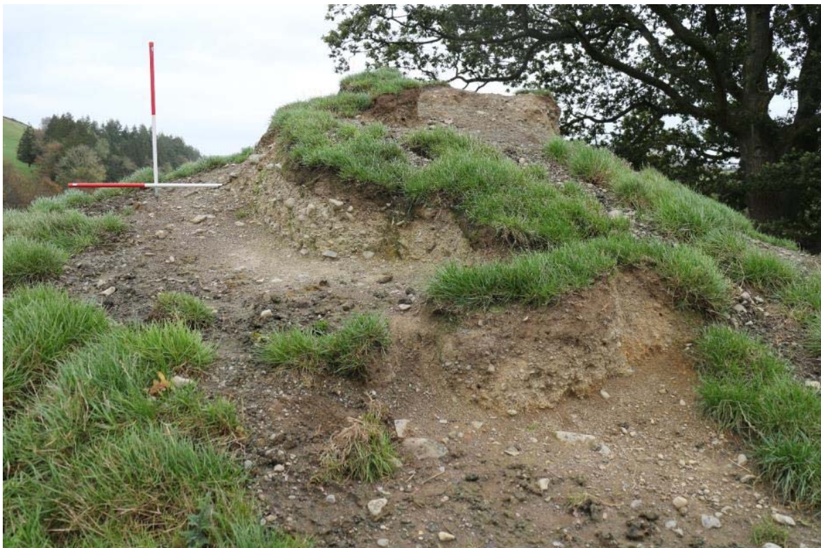
The motte summit, prior to repair, IMG_2525, 22.10.2014
