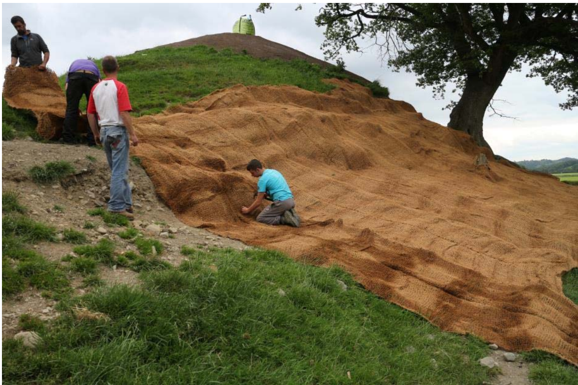
During repair, IMG_7222, 25.06.2015
