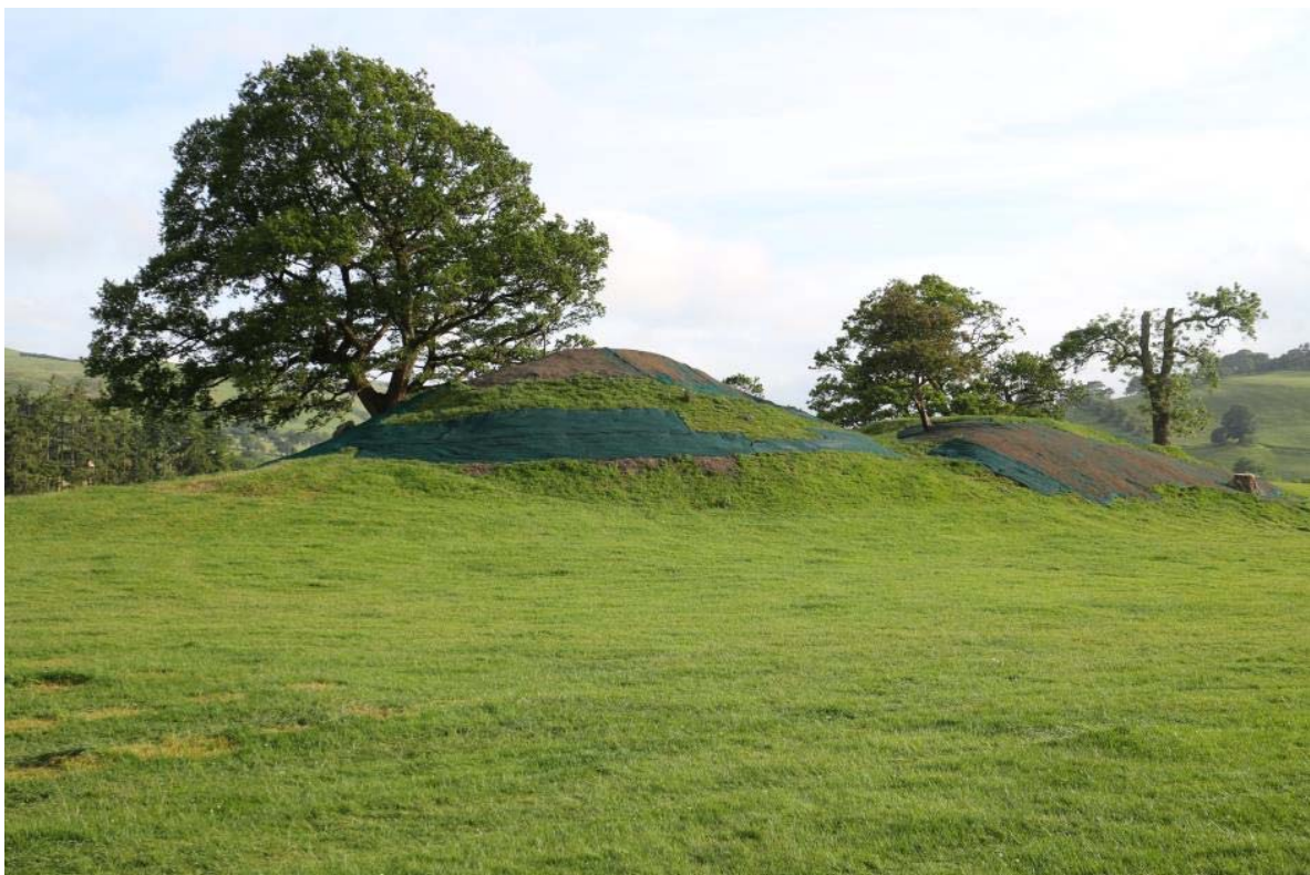
North side, immediately after completed repairs, IMG_7301, 26.06.2015
