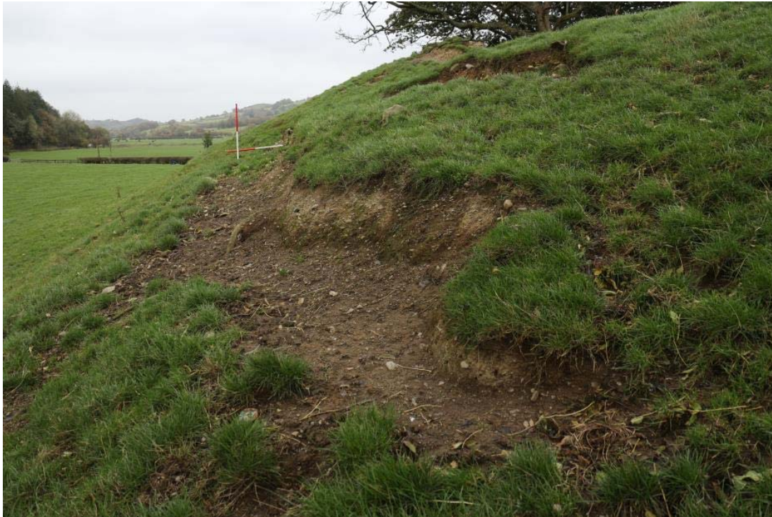
Prior to repair, IMG_2518, 22.10.2014
