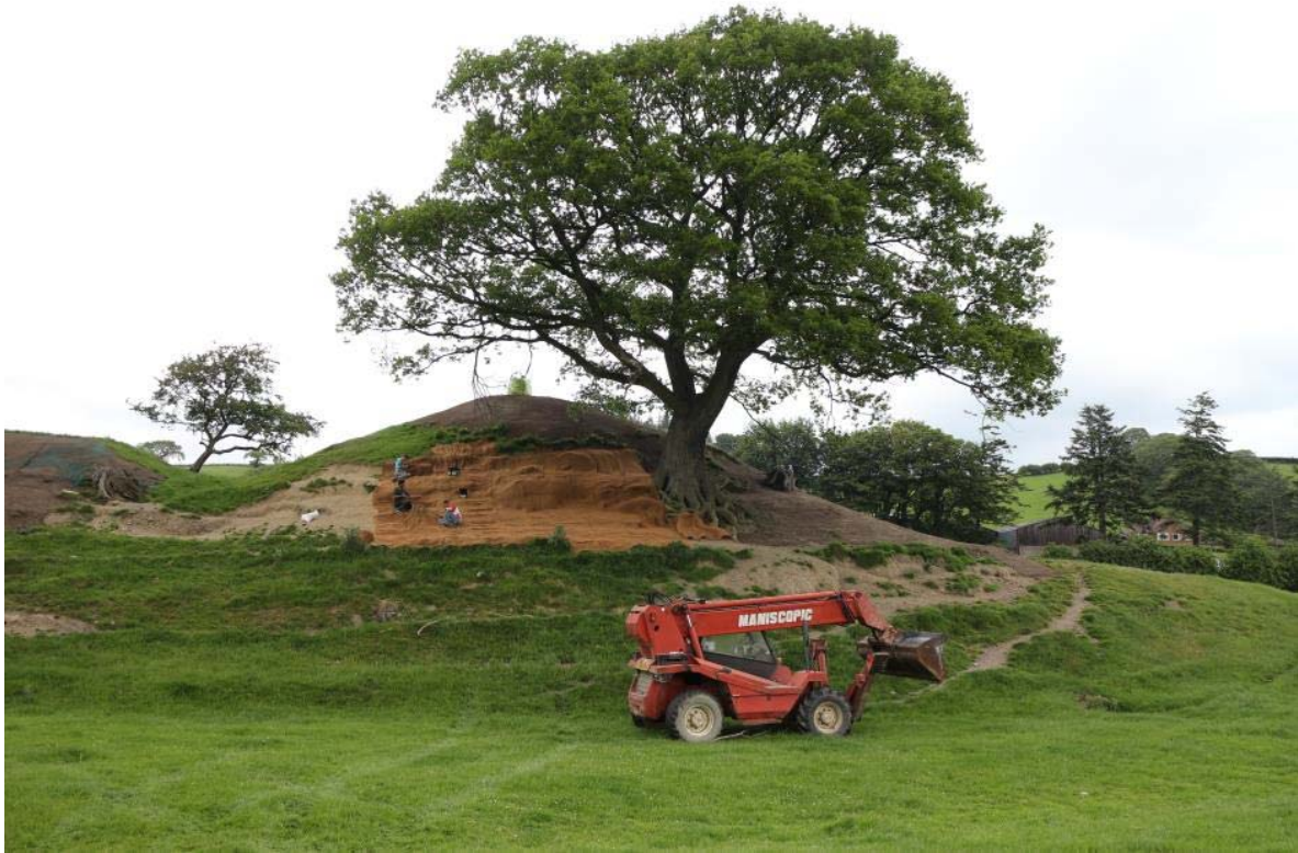
During repair, IMG_7214, 25.06.2015
