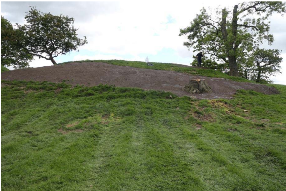
Infilling and profiling completed, IMG_6960, 22.06.2015
