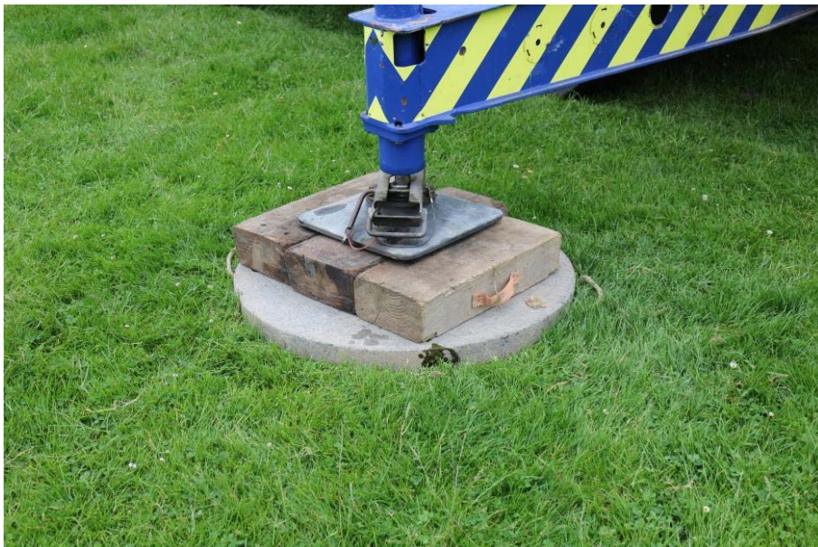
Crane stabiliser jack and load-spreading plate, IMG_7138, 25.06.2015
