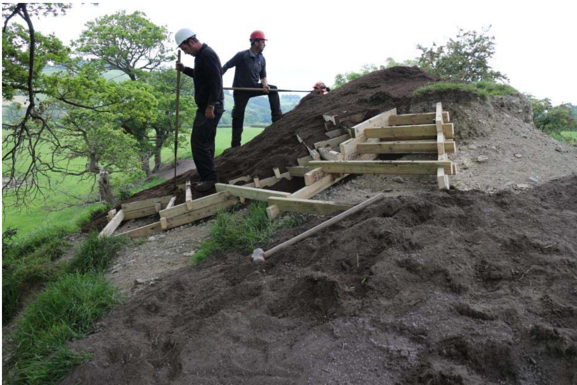
Commencing infilling timber crib, IMG_7173, 25.06.2015
