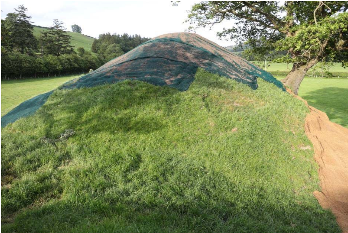
Completed repair to motte, looking east, IMG_7287, 26.06.2015
