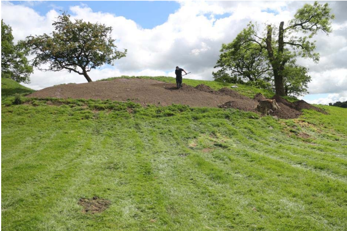
Compacting and profiling infill topsoil, IMG_6949, 22.06.2015
