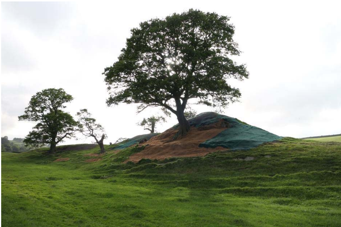
South side, immediately after completed repairs, IMG_7274, 26.06.2015
