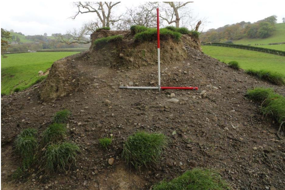
The motte summit, prior to repair, IMG_2527, 22.10.2014
