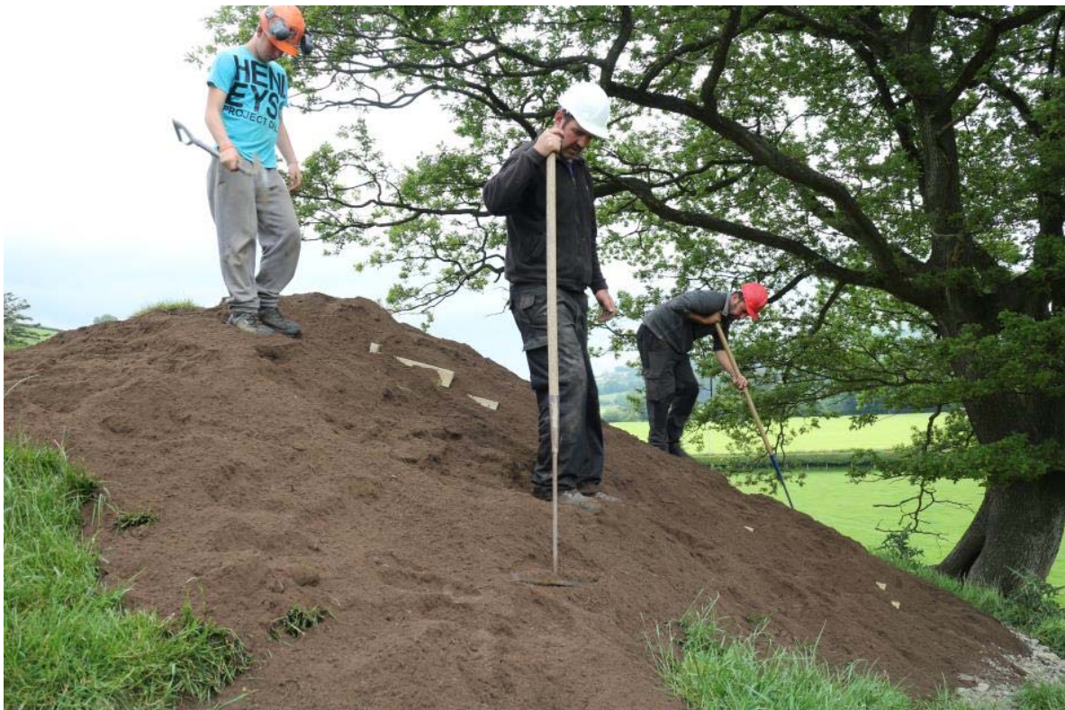
Compacting infill topsoil, IMG_7185, 25.06.2015
