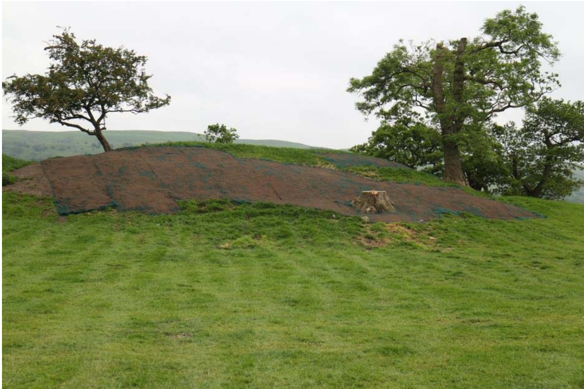
Completed repair, IMG_7108, 25.06.2015
