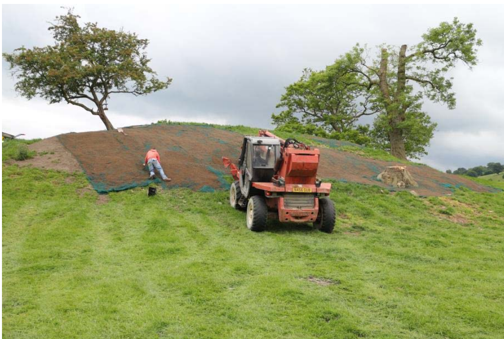
Top-dressing installed Western Excelsior Excel PP5-12 TRM, IMG_7097, 24.06.2015
