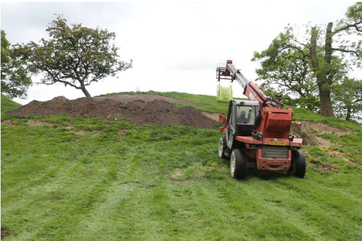
Infilling of scars in progress, IMG_6946, 22.06.2015
