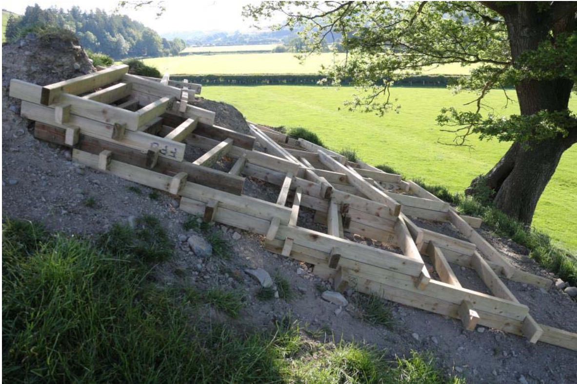
Completed timber crib, IMG_7032, 24.06.2015
