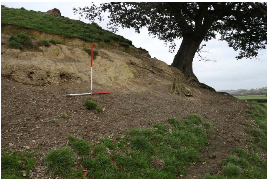
Prior to repair, IMG_2535, 22.10.2014
