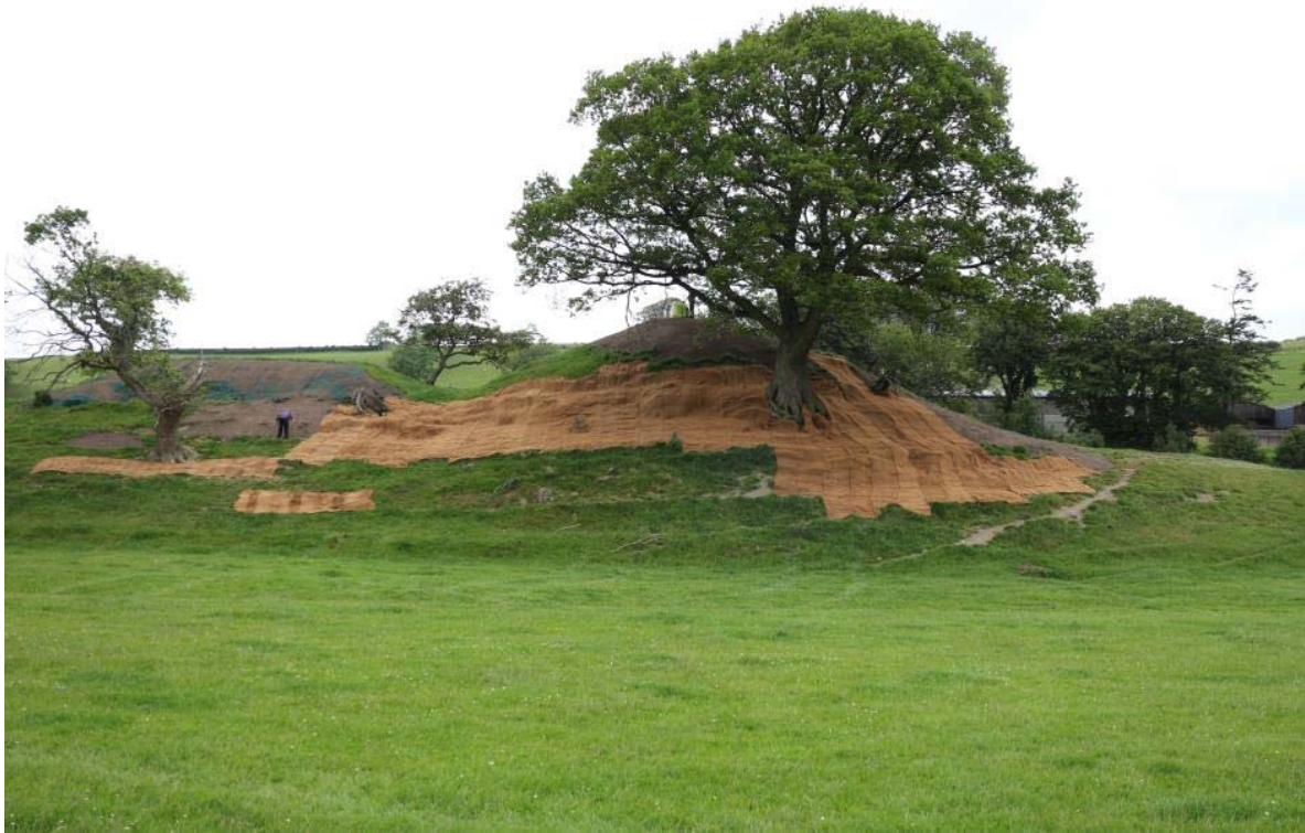
Completed repair, IMG_7236, 25.06.2015
