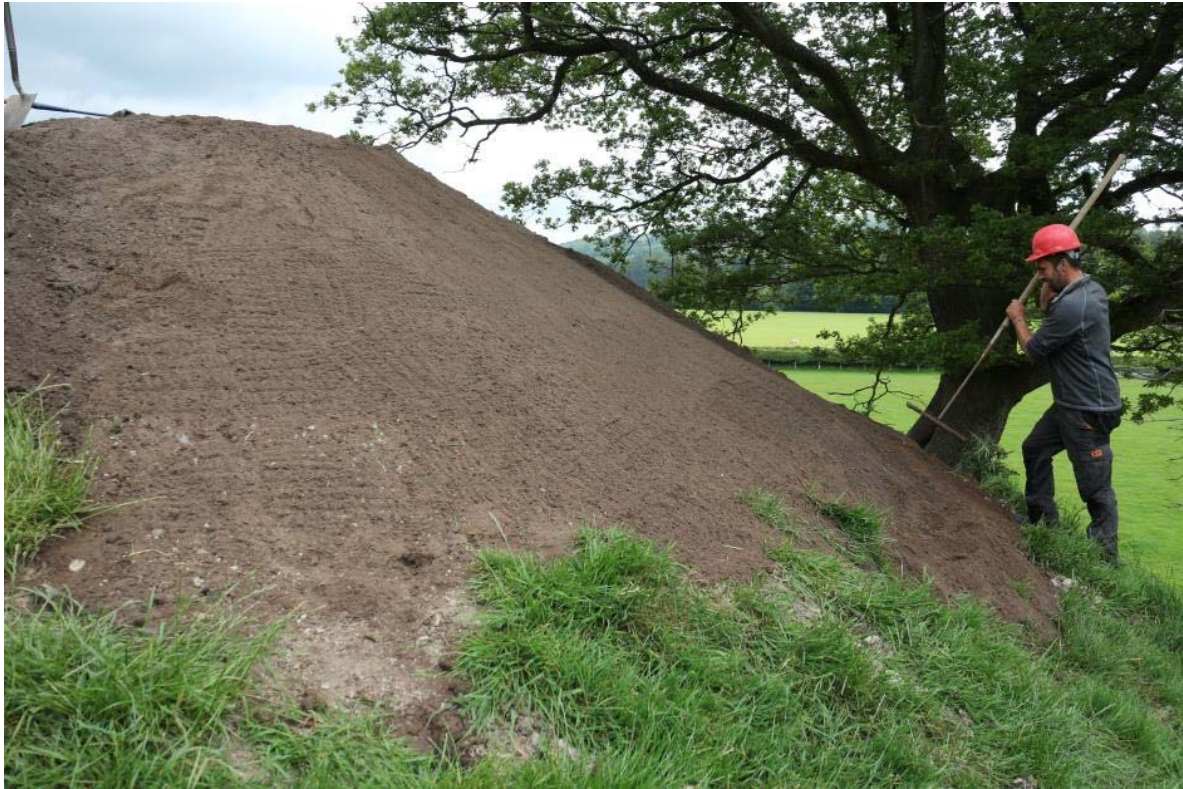
Final profiling of infill topsoil, IMG_7205, 25.06.2015
