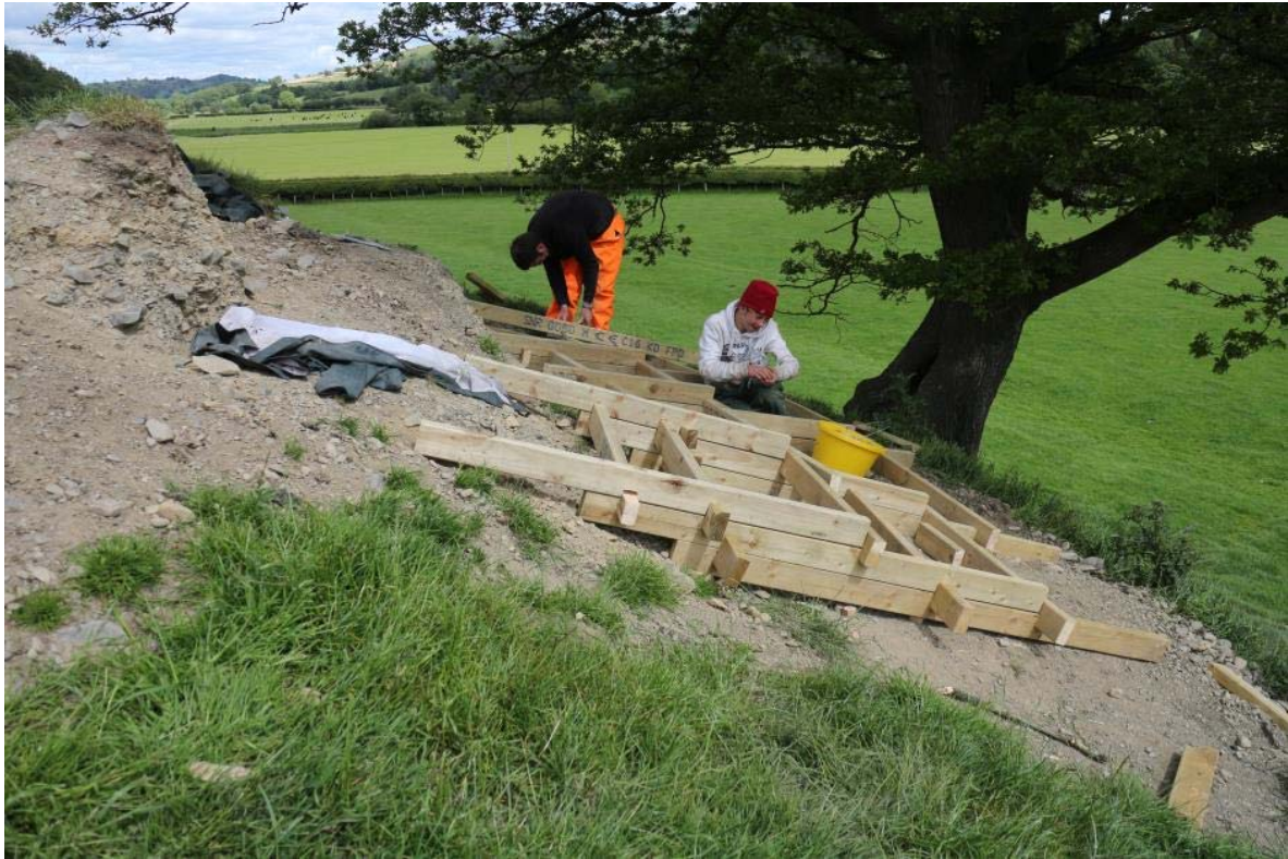
Commencing construction of timber crib, IMG_6956, 22.06.2015
