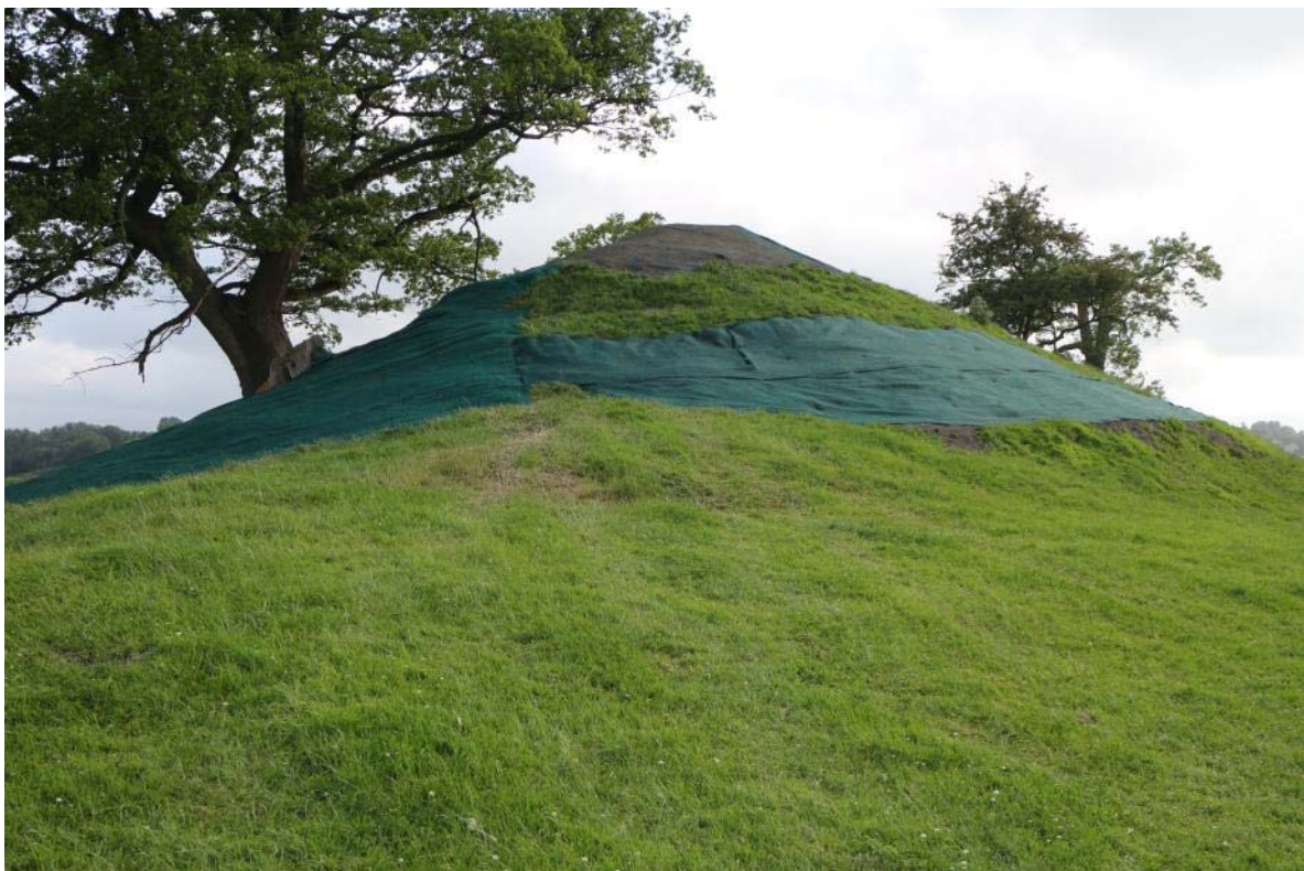
Completed repair to motte, looking west, IMG_7272, 26.06.2015
