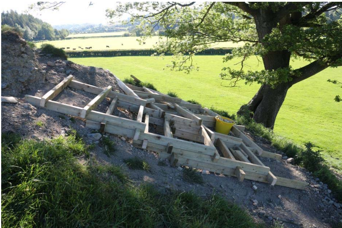
Midway through construction of timber crib, IMG_6979, 23.06.2015
