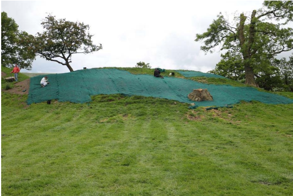
Installing Western Excelsior Excel PP5-12 Turf Reinforcement Matting, IMG_7070, 24.06.2015
