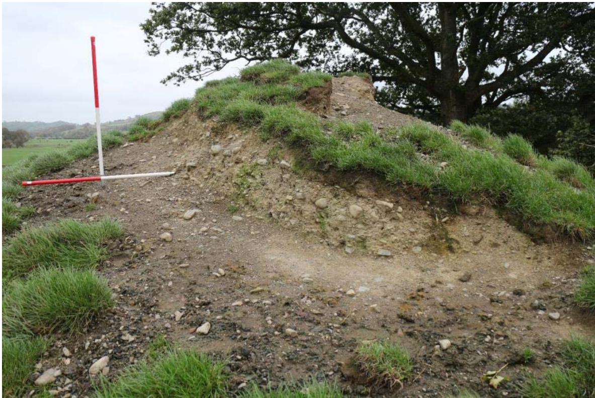
The motte summit, prior to repair, IMG_2524, 22.10.2014
