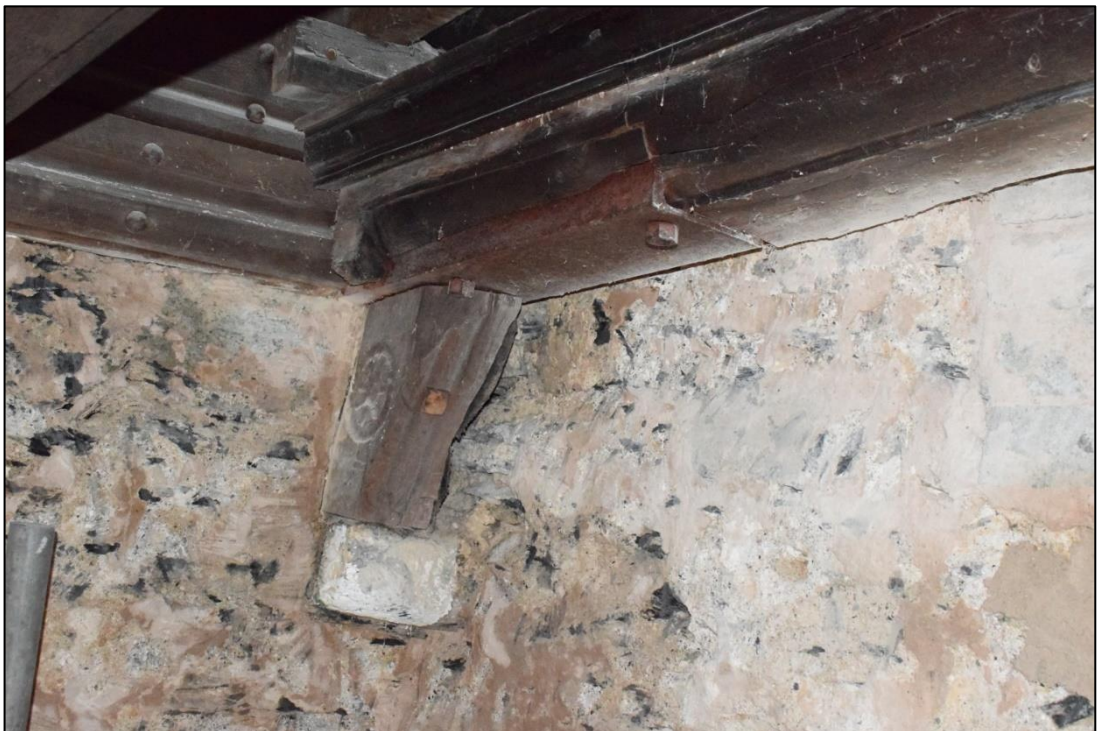
Fig. 21: Repairs at the south-west corner of the chapel roof. CPAT 4679-0162
