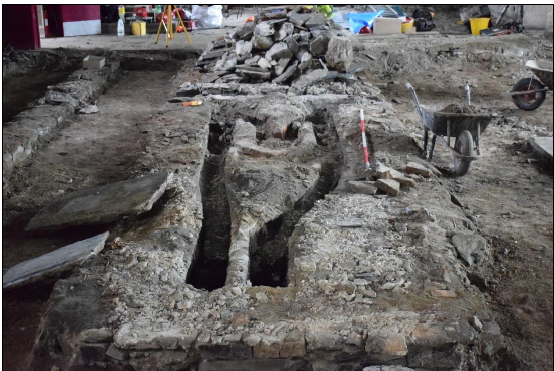
Fig. 13: Underfloor ducts in the nave, most likely from a 19 th -century heating system. CPAT 4679-0057
