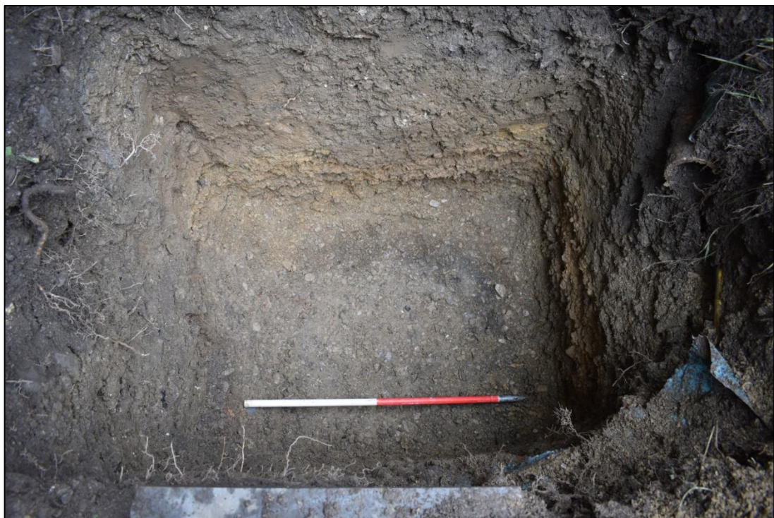
Fig. 24: The trench excavated to place the new sewage treatment plant, showing the outline of the grave, from the west. The end of the repositioned ledger 15 is visible in the foreground. CPAT 4679-0120
