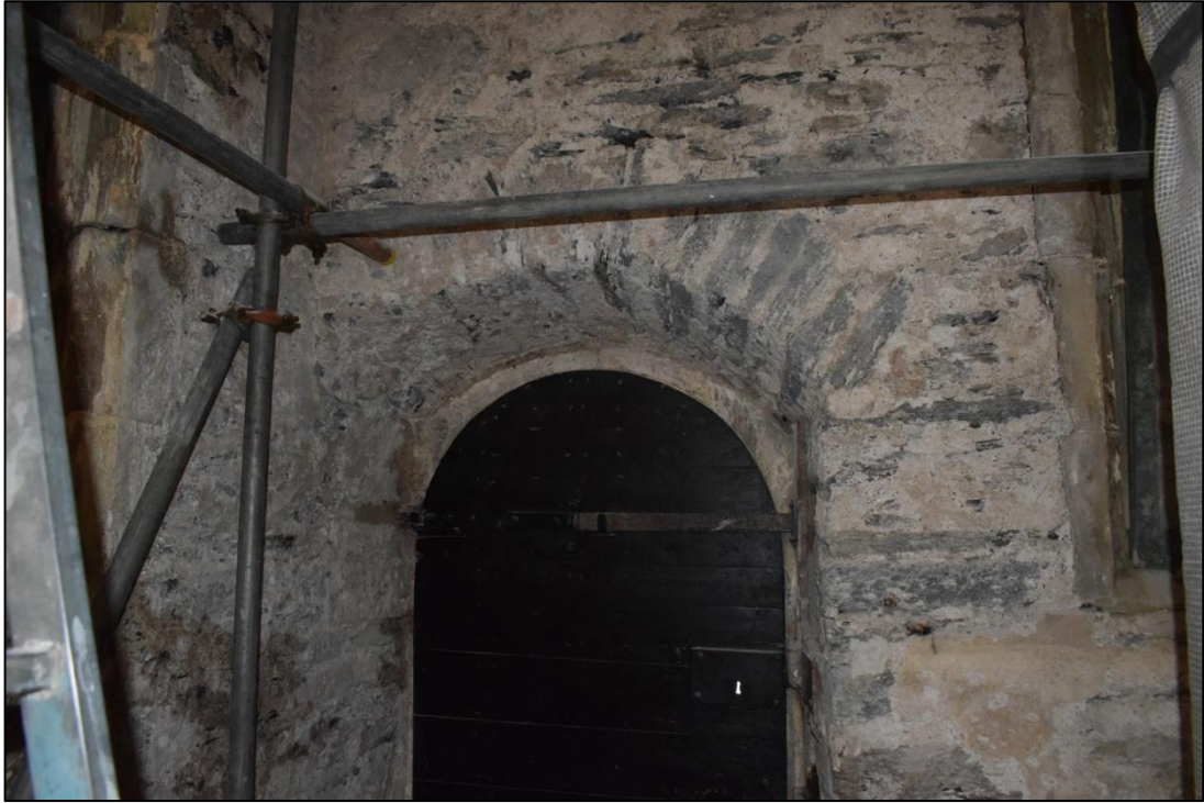
Fig. 22: The stone arched doorhead at the external door at the south-west corner of the chapel. CPAT 4679-0169
