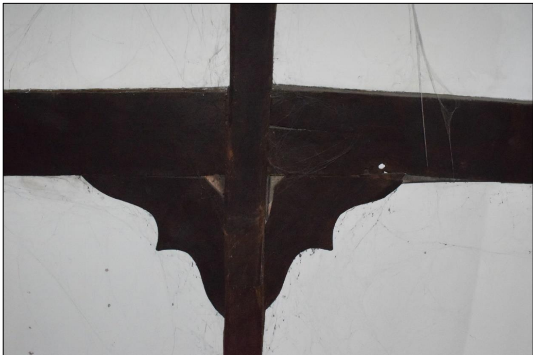
Fig. 18: Windbraces on the roof truss crossing the rood screen, which most likely provided an overall appearance copied to shape those in the north aisle (see Fig. 19). CPAT 4679-0182
