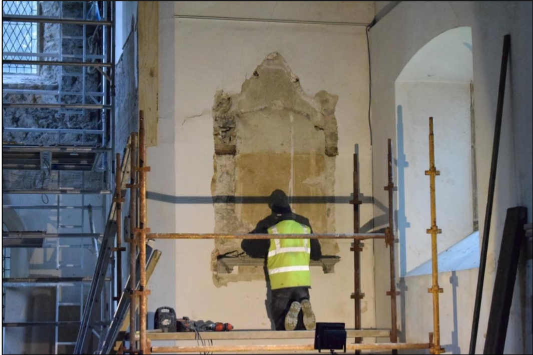
Fig. 14: The wall monument on the west wall of the nave, to the north of the tower in the process of being taken down, and moved to the north wall of the north aisle. CPAT 4679-0115
