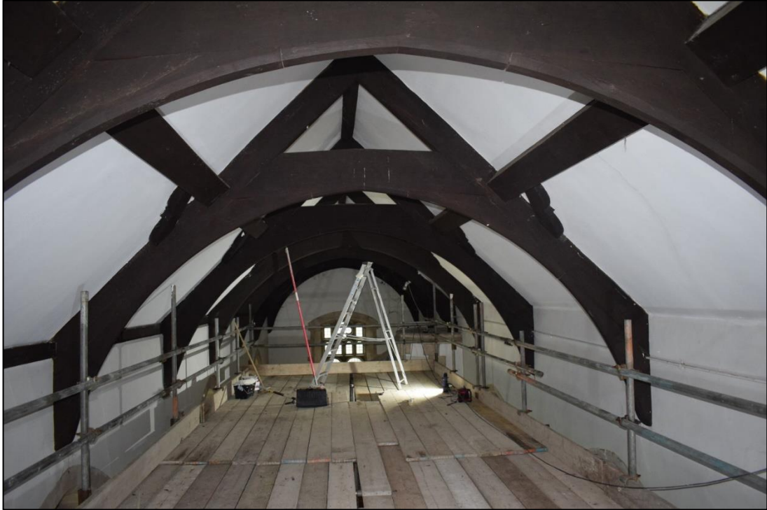
Fig. 19: The roof trusses of the north aisle. CPAT 4679-0173
