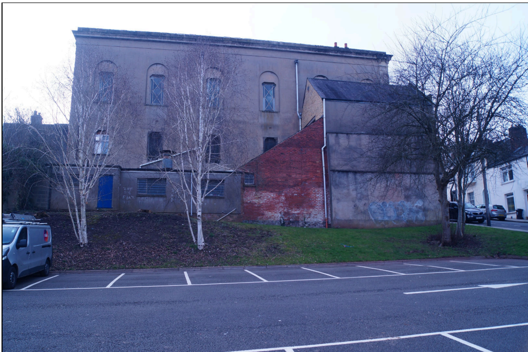
Plate 30: A view of the plain, unadorned eastern elevation of Victoria Road Chapel from the proposed development site. Deciduous trees screen the view in summer. This view was left plan as Hill Street was already in place when the chapel was built and would not be readily visible. Looking west-southwest.
