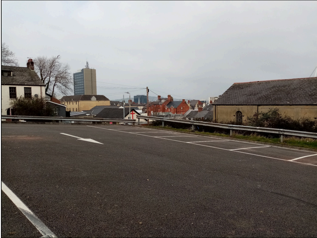
Plate 21: A view from the development site in Hill Street Car Park towards the red-brick listed buildings in Commercial Road. They are listed for their impressive facades but only the rear of the buildings are visible from here. Looking north-northeast.
