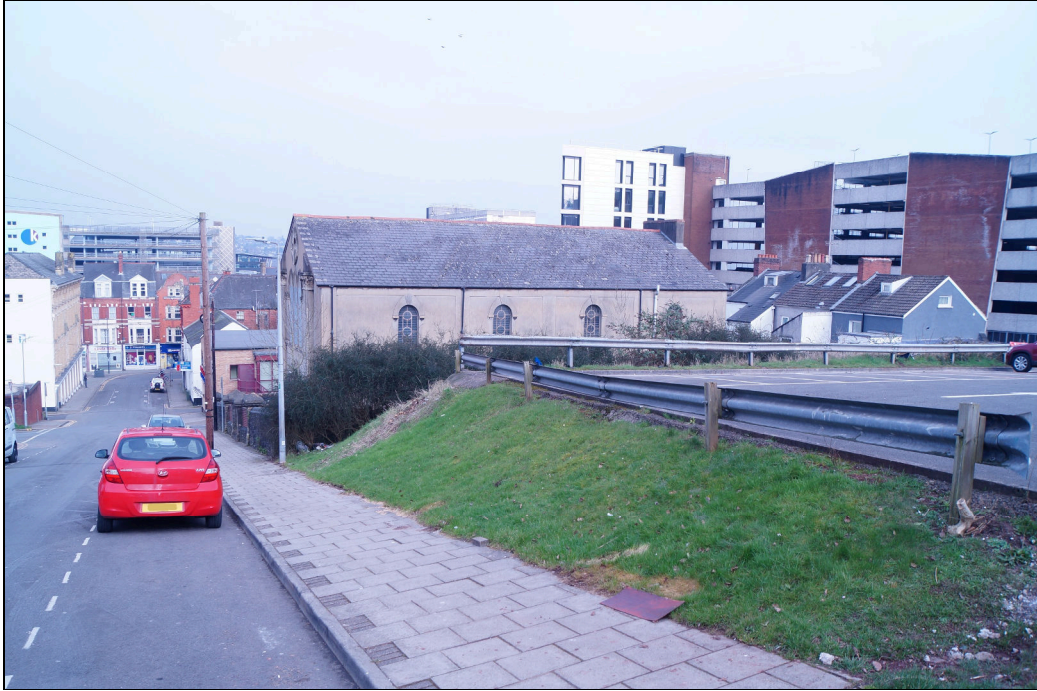
Plate 25: A view down Hill Street along the northern side of car park, showing the depth of material added to the site to level the surface. Commercial Street is glimpsed at the bottom of the slope. Looking east-northeast.
