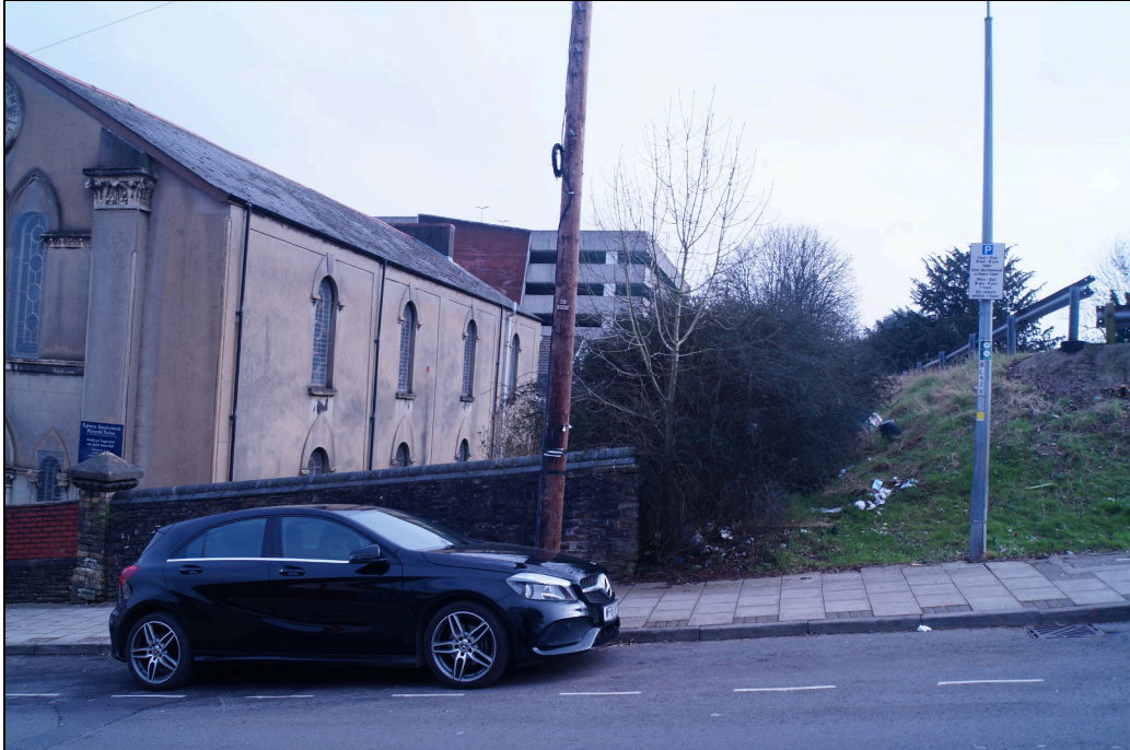
Plate 13: A view of the gap between Mount Zion chapel to the left and the bottom of Hill Street Car Park to the right. This shows the considerable depth of material added to level up the Hill Street Car Park on the steeply sloping ground which formerly existed here. Looking south-southeast.
