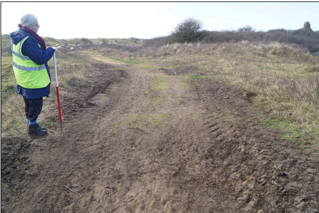
Plate 30: KFD2021_130. Part of the trackway through the Scheduled Monument, after the bog mats had been removed. Looking east-northeast. SS8016382669
