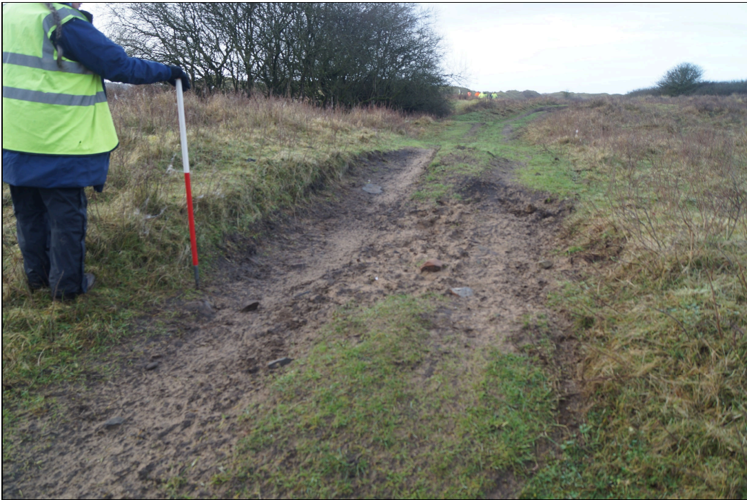
Plate 1: KFD2021_101. Part of the trackway through the Scheduled Monument showing existing erosion, looking west-southwest. SS8020182690. This part of the trackway was not used for access by the project due to flooding to the east of this location.
