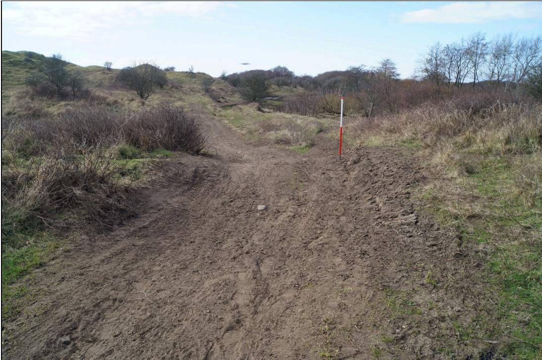
Plate 37: KFD2021_137. Part of the trackway through the Scheduled Monument showing existing erosion, after the bog mats had been removed. The medieval town bank is visible crossing the track from left to right. Stones are becoming exposed. Looking west. SS7997882593
