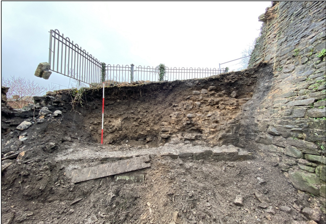
Plate 17. View to the east of the excavated and cleaned section (following the collapse) showing the masonry of the Northeast Tower [012], medieval deposits (011) and later back-filling deposits (013, 014 and 015).
