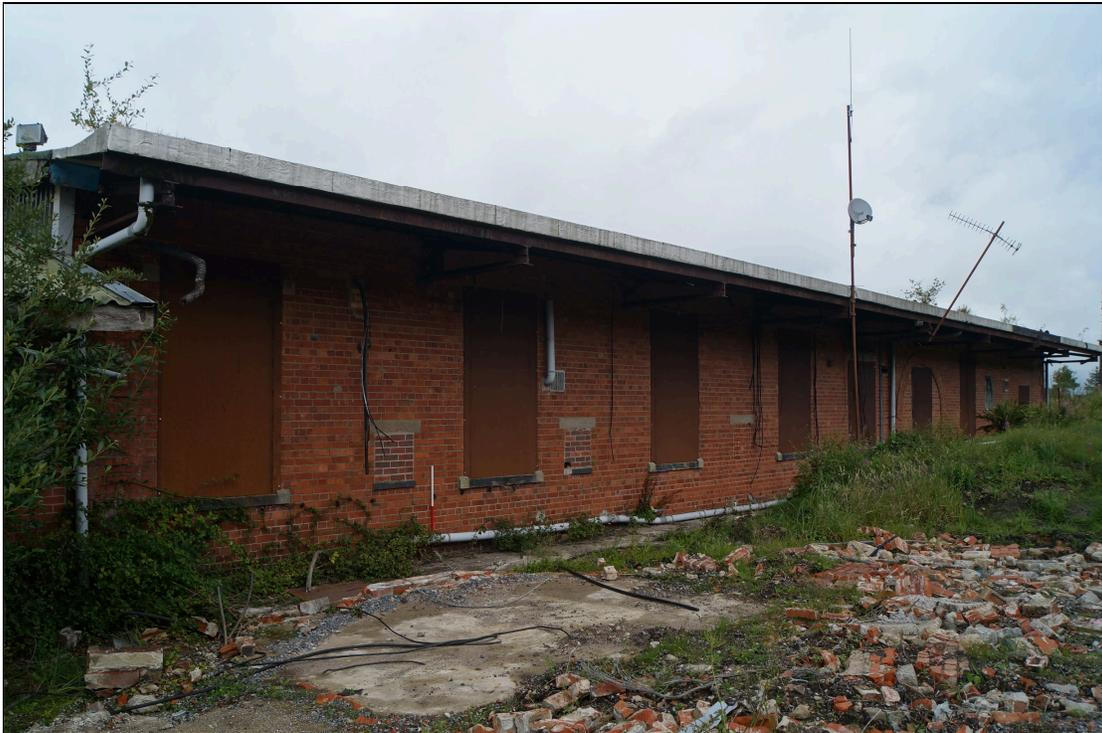
*Plate 16: A view of the southeast elevation of the lamp room building (ID Number 13). The three blocked up hatches visible in the wall were the hatches through which the miners returned their safety lamps at the end of a shift, protected by the broad overhang of the roof. The large windows, now shuttered, gave good light inside the building. Looking north.*
