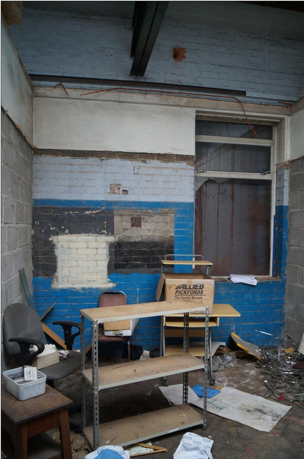
*Plate 49: A view of the original lamp room showing a shuttered window and bricked-up hatch from the inside the building. Looking northwest.*
