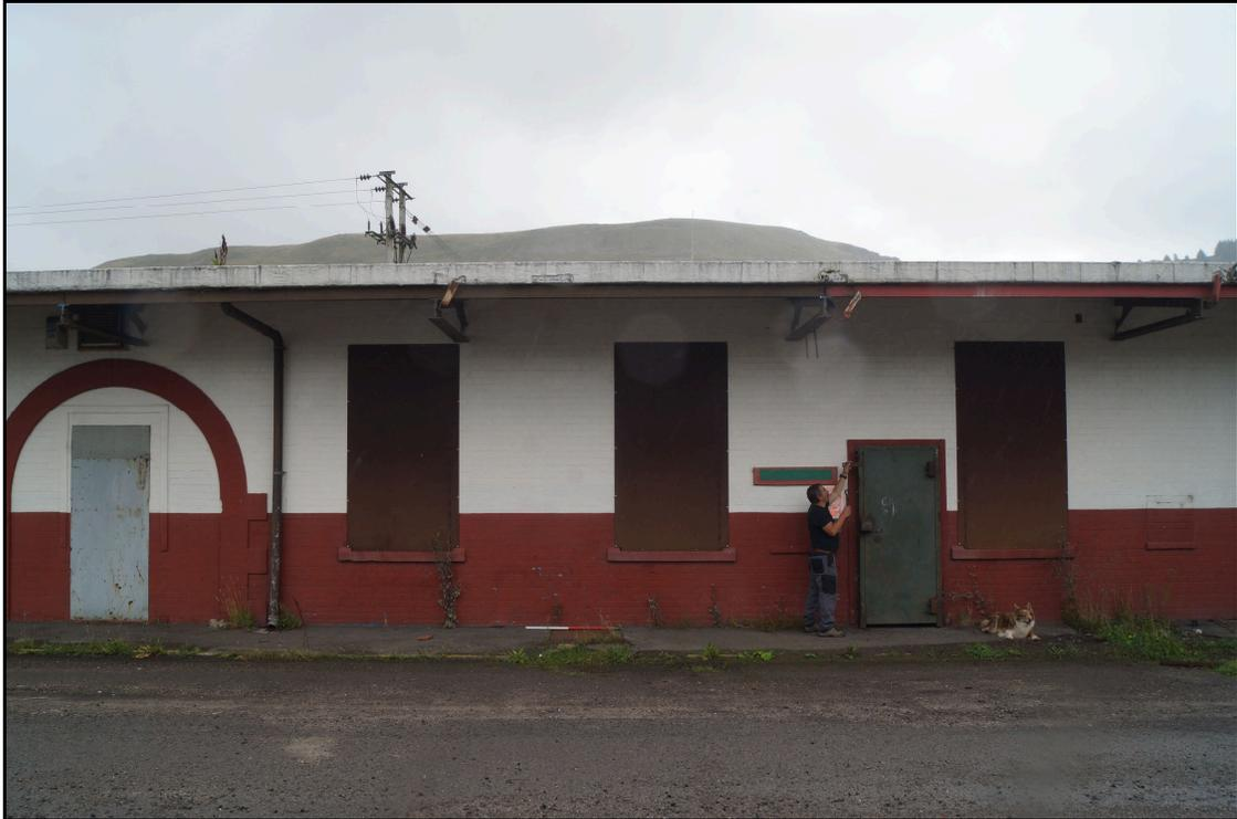
Plate 42: A view of the centre of the northwest elevation of the lamp room. The large windows of the lamp room are shuttered and the small hatches where safety lamps were passed out to miners walking to the pithead at the start of their shift can be seen as bricked-up features between the shuttered windows. Looking southeast.
