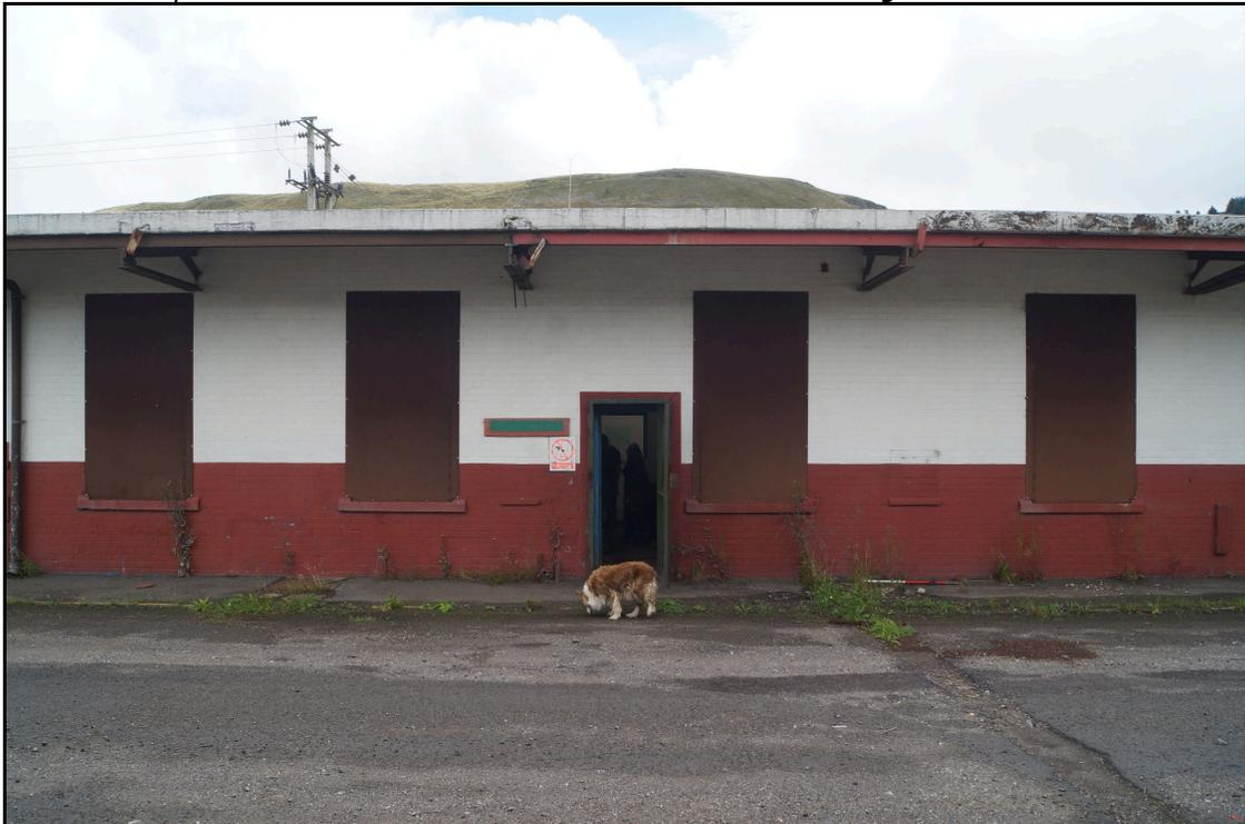
Plate 43: A view of the southern end of the northwest elevation of the lamp room. The large windows of the lamp room are shuttered and the small hatches where safety lamps were passed out to miners walking to the pithead at the start of their shift can be seen as bricked-up features between the shuttered windows. Looking southeast.
