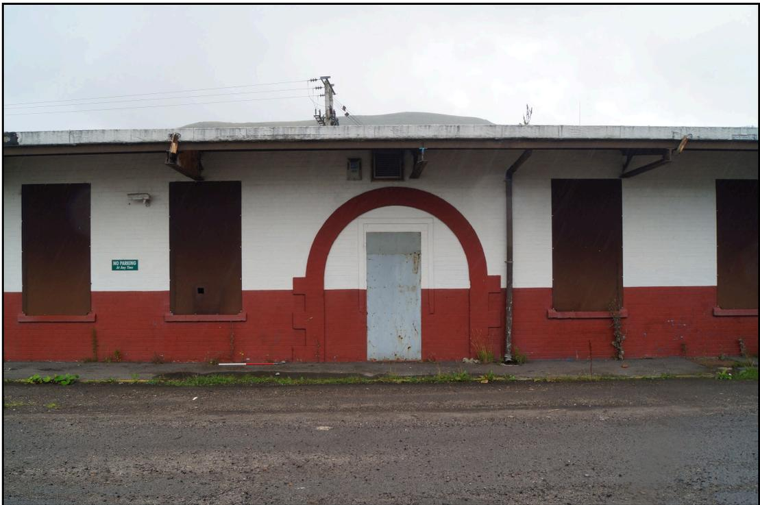
*Plate 41: A view of the brick archway in the northwest elevation of the lamp room. An open ended passage ran through the building here, dividing the lamp room to its right from the colliery offices to its right. It was blocked up during the later 20<sup>th</sup> century when the office space was extended. Looking southeast.*
