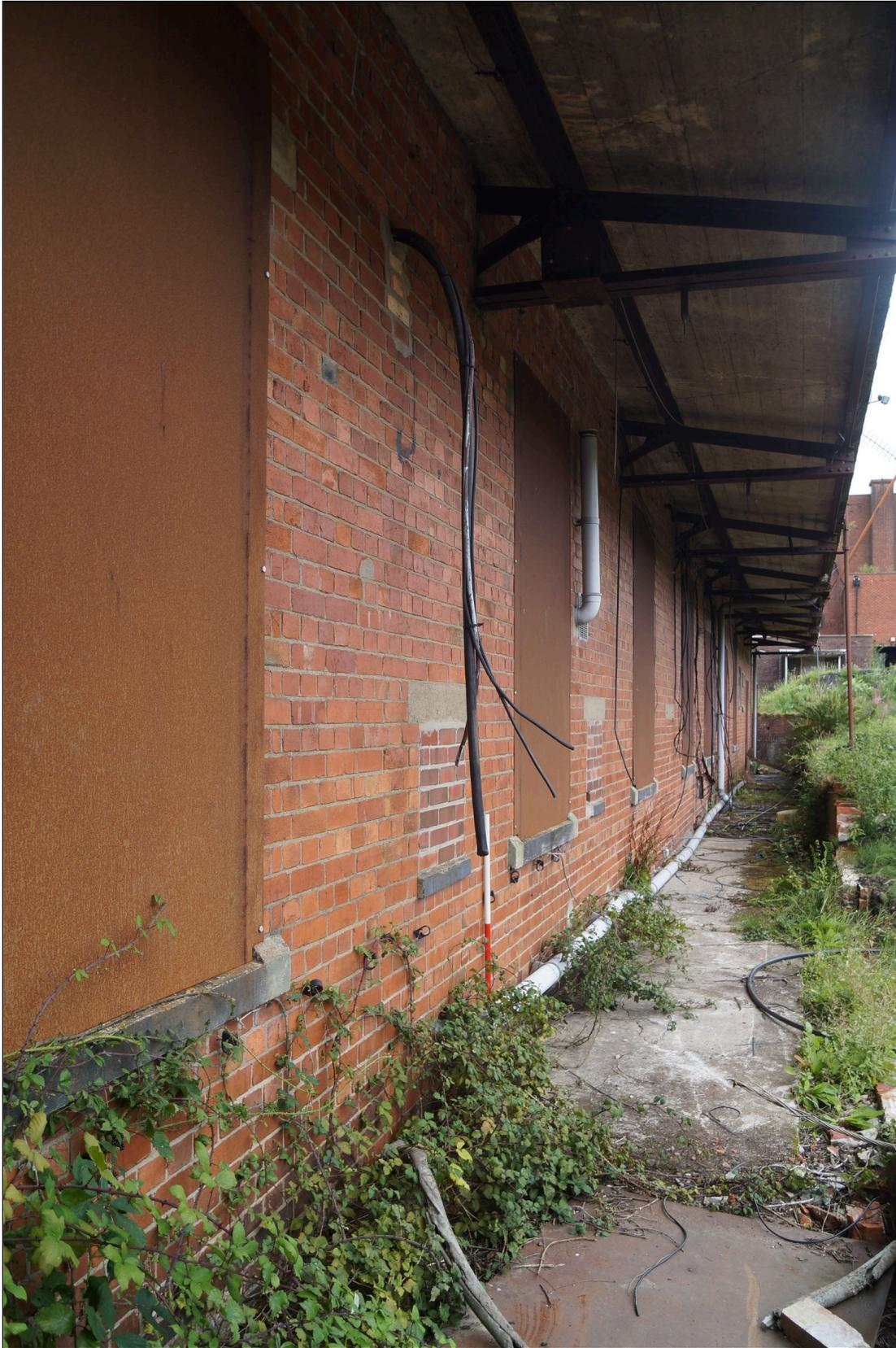
*Plate 17: A view along the southeast elevation of the lamp room showing the bricked-up hatches and the broad overhang of the steel-framed roof. Looking north-northeast.*
