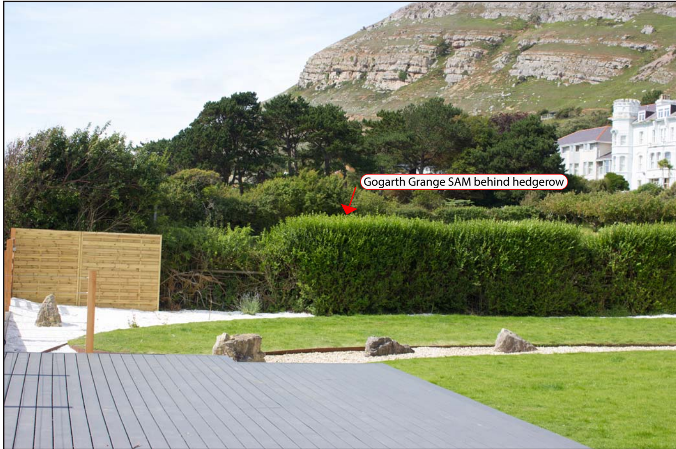
Plate 06: View from the Garden Room decking at the rear of Abbey Lodge towards the Gogarth Grange SAM, from the southeast (taken at 35mm focal length to simulate actual viewpoint).
