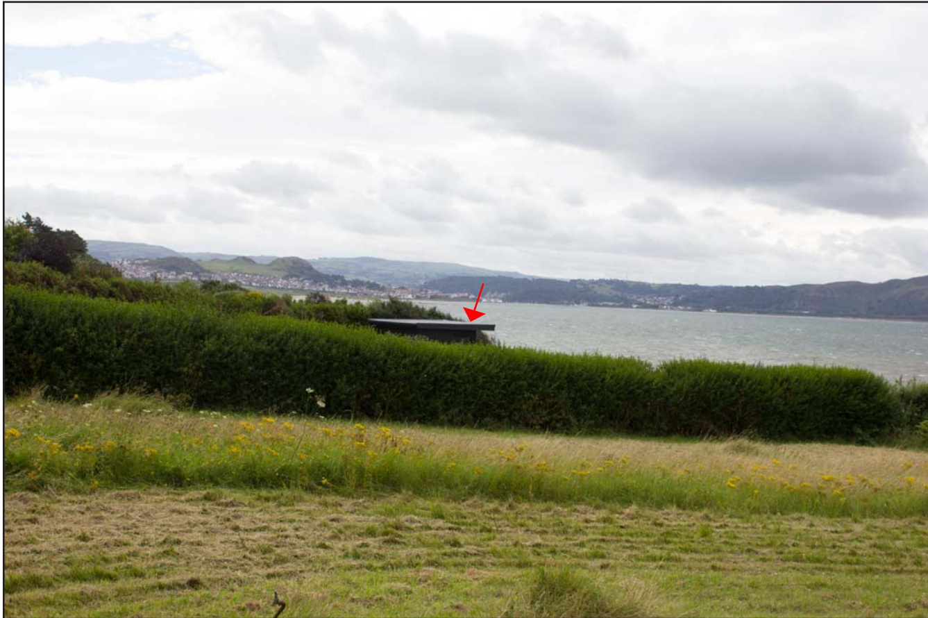
Plate 03: View from the Gogarth Grange SAM towards the Garden Room and decking to the rear of Abbey Lodge, from the northwest (taken at 35mm focal length to simulate actual viewpoint).
