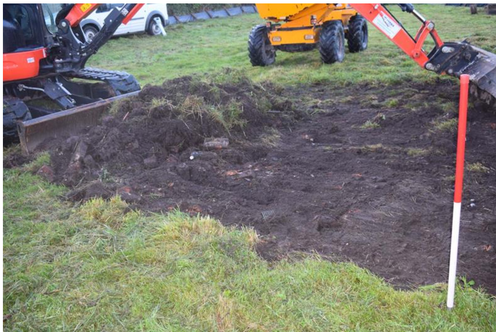
Figure 6 Topsoil stripping, with brick material and waste. Viewed from north west. CPAT Photo 4957-0005
