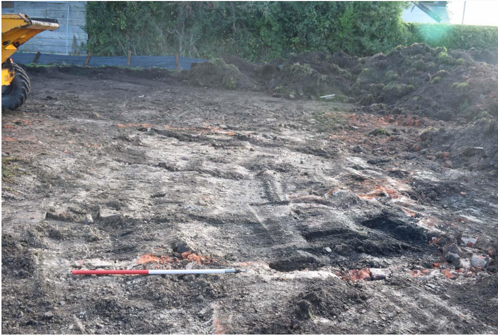
Figure 9 Lean-to room with coal-rich deposit in south-west corner of room. Viewed from west. CPAT photo 4957-0014
