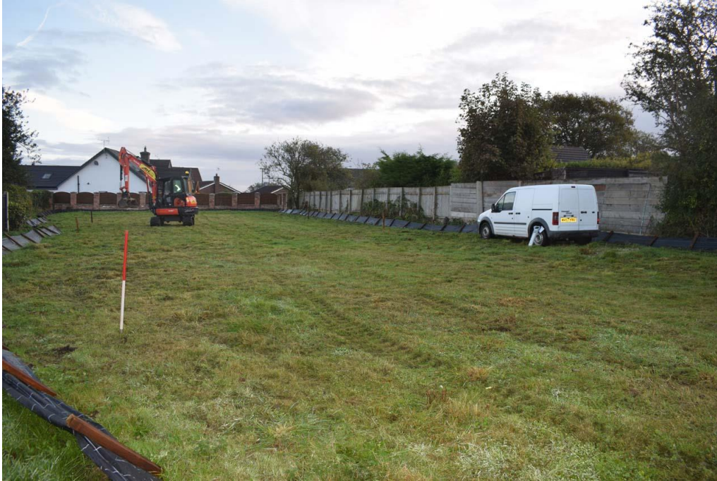
Figure 5 Site of development plot before stripping. Viewed from south. CPAT Photo 4957-0001
