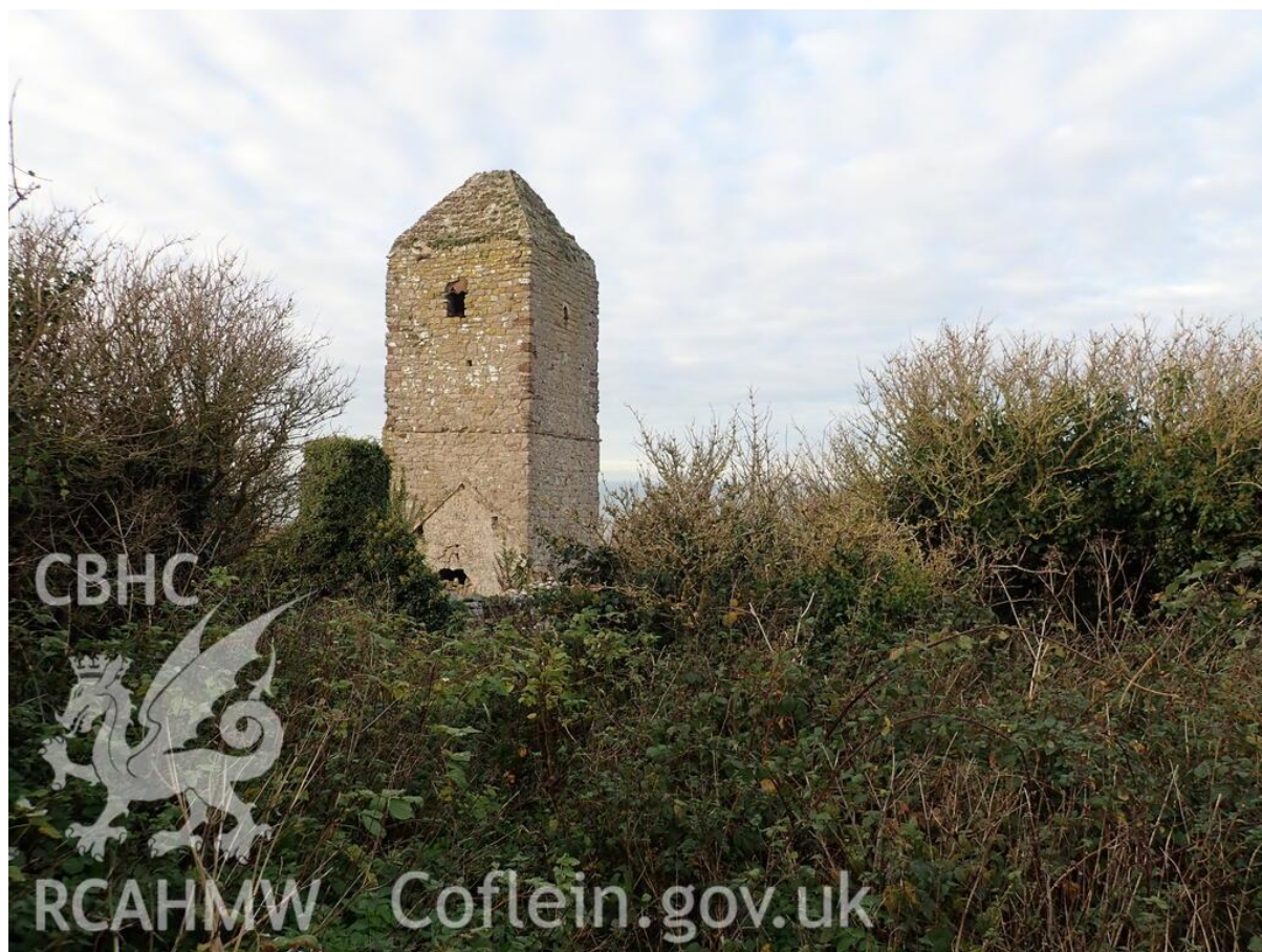
Figure 17 The church tower in November 2018 rising above the local vegetation. (© CHERISH Project. Archive no. 6522905)
