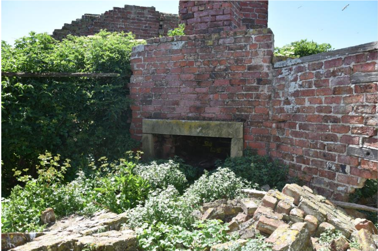
Figure 22 The Telegraph Station: interior view of ruin, June 2018, showing vegetation and elder/buddleia taking hold, and collapsed brickwork (© CHERISH Project: CH2019_098_002)
